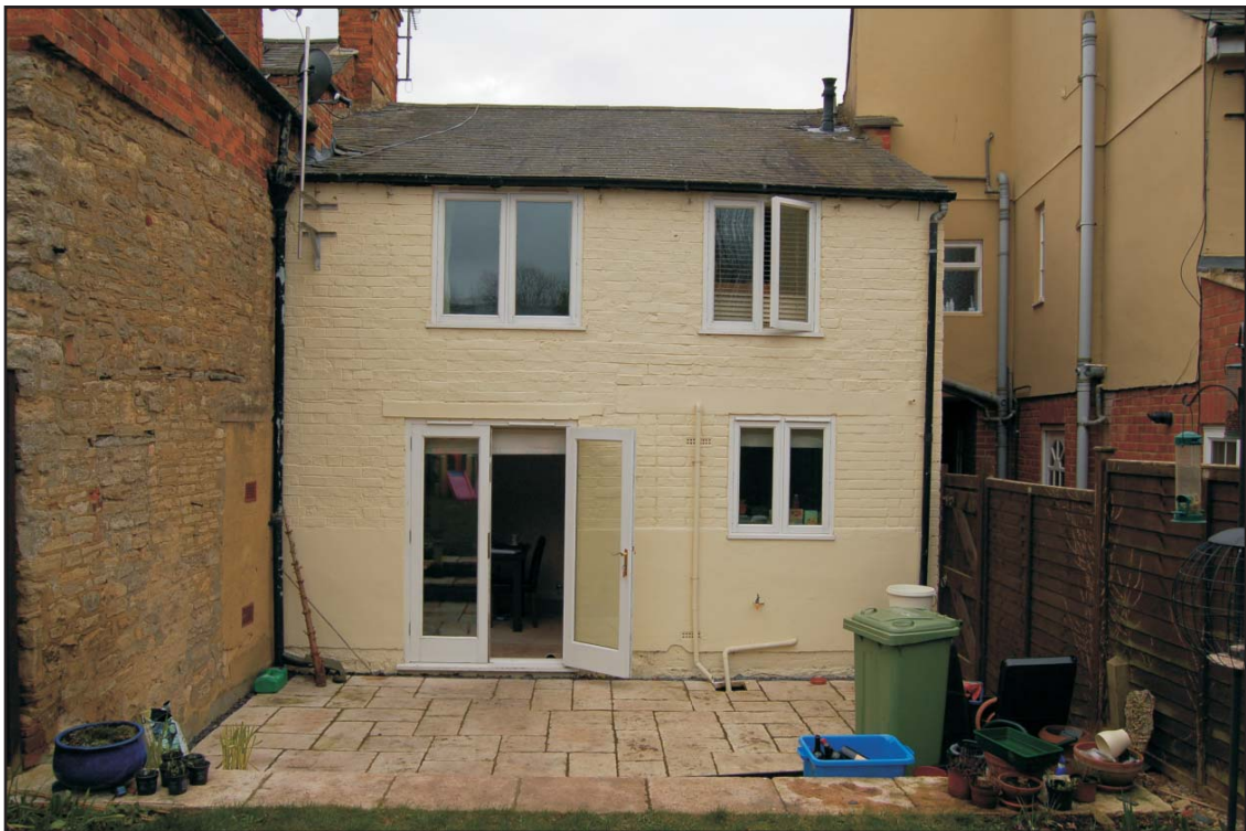
The west elevation, looking east Plate 2
