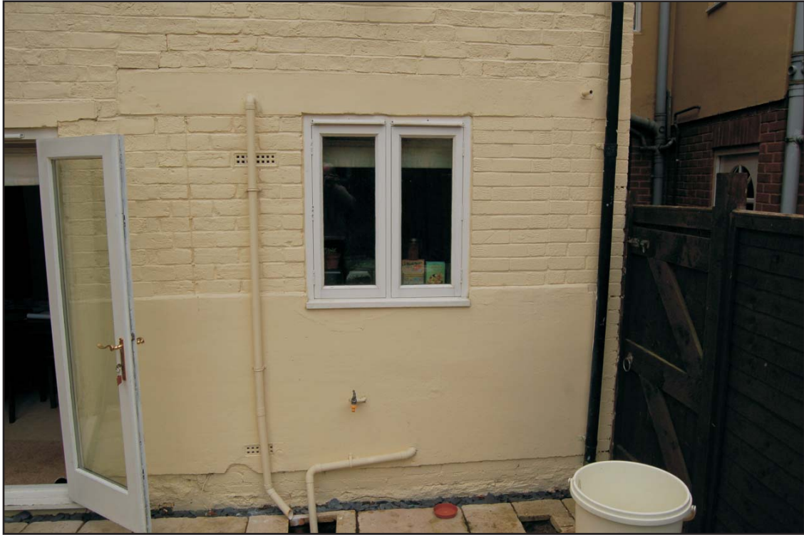
The kitchen window showing evidence for earlier, wider, opening Plate 3
