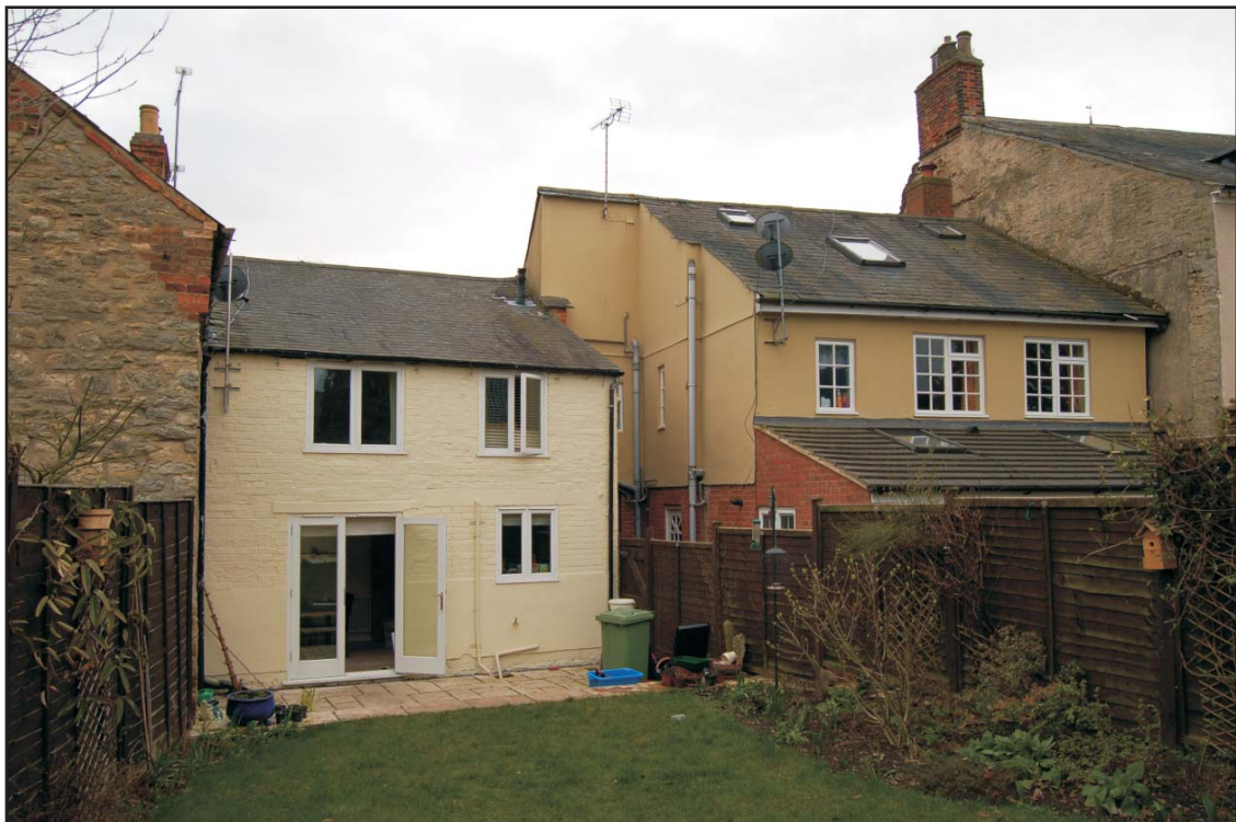
The rear elevation of number 13 and adjoining properties, looking south-east Plate 7
