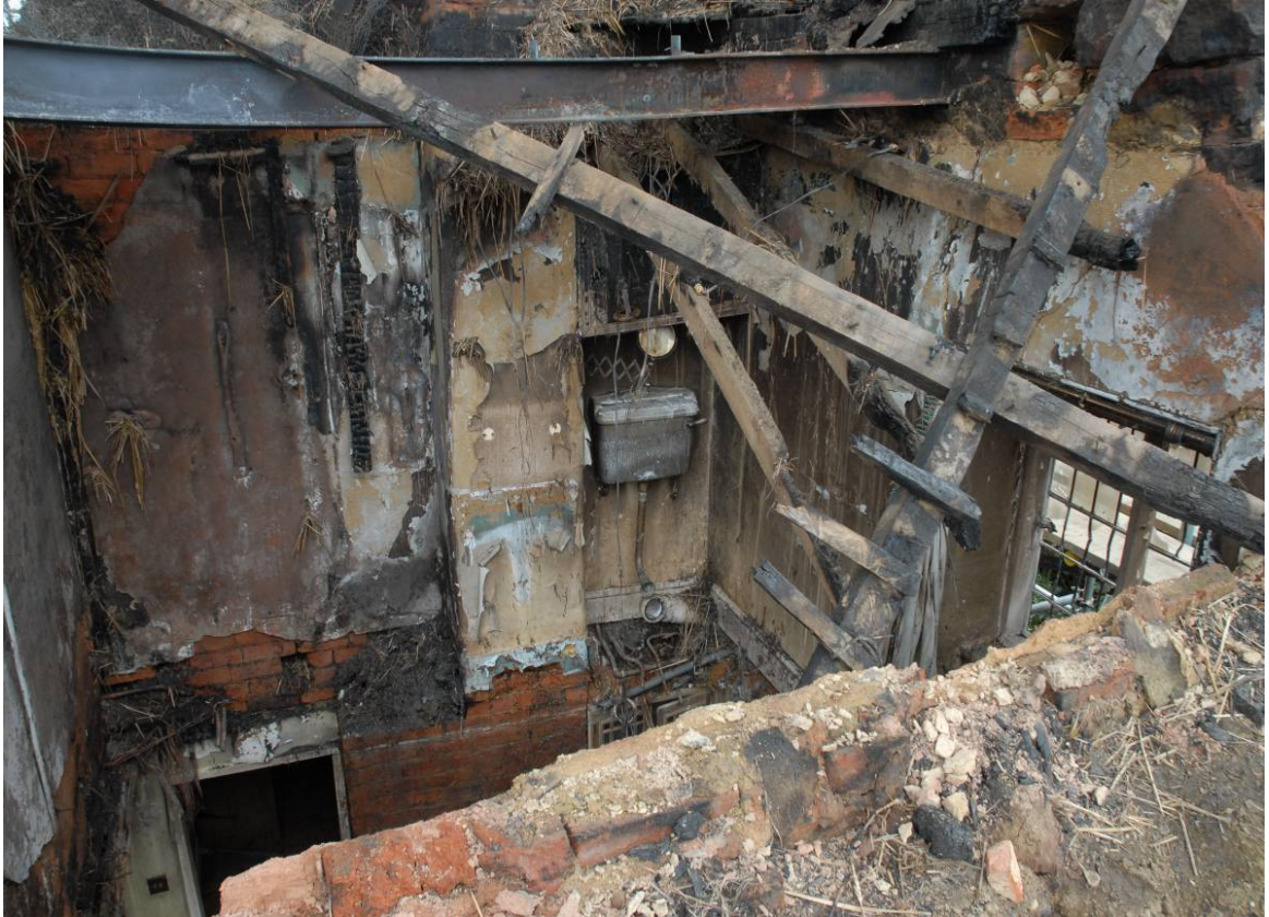
The en-suite bathroom, looking south-west Fig 29
