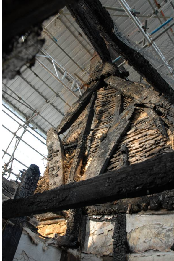
Cruck, yoke and braces, looking north-east Fig 25
