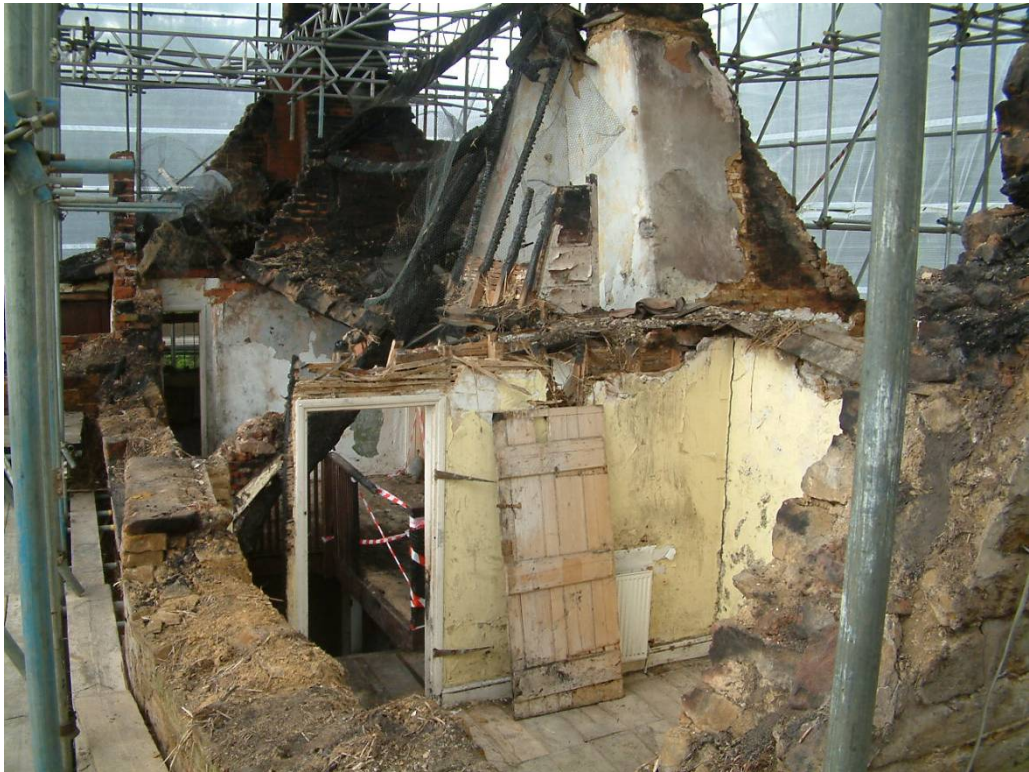
First floor, looking west Fig 8
