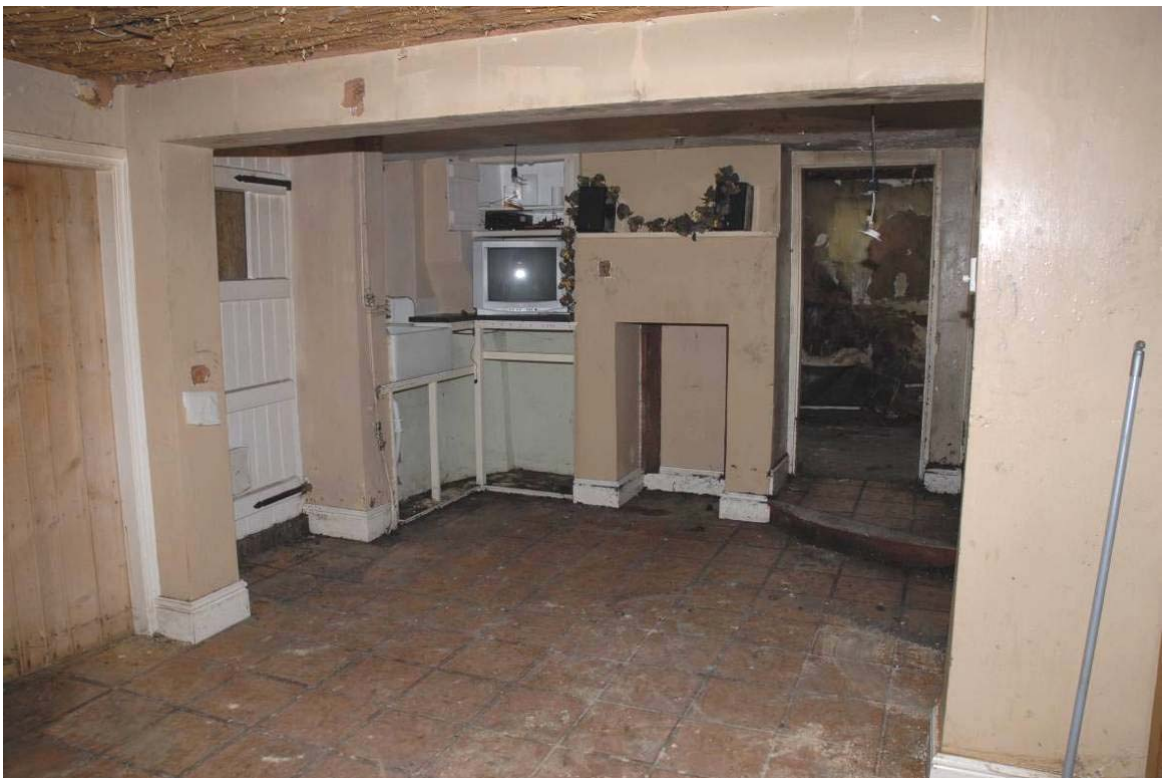
Kitchen, looking north-west Fig 21
