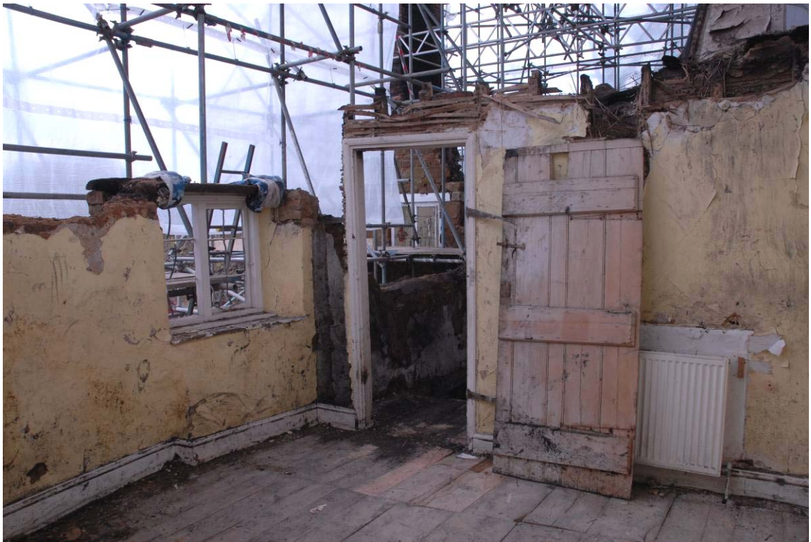
Bedroom 4, looking south-west Fig 33
