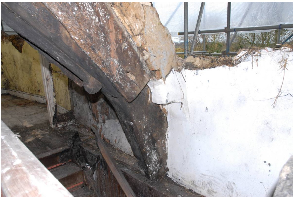
Cruck, looking south-east Fig 22
