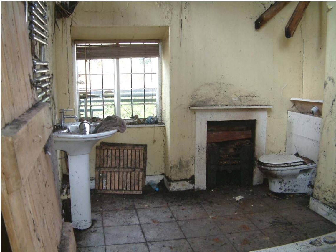
Bathroom, looking west Fig 30
