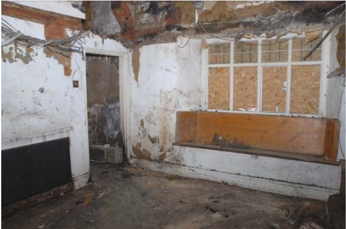
Lounge, looking north-west Fig 17
