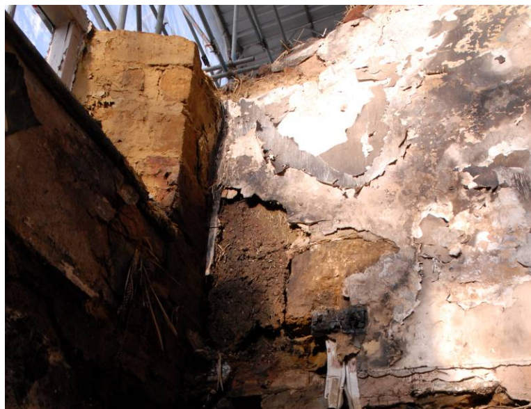
Cob fill, looking east Fig 26
