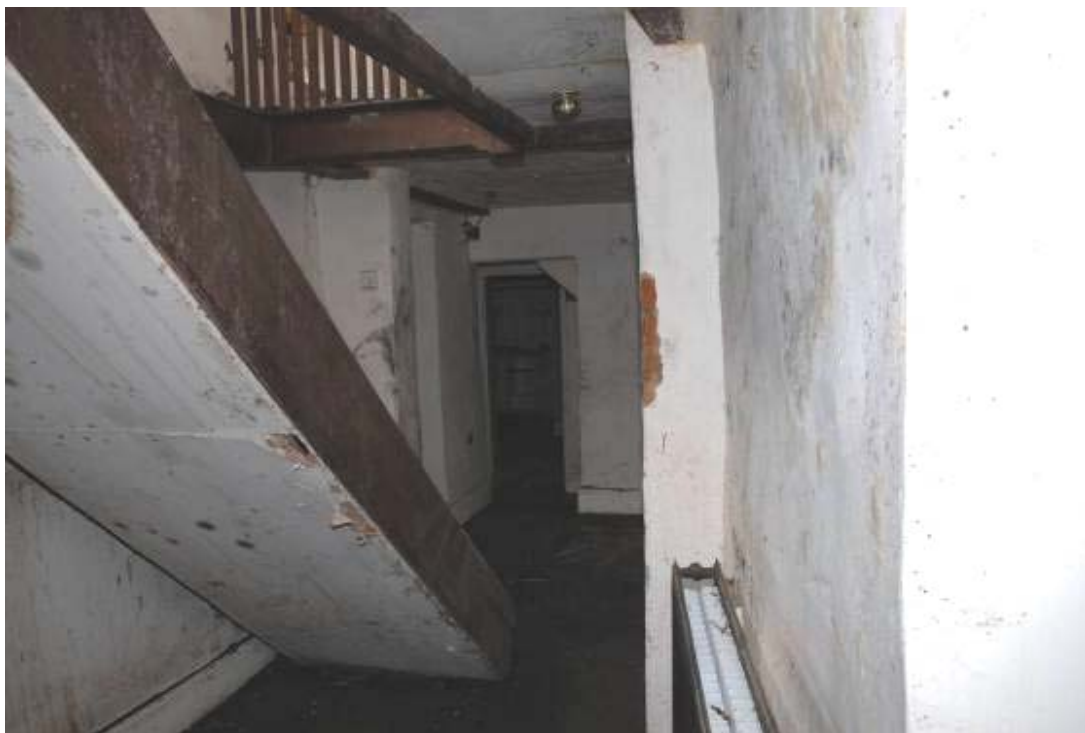
Hallway, looking west Fig 11
