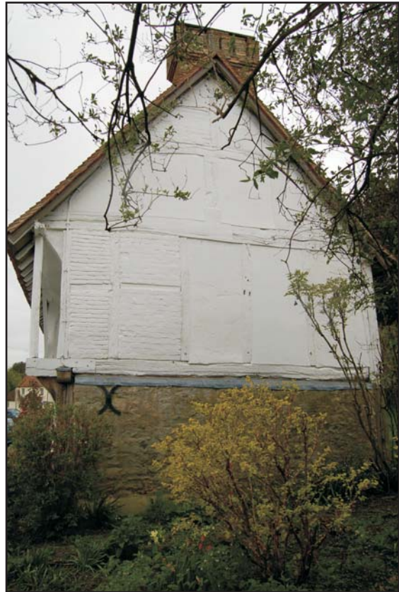
The East gable, looking west Plate 5
