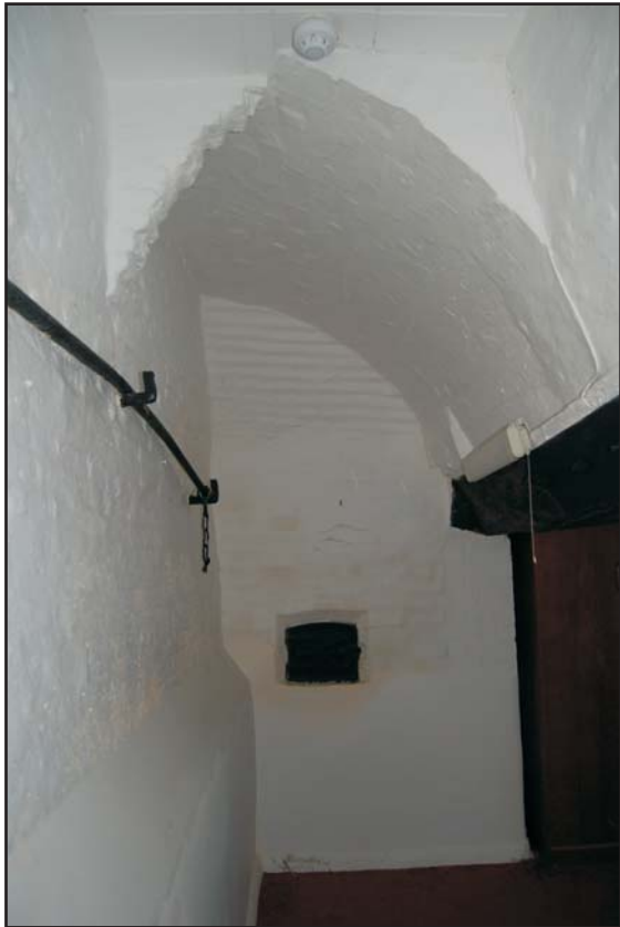
Inglenook, looking south, showing the brick springing supporting the fireplace above Plate 16
