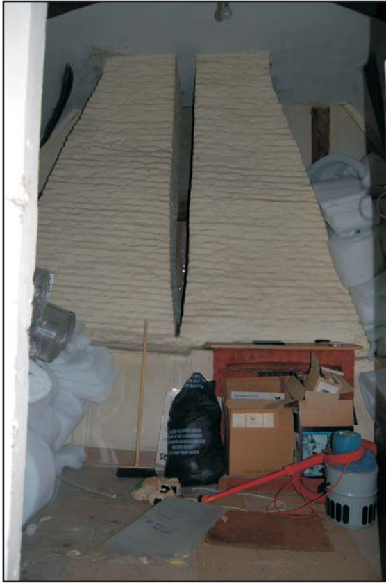
Room 9, the chimney flues and fireplace, looking east Plate 18
