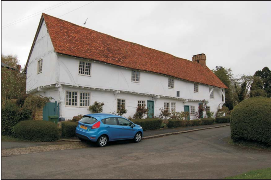
Long Crendon Courthouse, looking north-east Plate 1
