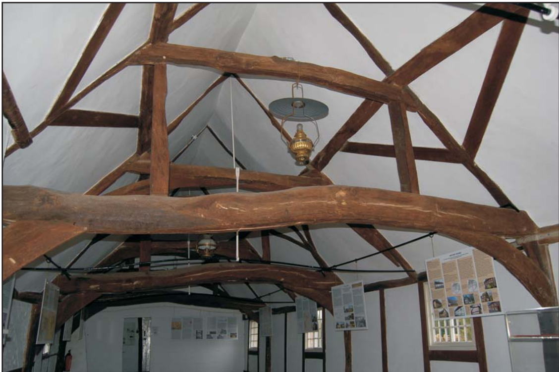
Queen post truss, looking east Plate 20
