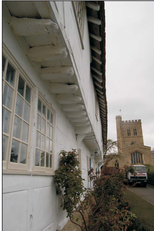
The jetty with principal transverse beams and joists, looking east Plate 2
