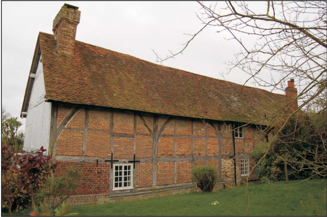
The north elevation, looking south-west Plate 6
