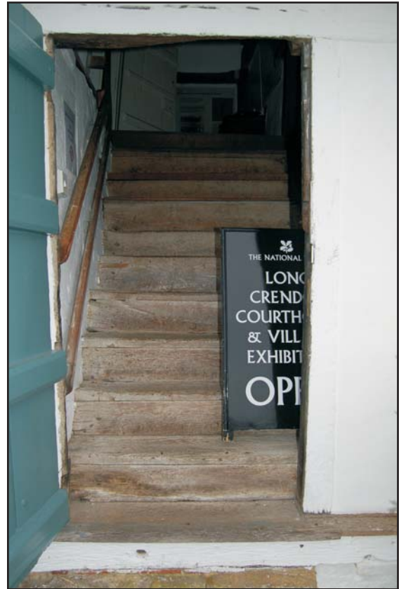
Stairs to the first floor, looking north Plate 17
