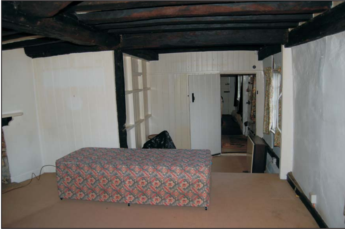
Room 1, looking east Plate 8
