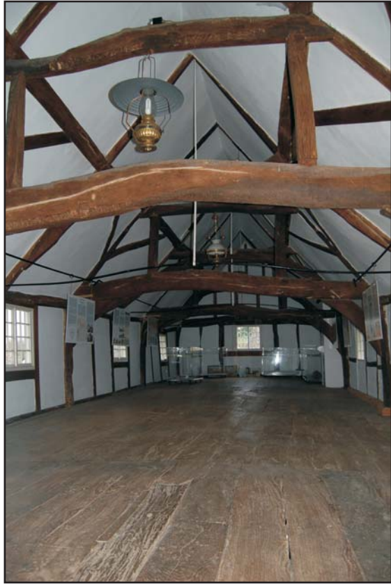
Room 10, looking west Plate 19
