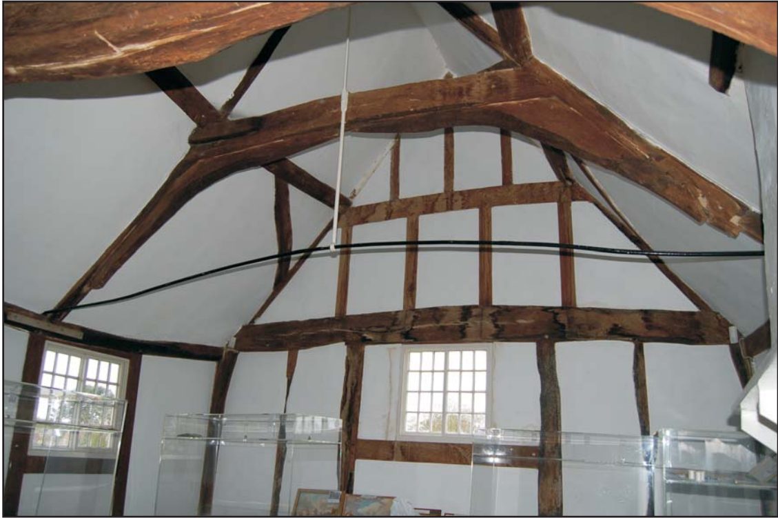
Braced truss, looking west Plate 21
