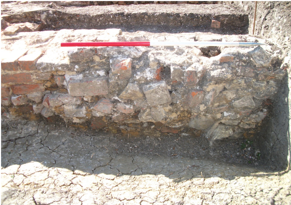
The possible repair to wall (109), looking south-east Fig 8
