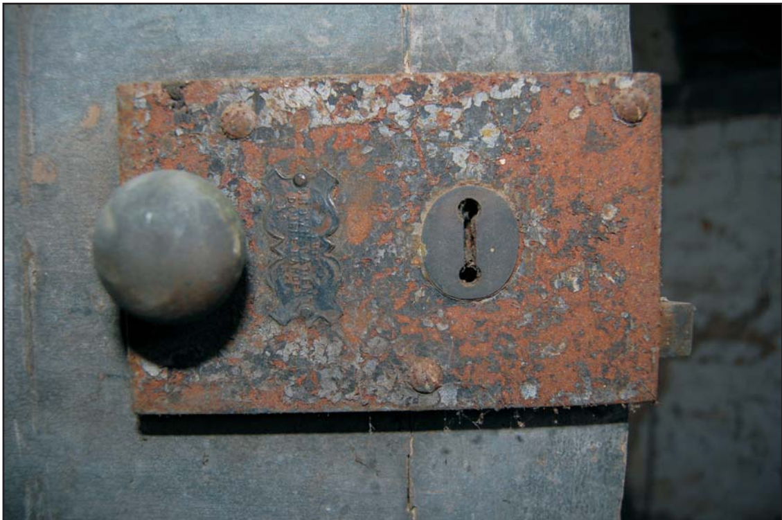
Rim lock on the west side of the door between the two rooms at first floor level, looking east
