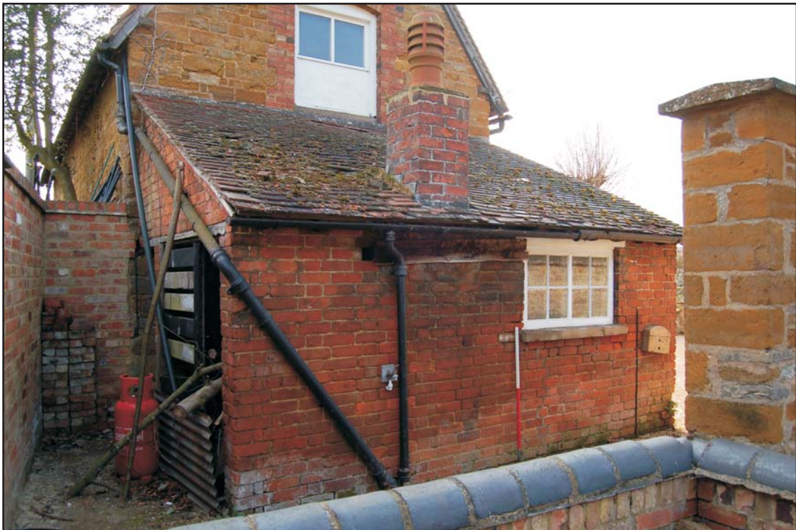
The west elevation with later tack room, looking south-east Plate 4
