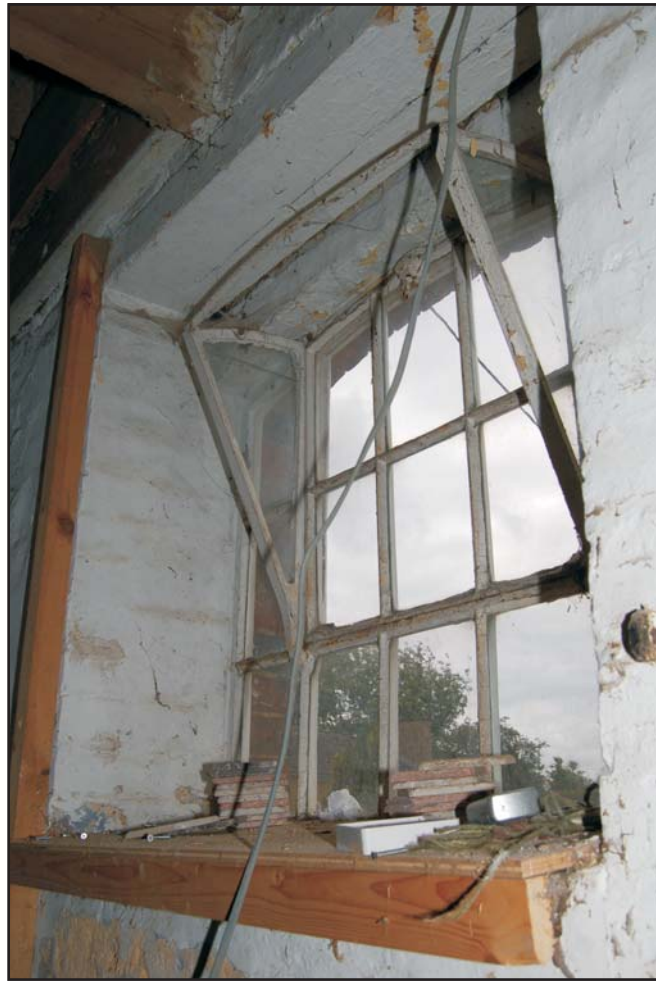
The eastern cast iron stable window, looking south-east Plate 11
