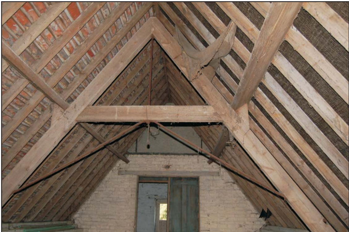
The first floor, looking west Plate 12
