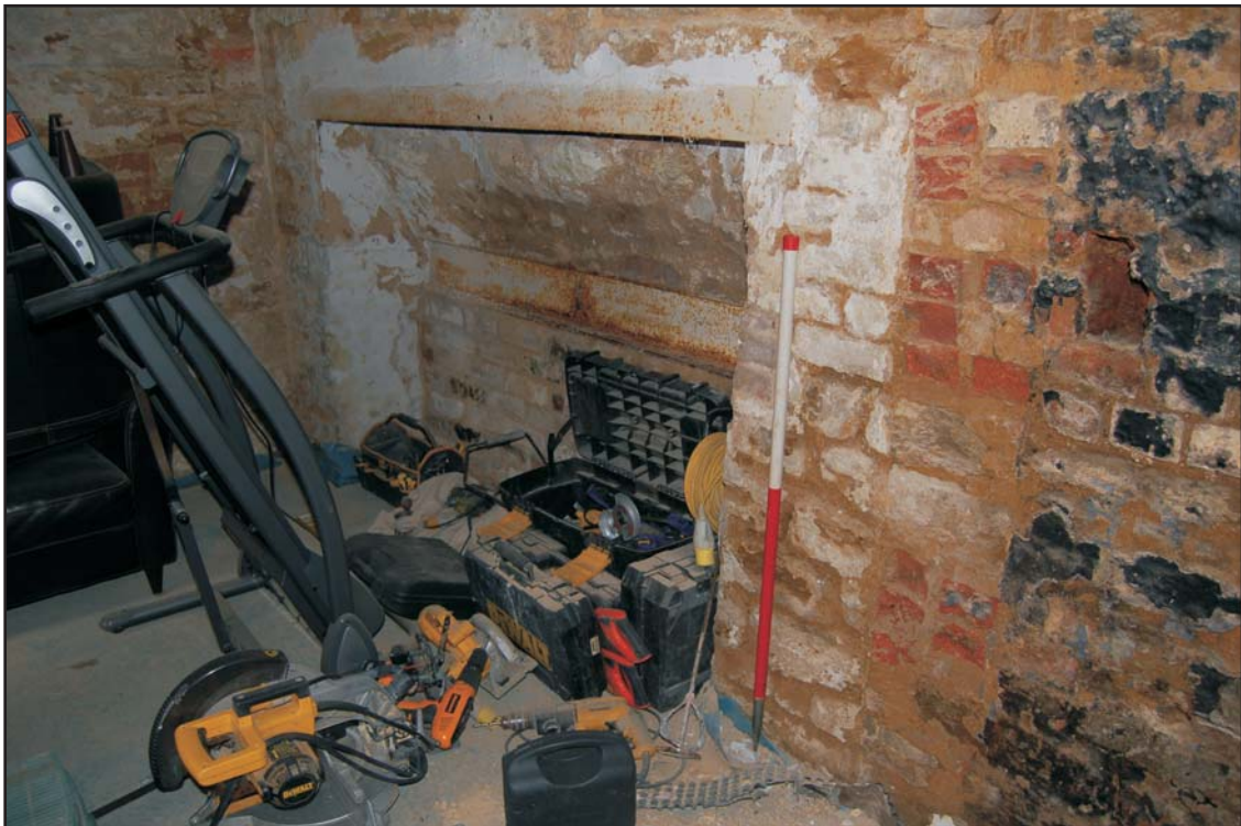
Recess in the north wall of carriage house, looking north-west Plate 6
