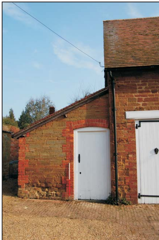
The tack room, looking north Plate 18
