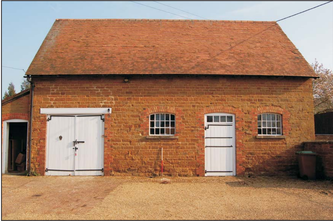
The south elevation of the stable block, looking north Plate 1
