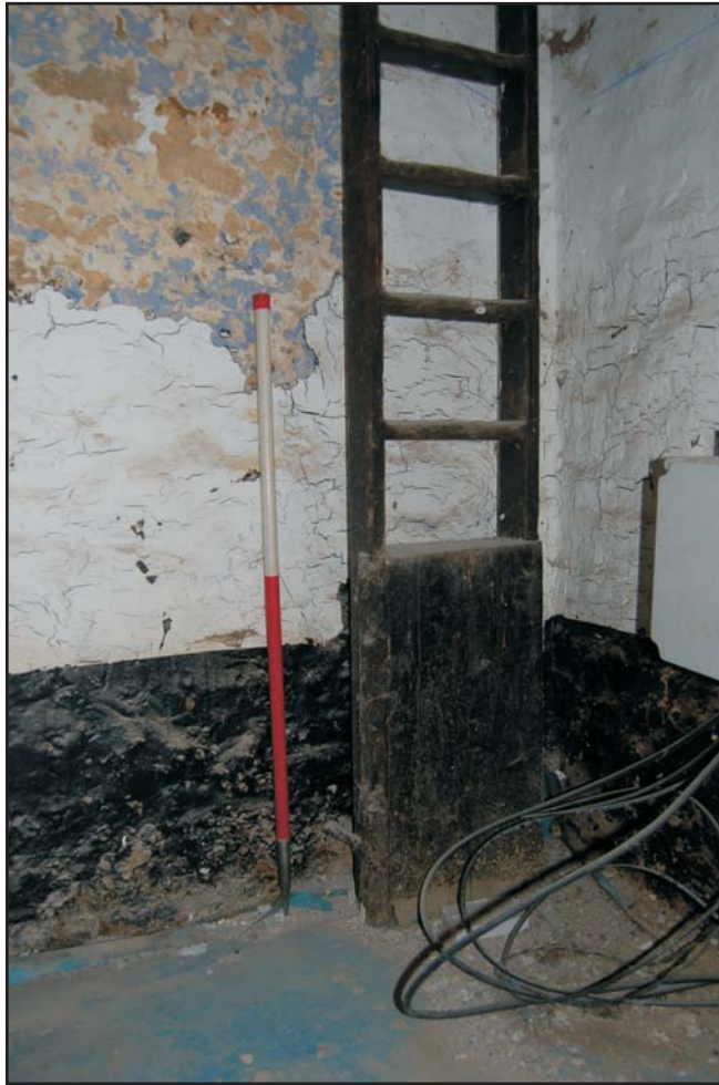
Loft ladder to the first floor, looking south-east Plate 7
