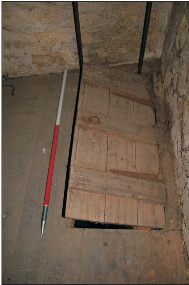
The loft ladder trap door, looking east Plate 13
