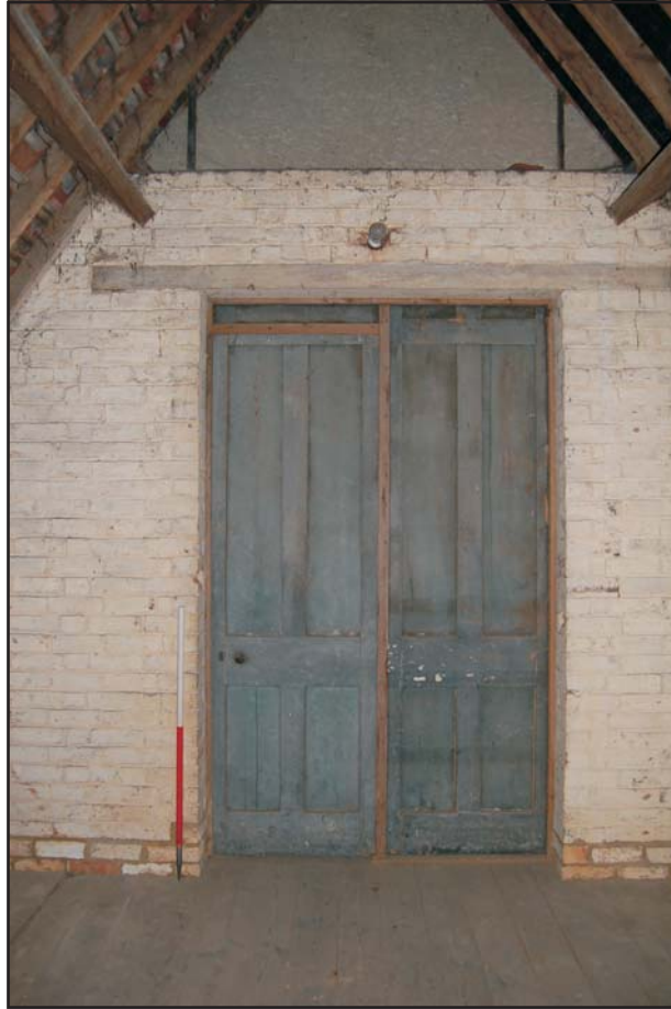
The dividing wall at first floor level, looking west Plate 15
