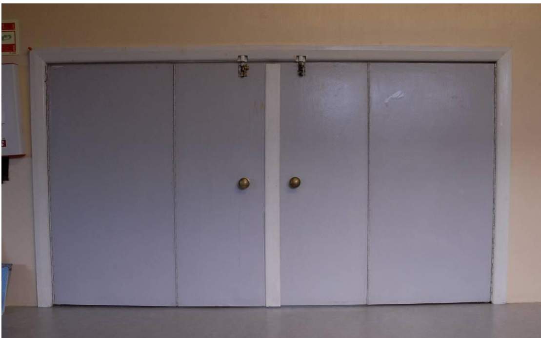
The serving hatch between the Hall and Kitchen Fig 12
