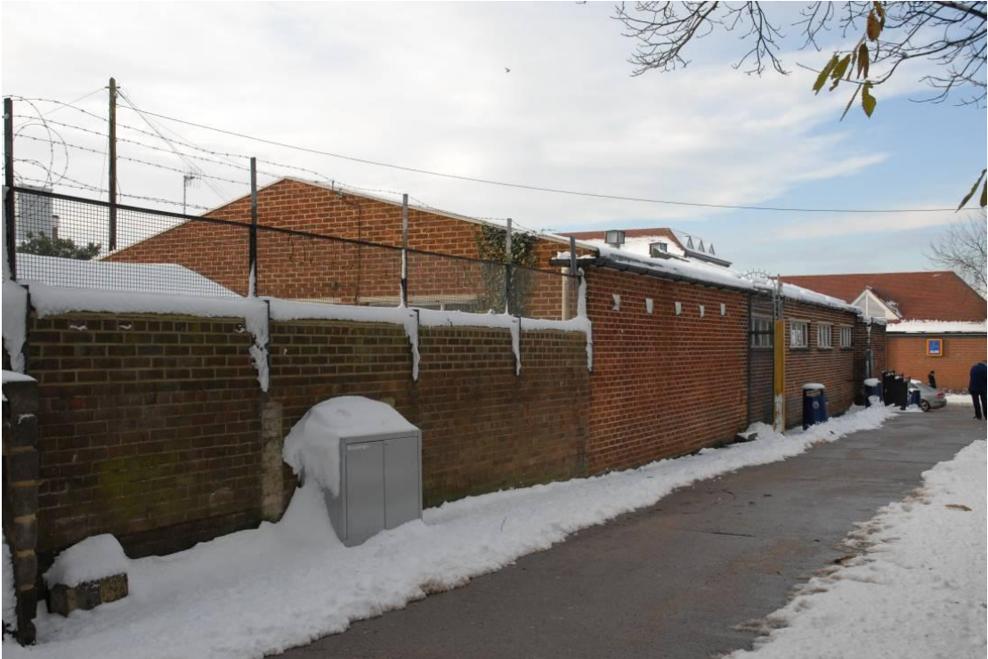
The north-east elevation showing a rear extension of the 1955 building Fig 5
