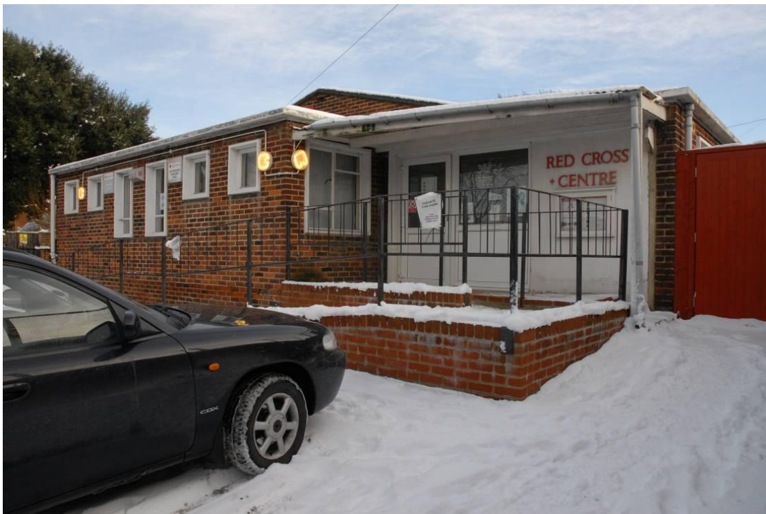
The front elevation of the building, looking east, showing the extensions Fig 4
