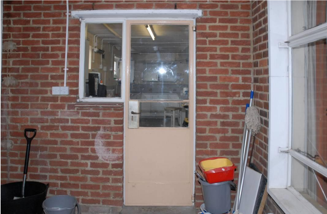
The external door to the kitchen Fig 9
