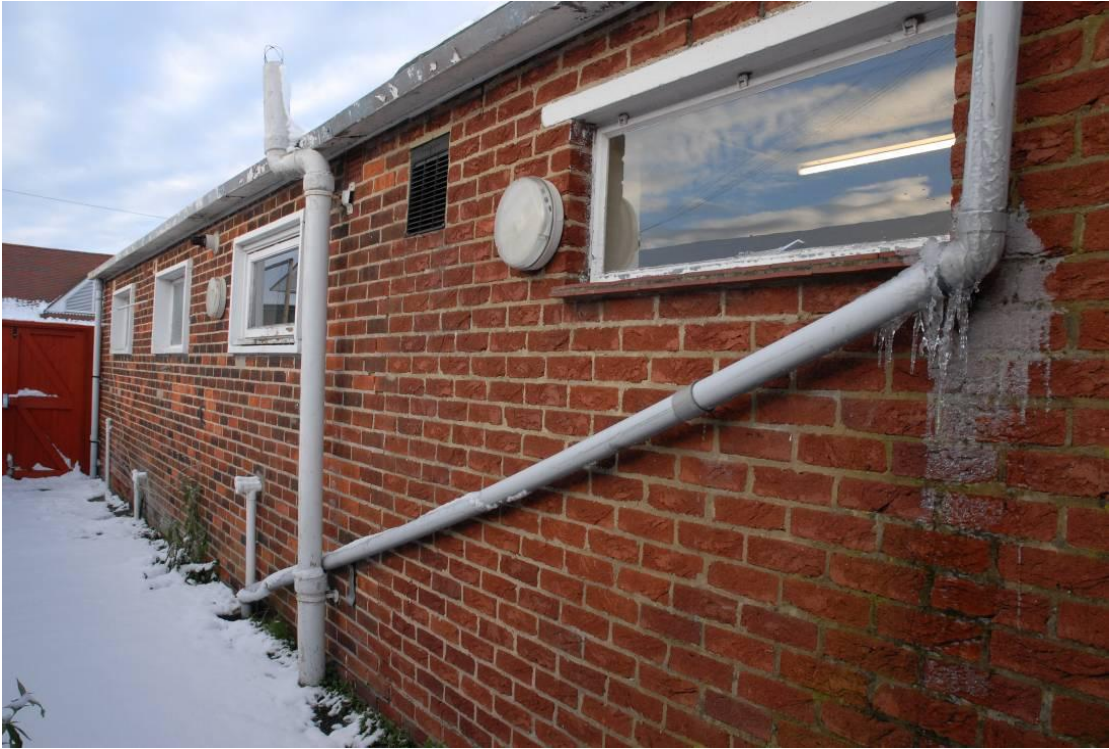
The kitchen extension showing the change in brickwork and fenestration Fig 7
