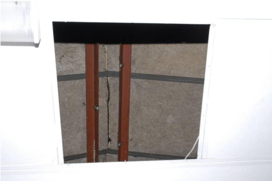
The roof frame visible through the ceiling Fig 10
