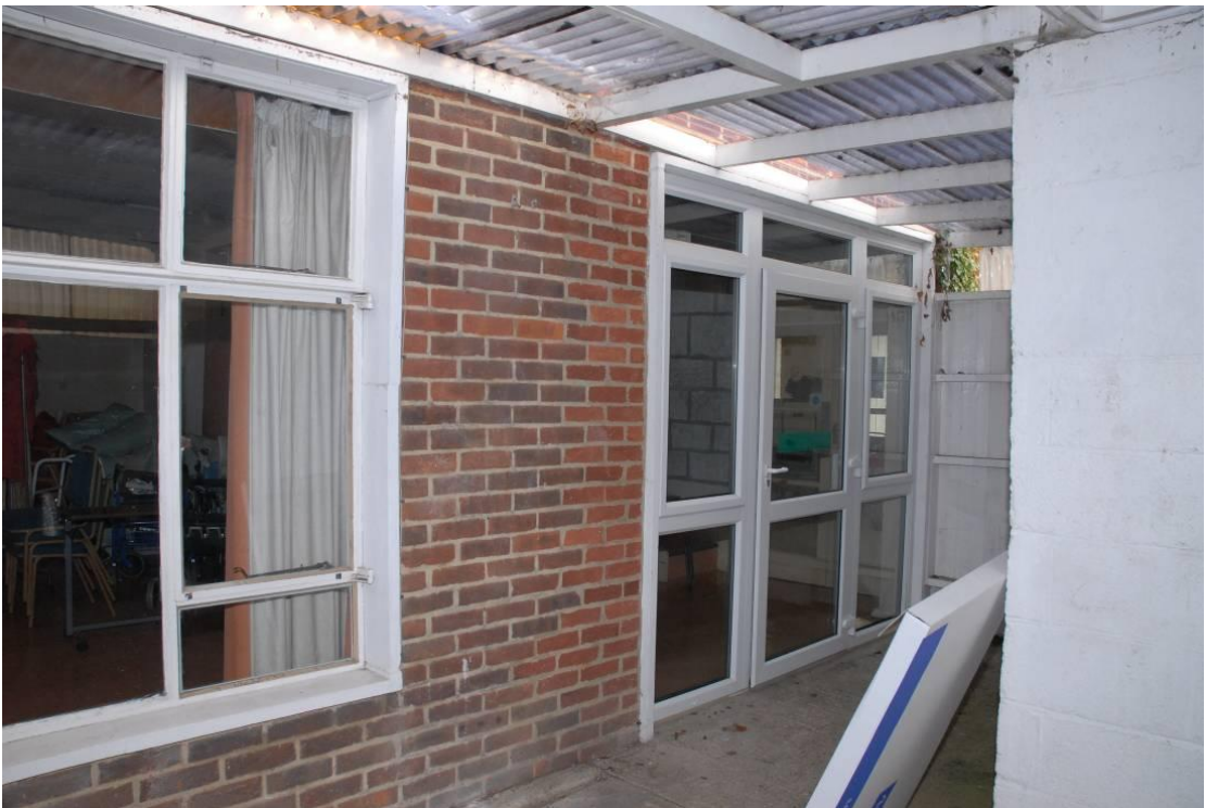
The south doorway showing the change in brickwork Fig 6
