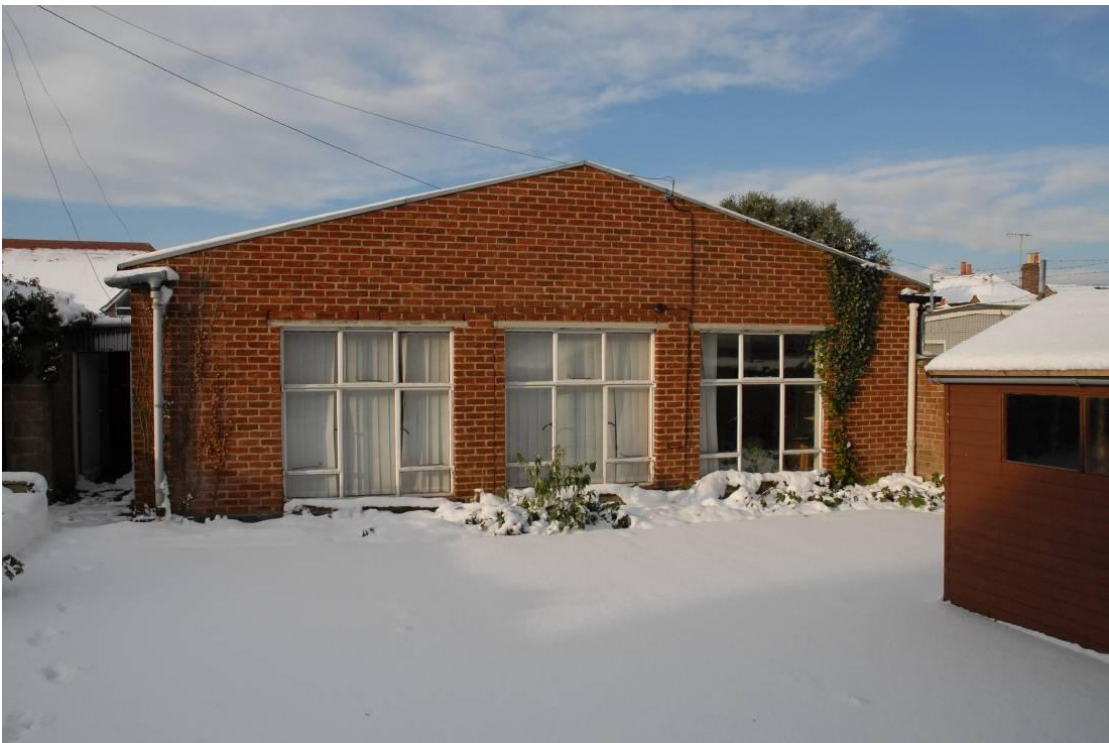
The rear elevation showing window and lintel styles Fig 8
