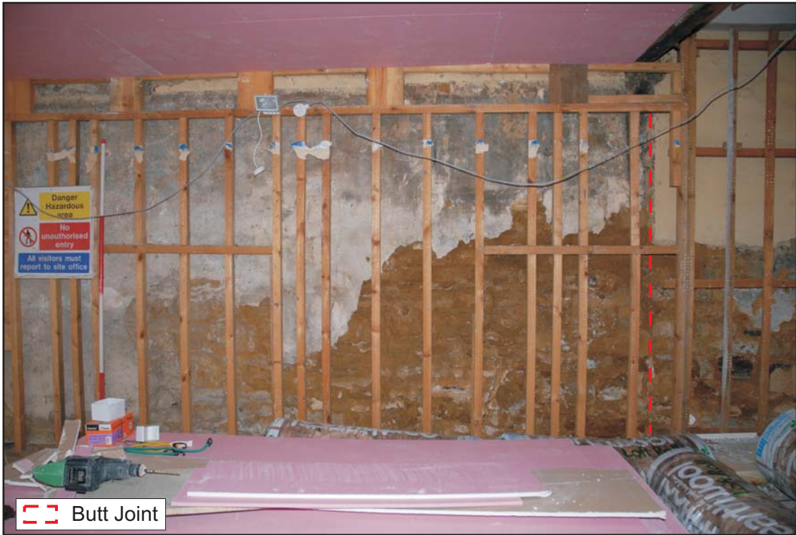
View of plain east wall, interior face. (Butt joint to the right) Fig 6
