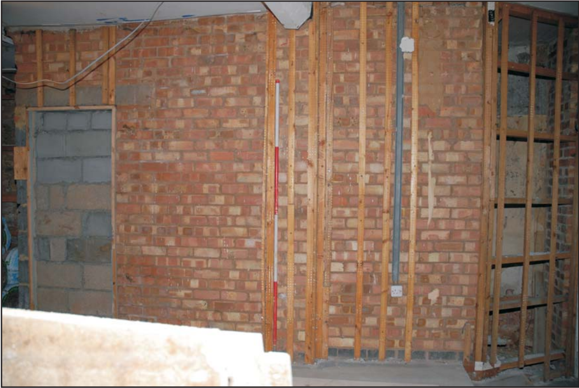
View of former stairwell in west wall Fig 4
