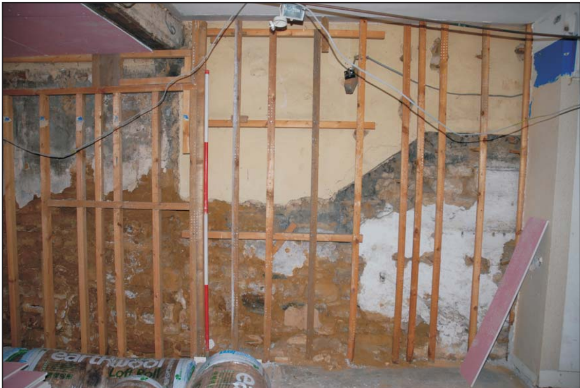
View of former stair location Fig 7
