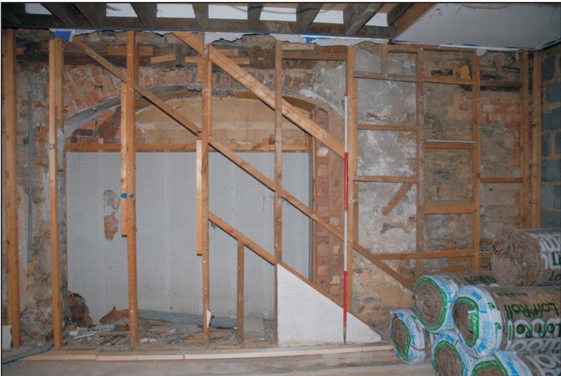
View of blocked doorway in west wall Fig 5
