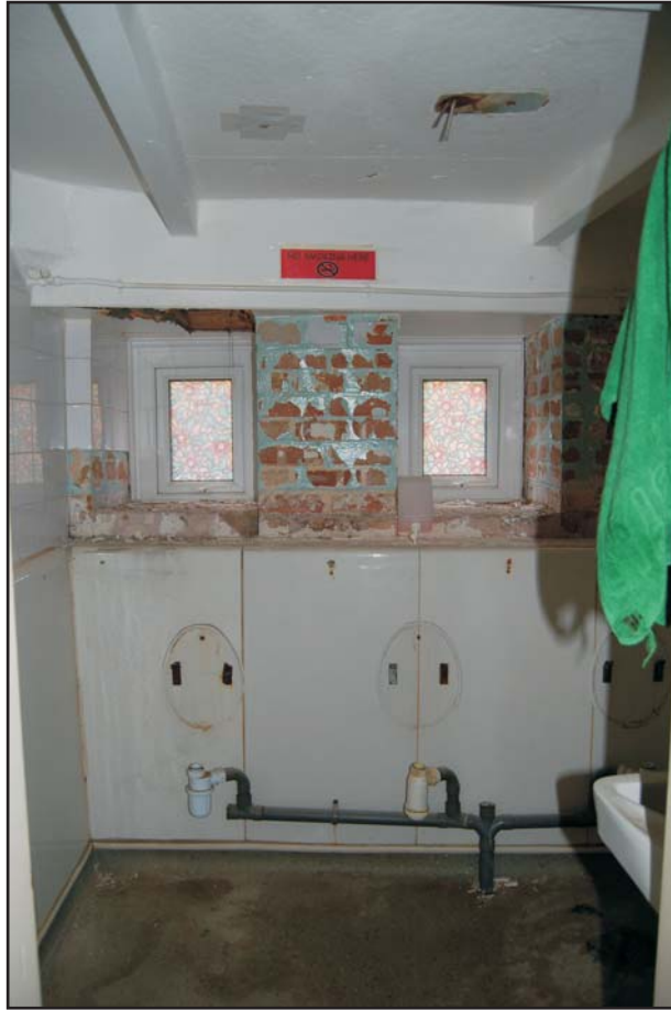
Room G4, showing urinals, looking south Plate 5
