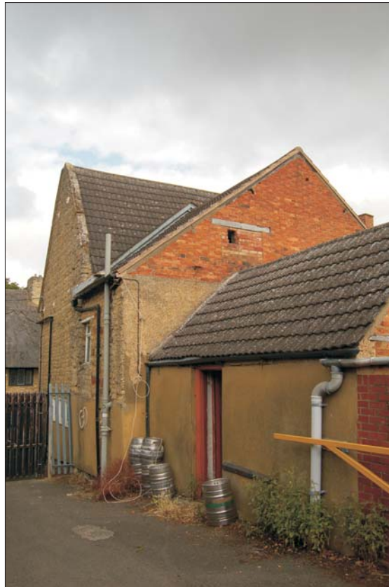
Room F4, east elevation, looking north-west
