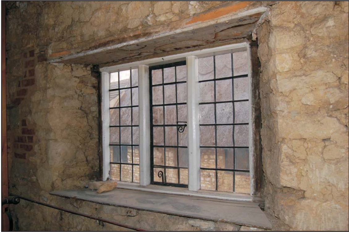
Room F,1 showing window in the west wall, looking west Plate 11
