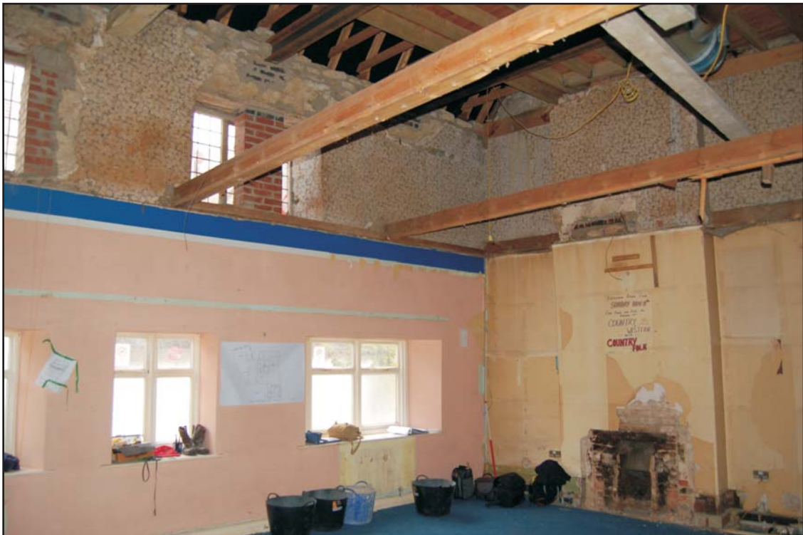
Room G5, looking north-west Plate 6
