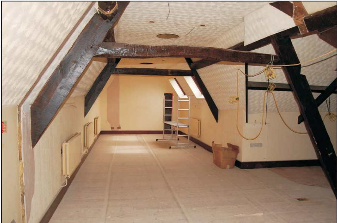
Room S1, looking north showing original roof trusses Plate 12
