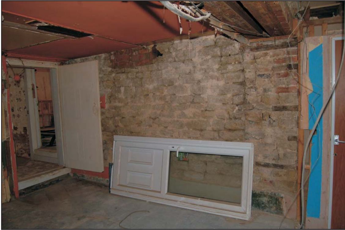
Room G12, north (original external) elevation of stone addition, looking south, showing butt joint with east face of the stone house
