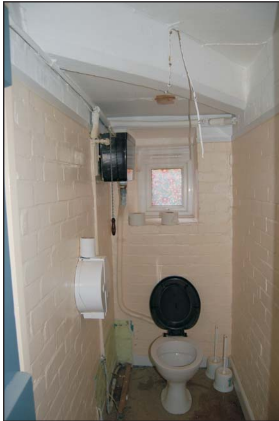
Room G3 showing diagonal beam in ceiling, looking south Plate 4
