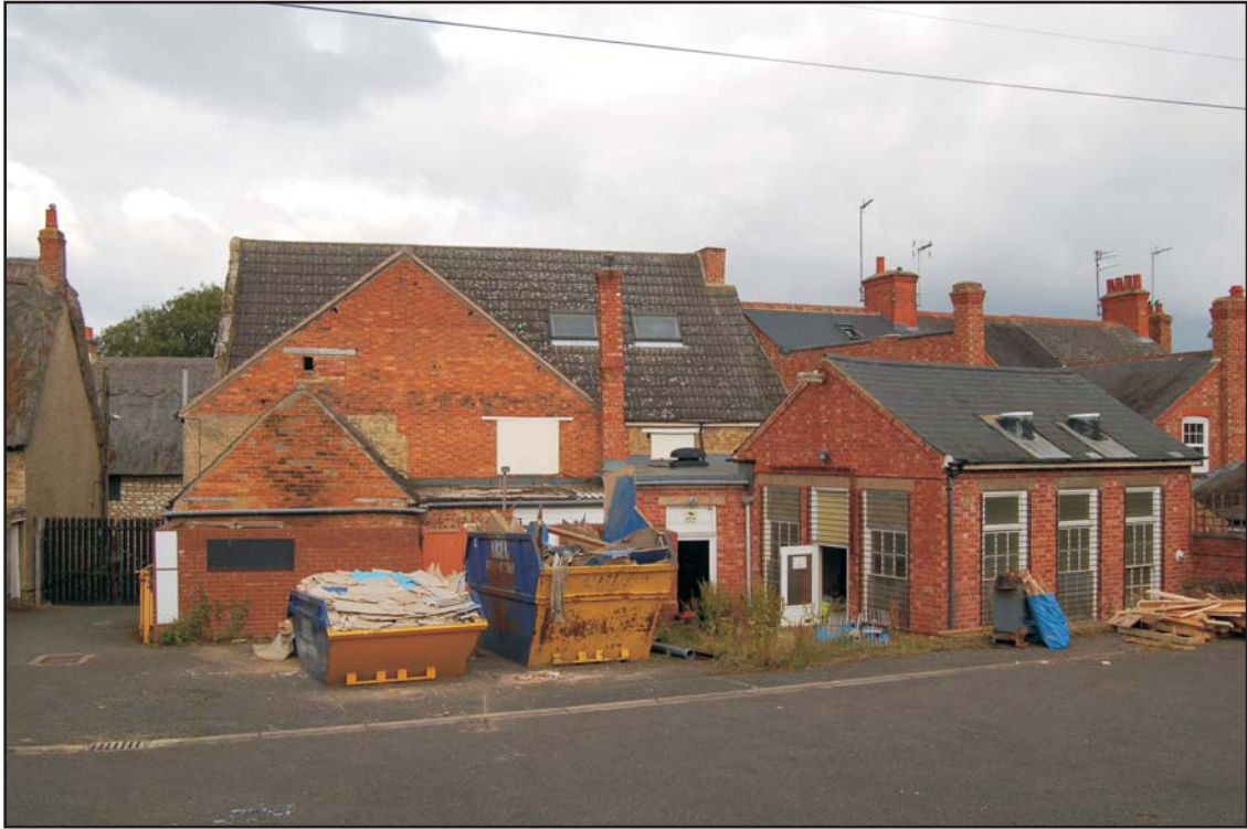
East elevation, looking west Plate 3
