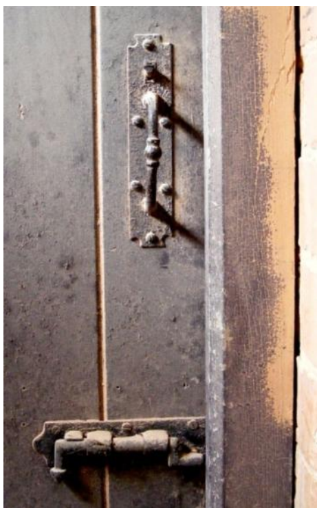
The decorative latch lifter and bolt on the carriage house door Fig 30
