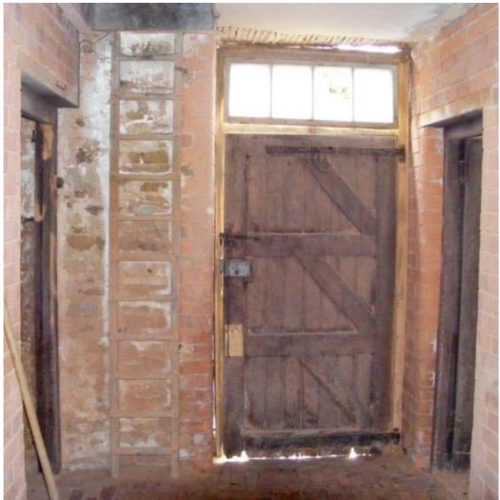
Stable 1, the front door and hayloft ladder Fig 35
