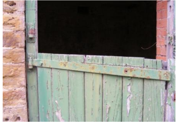
Lower door and strap hinge, Stable 3 Fig 14
