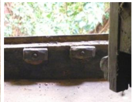
Simple shutter catches Fig 59
