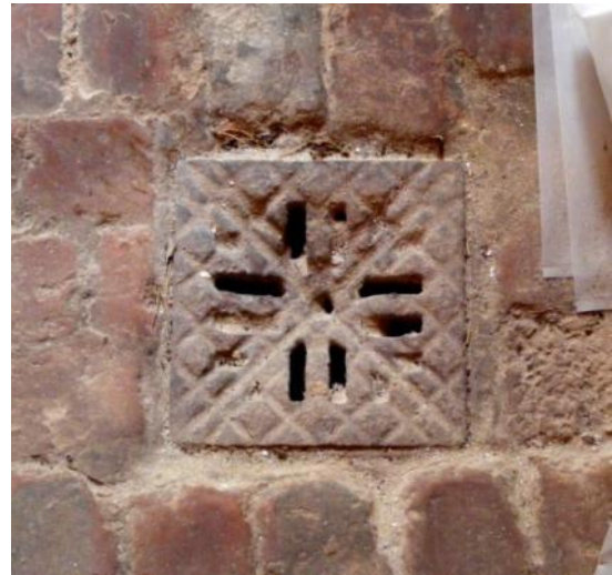
Stable 1, brick floor with central drain Fig 32 Stable 1, the pierced iron grille drain cover Fig 33
