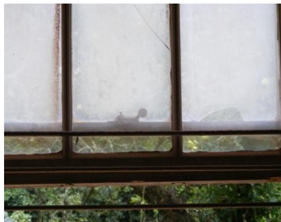
Stable 2, showing metal window catch Fig 44
