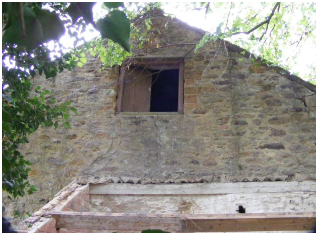
The eastern gable end above the tool shed roof Fig 22
