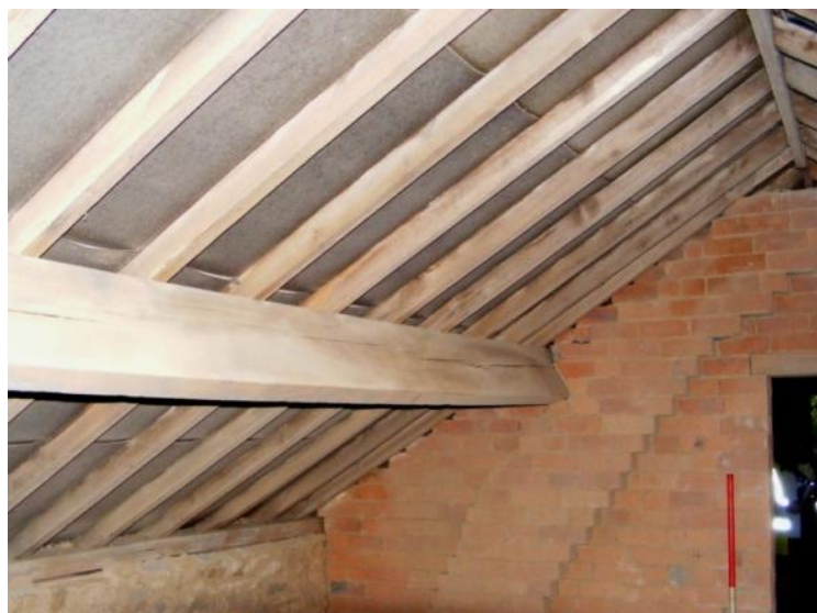
The hayloft, showing wall plate, purlin and rafters, looking east Fig 52
