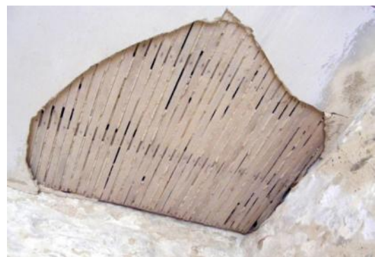
Stable 3, lath and plaster ceiling Fig 49
