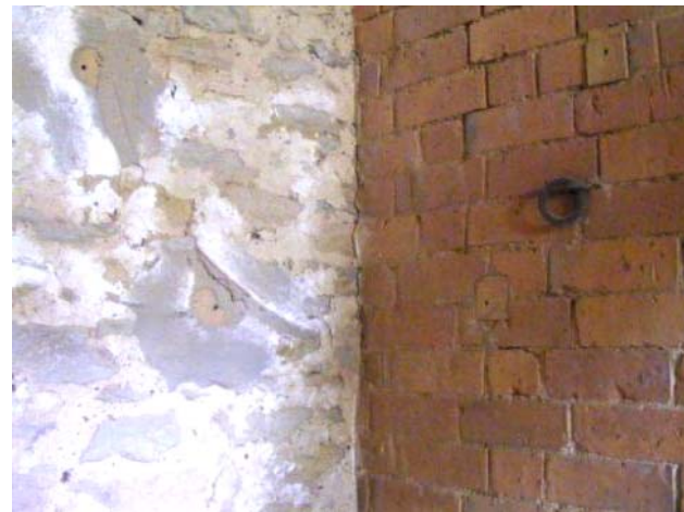
Stable 1, the fittings for a corner manger Fig 37
