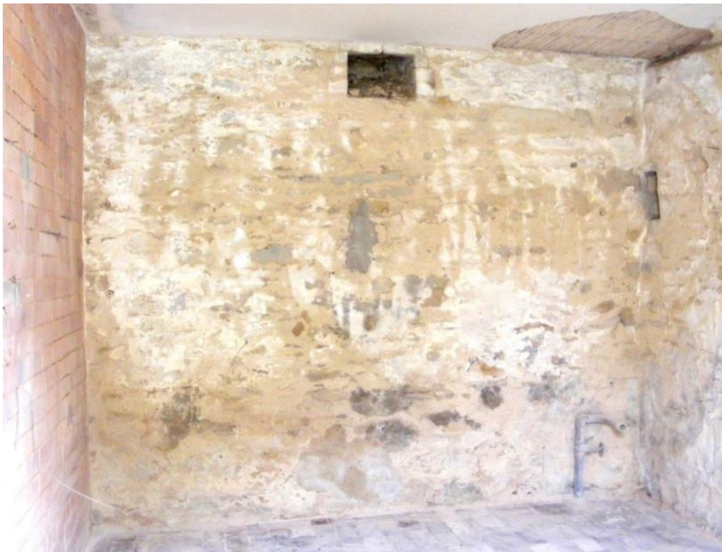
Stable 3, the north wall, with ventilator, slot and water pipe Fig 46
