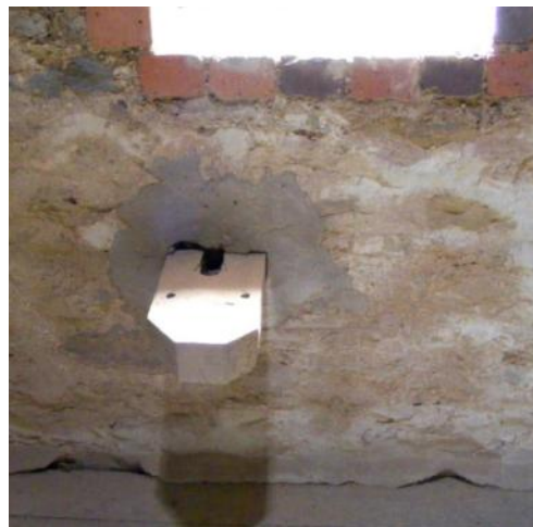
The hayloft, wooden bracket below west window Fig 62
