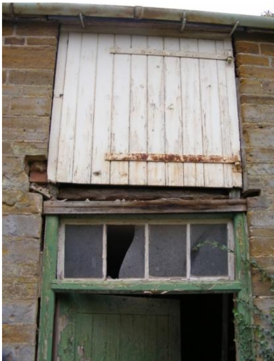
The hayloft door, with strap hinges Fig 11 The carriage house window Fig 12
