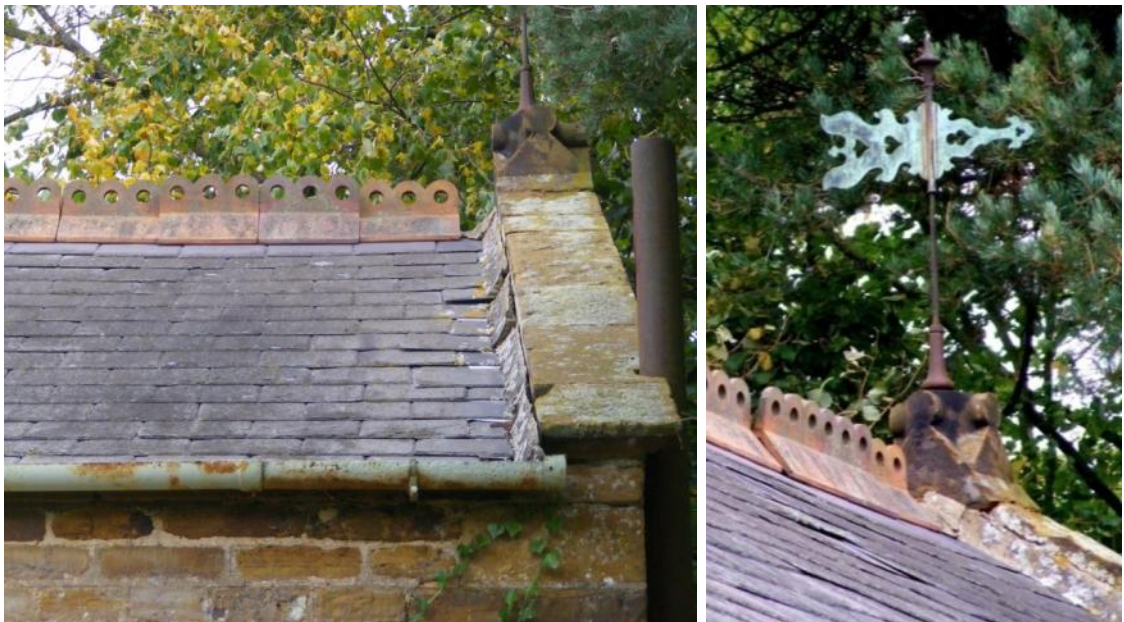
Detail of roof showing the ironstone coping and the decorative ridge tiles (left), and weather vane mounted on a stone finial at the eastern gable (right) Fig 18
