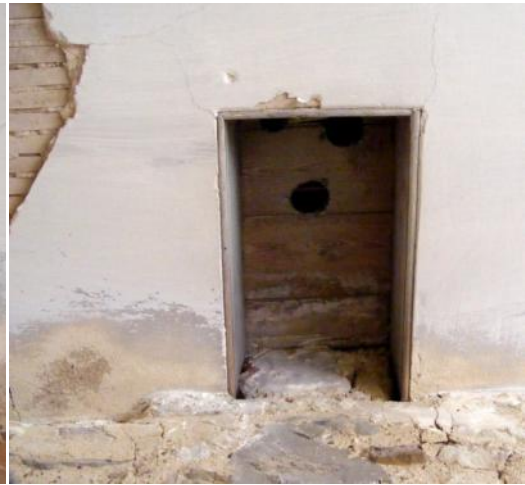
Stable 3, ceiling aperture Fig 51
