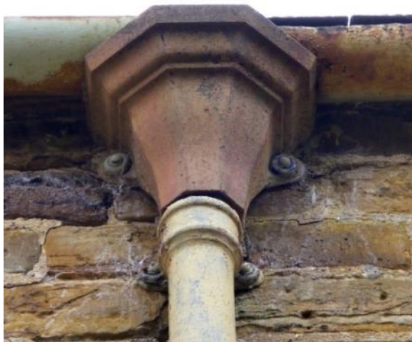
Cast iron rainwater head Fig 15
