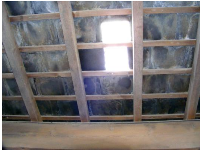
The hayloft, showing laths, Welsh slates and glass 'slate' Fig 53
