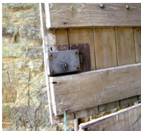
The tool shed, door lock Fig 65
