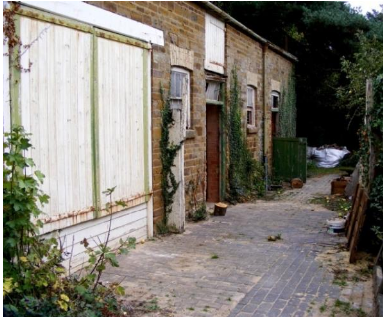
Brick yard along south frontage, looking east Fig 6
