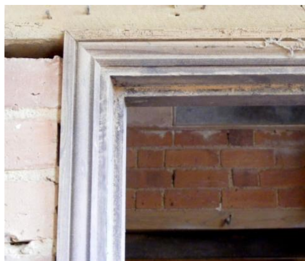
The moulded door frame in the carriage house Fig 31
