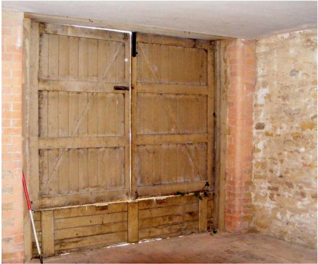
Carriage house doors interior, showing brick jambs Fig 8
