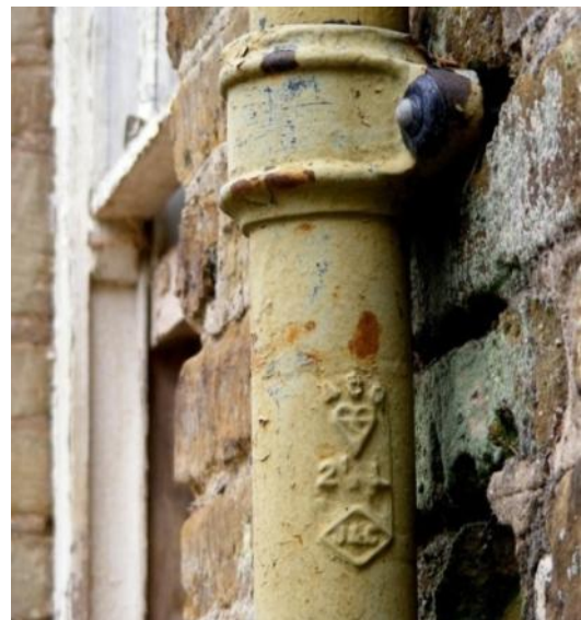
Kite-marked cast iron downpipe Fig 16
