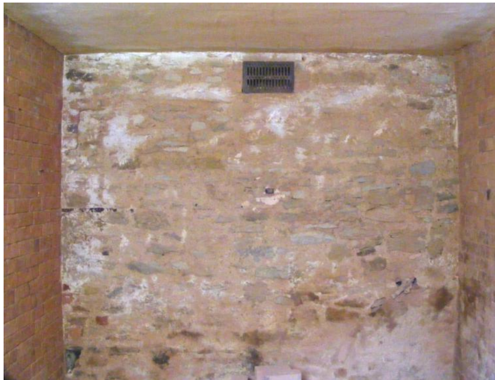
Stable 2, north wall, showing ventilator grille and painted band Fig 41
