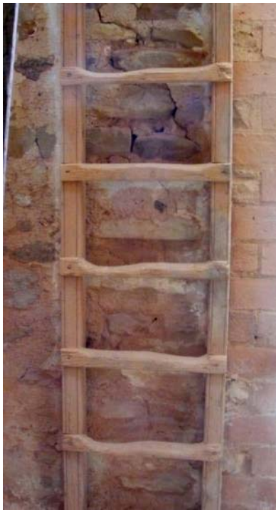
The rungs of the hayloft ladder, showing alternating wear pattern Fig 34
