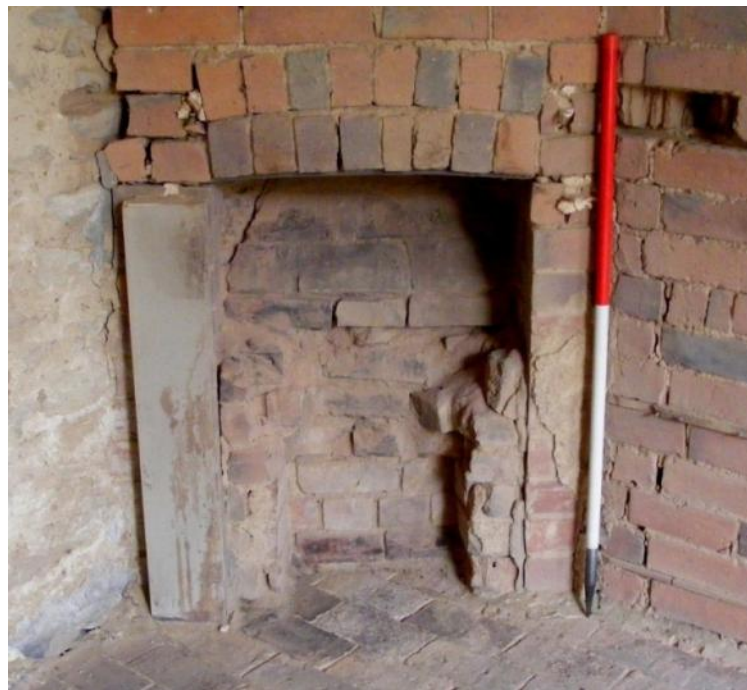
The carriage house fireplace Fig 28
