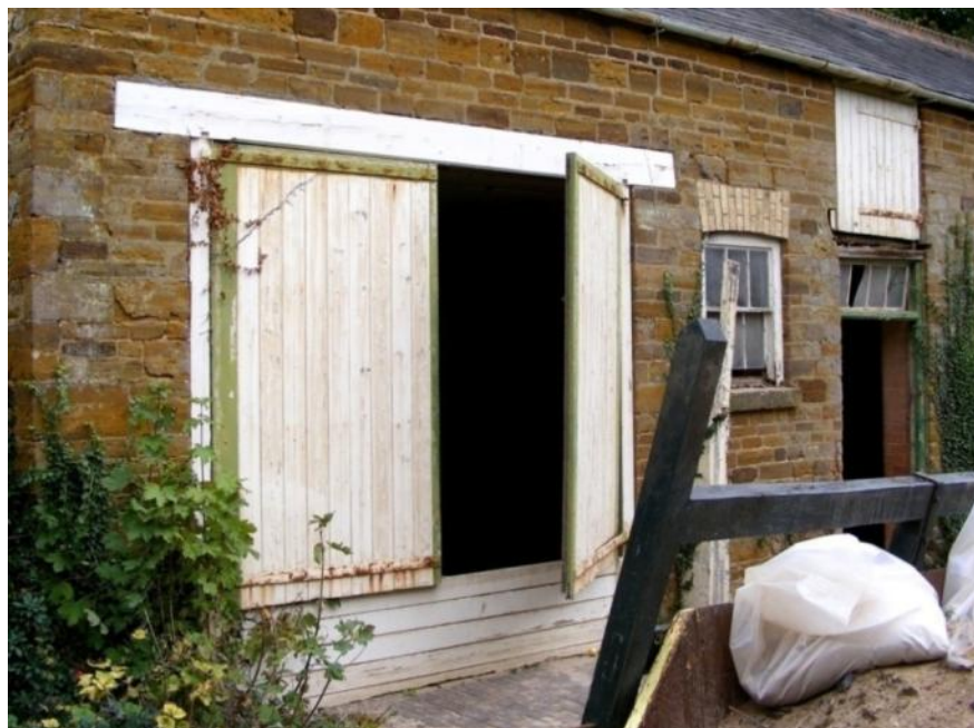
The carriage house doors, looking north-east
