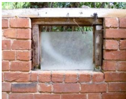
The tool shed window Fig 66
