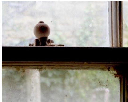
Decorative window catch Fig 26
