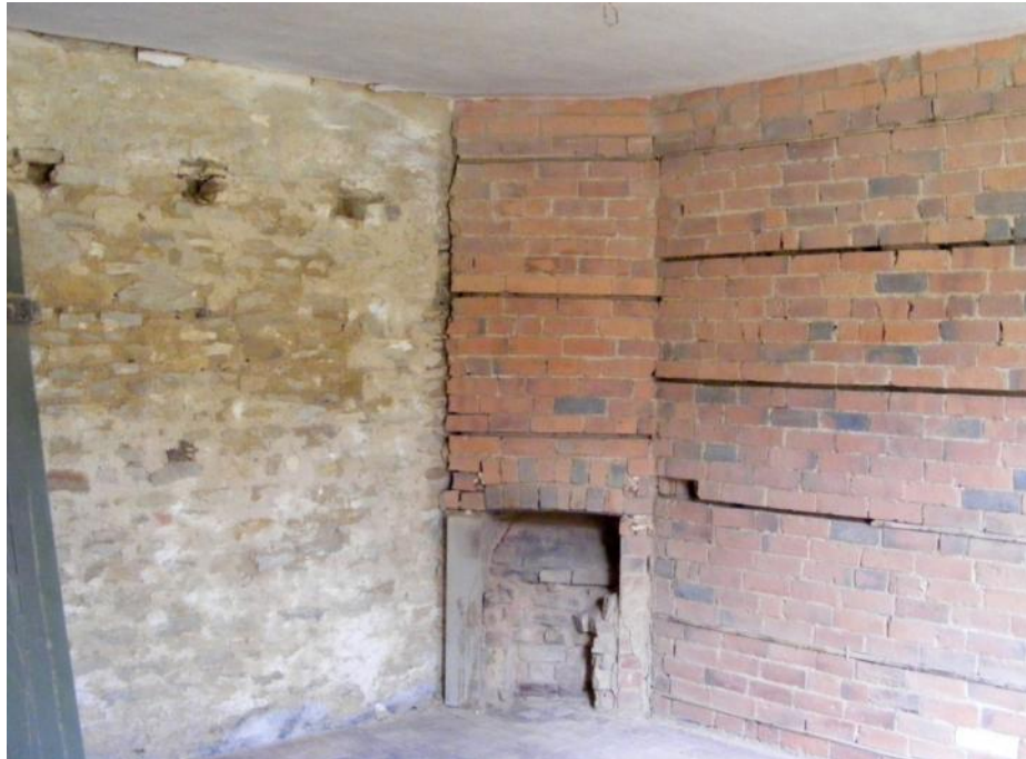
The carriage house, showing corner brick fireplace Fig 27
