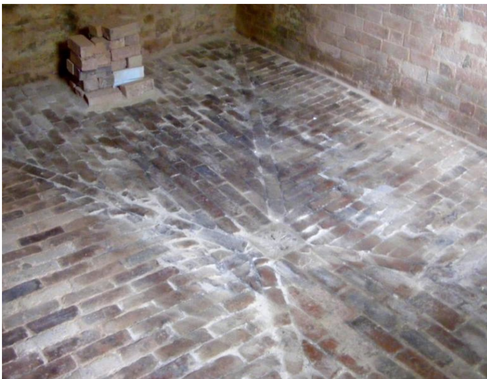
Stable 2, brick floor with central drain Fig 40
