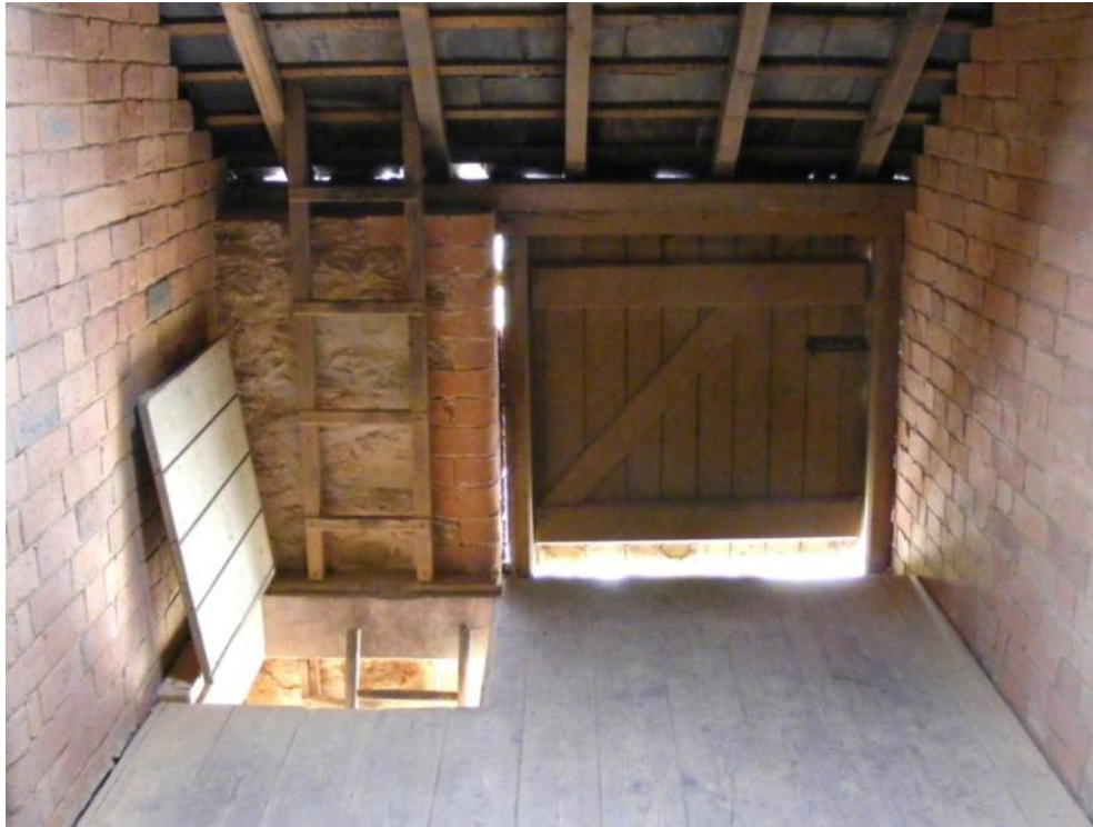
The hayloft door, trapdoor and ladder Fig 55
