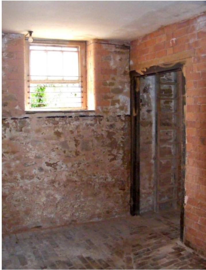
Stable 2, showing doorway and window Fig 43
