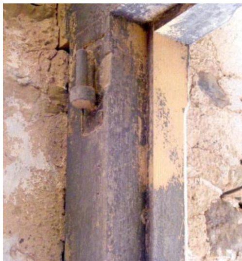
Stable 2, doorframe with pintle Fig 39
