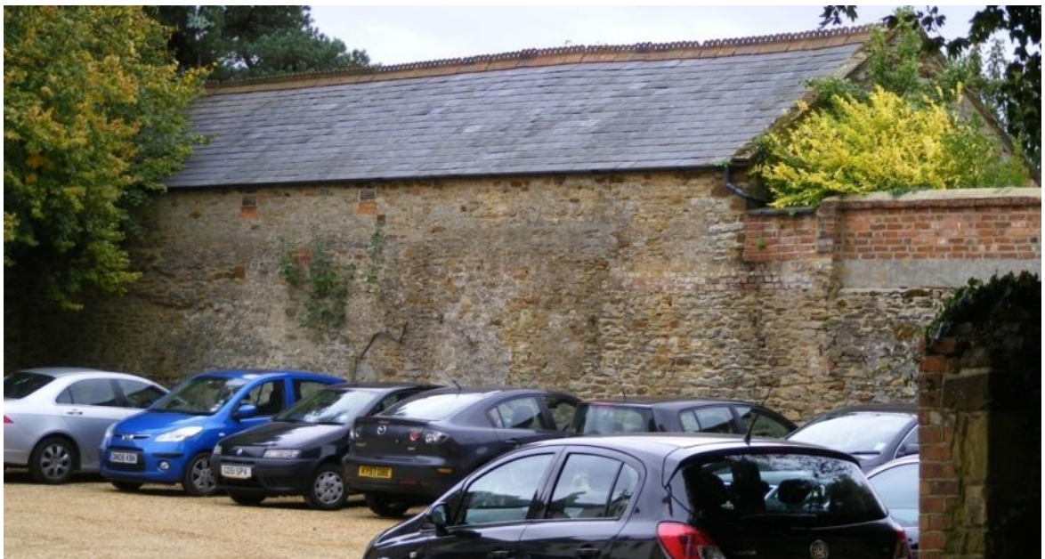
The north elevation, showing the roughly coursed ironstone wall Fig 20
