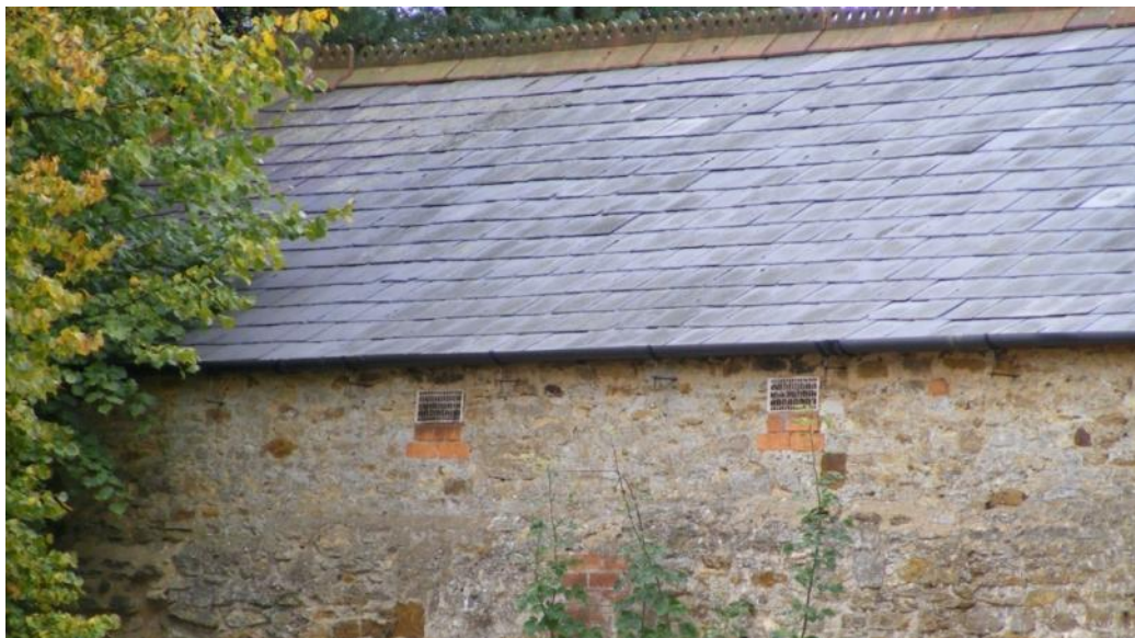
Detail of north elevation, showing metal grilles over the ventilators Fig 21
