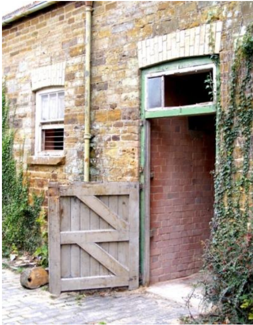
Doorway to Stable 3, and window to Stable 2 Fig 13
