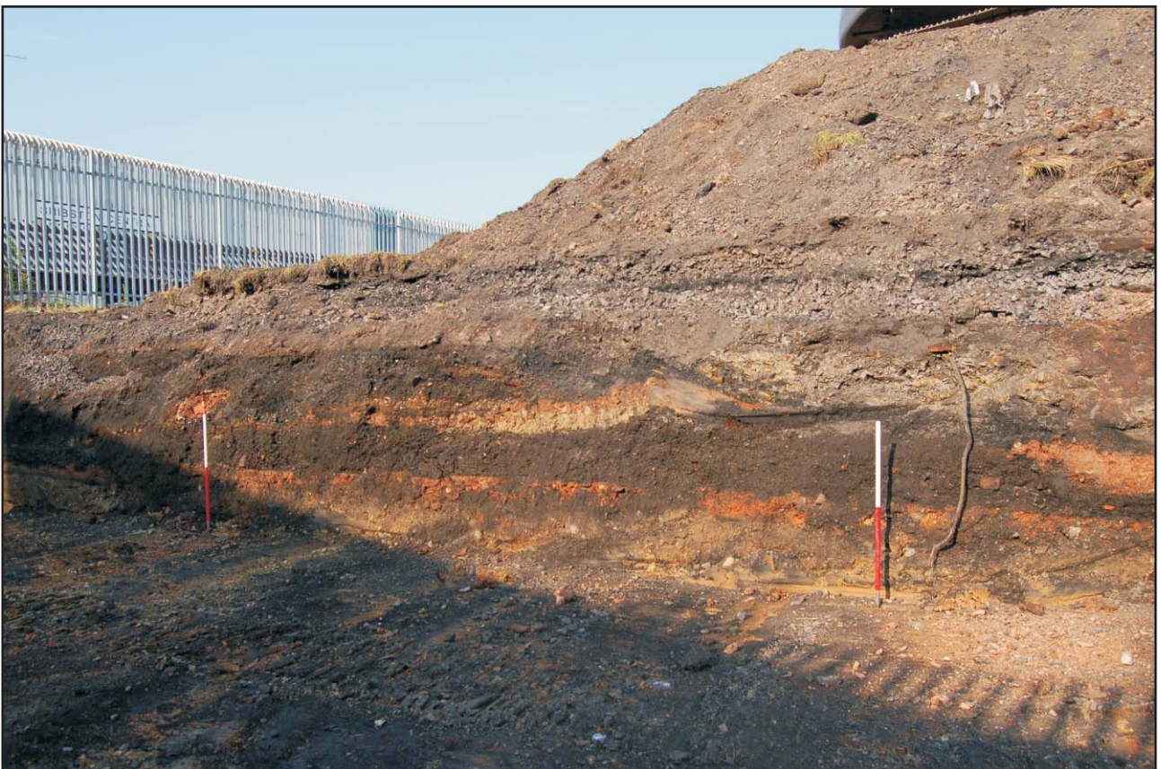
Made ground at the south-east corner of the site, looking south-west Fig 23
