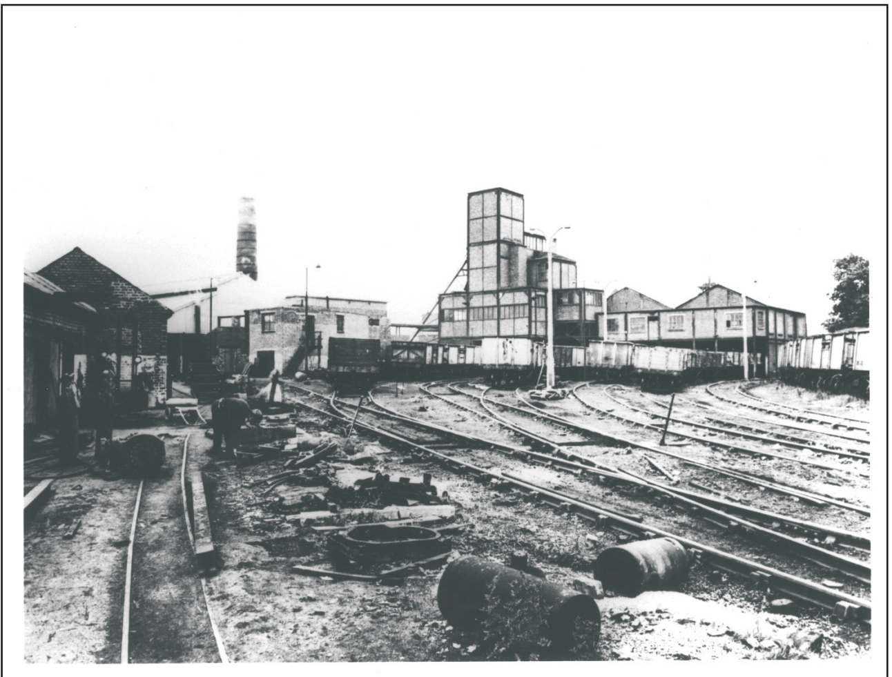
Railway tracks and ancillary buildings, looking north-east? c1962. Fig 12 Copyright Leicestershire County Council
