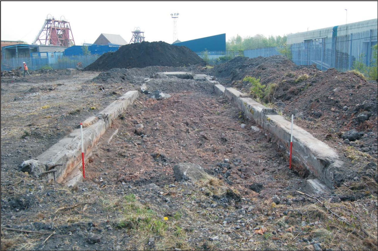
Parallel concrete foundations, looking east Fig 14
