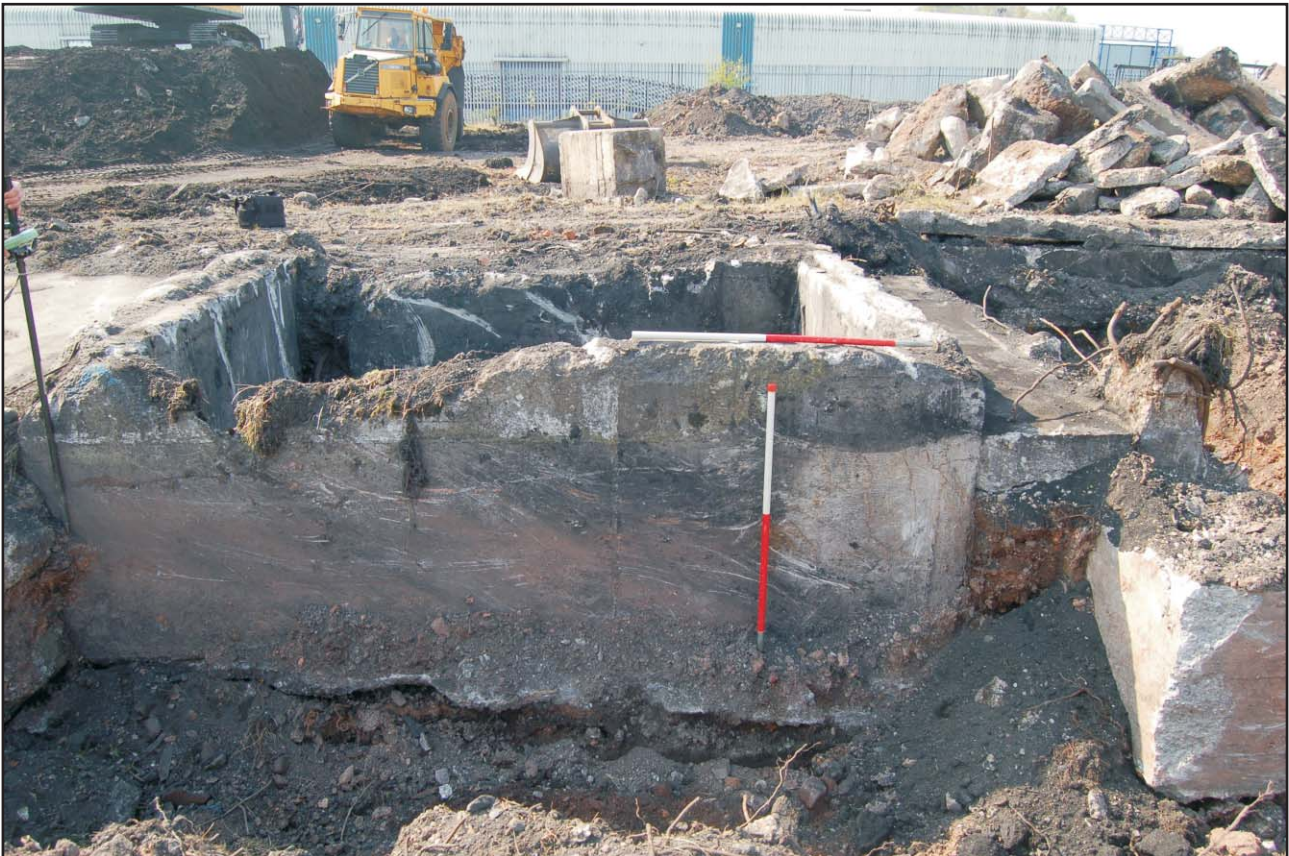
Concrete 'tank', possibly blending bunkers, looking south Fig 18
