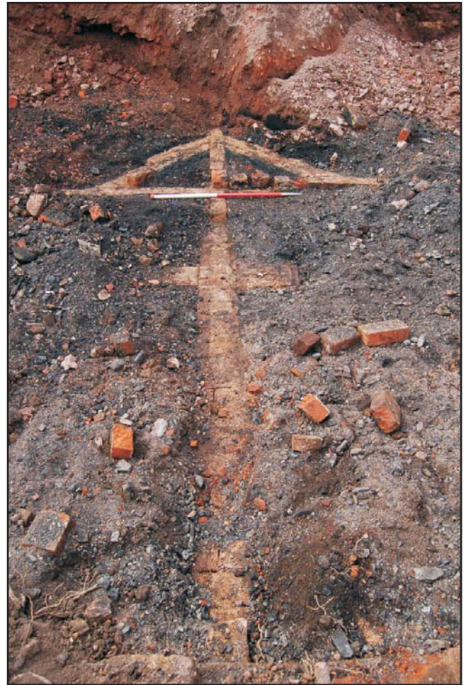
Dividing wall foundation between two cottages, looking south Fig 20
