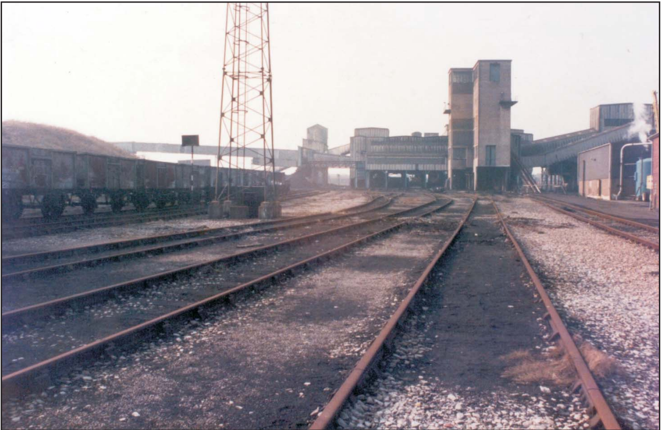
Coal preparation plant, looking west? Undated. Copyright Leicestershire County Council Fig 11
