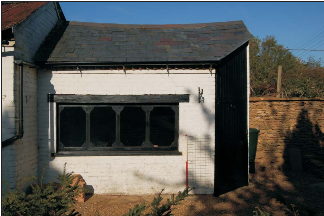
Store room, south elevation, looking north Plate 11
