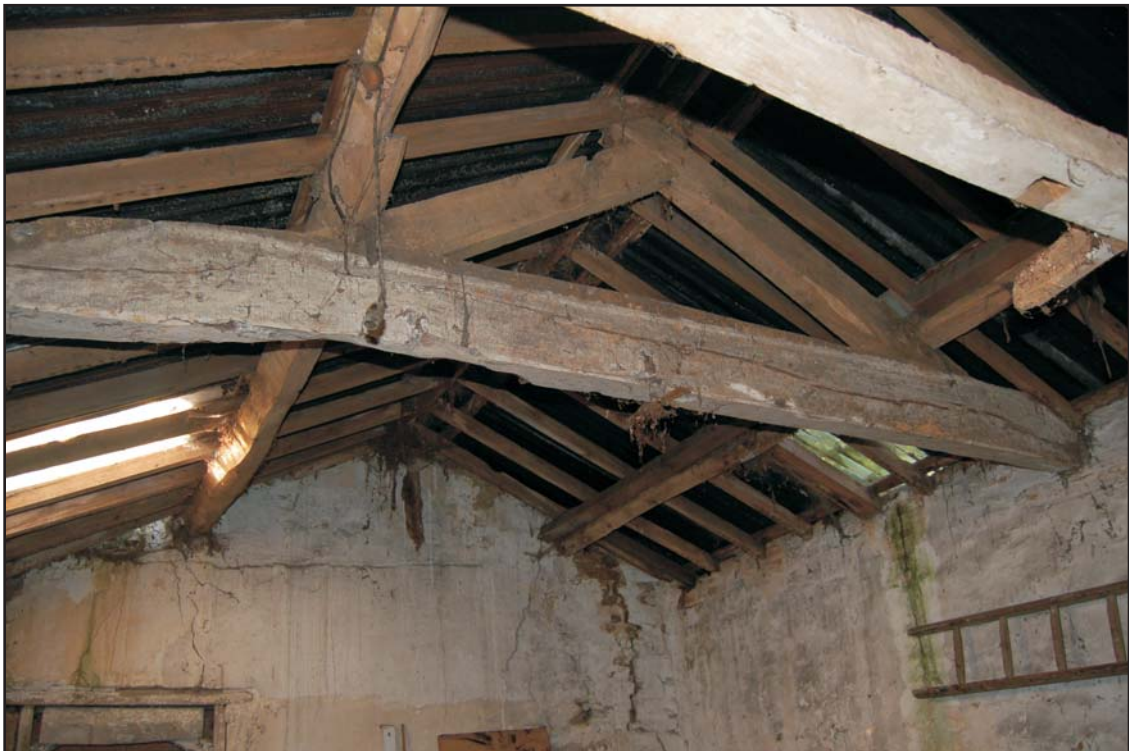
Roof truss in the west stalls, looking west Plate 7
