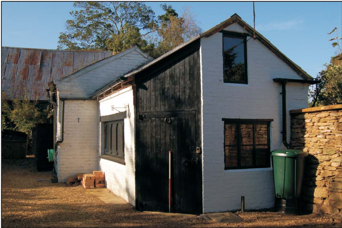
Store room, east elevation, looking west Plate 12
