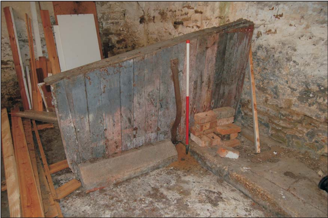
Timber travise in the west stalls, looking west Plate 9
