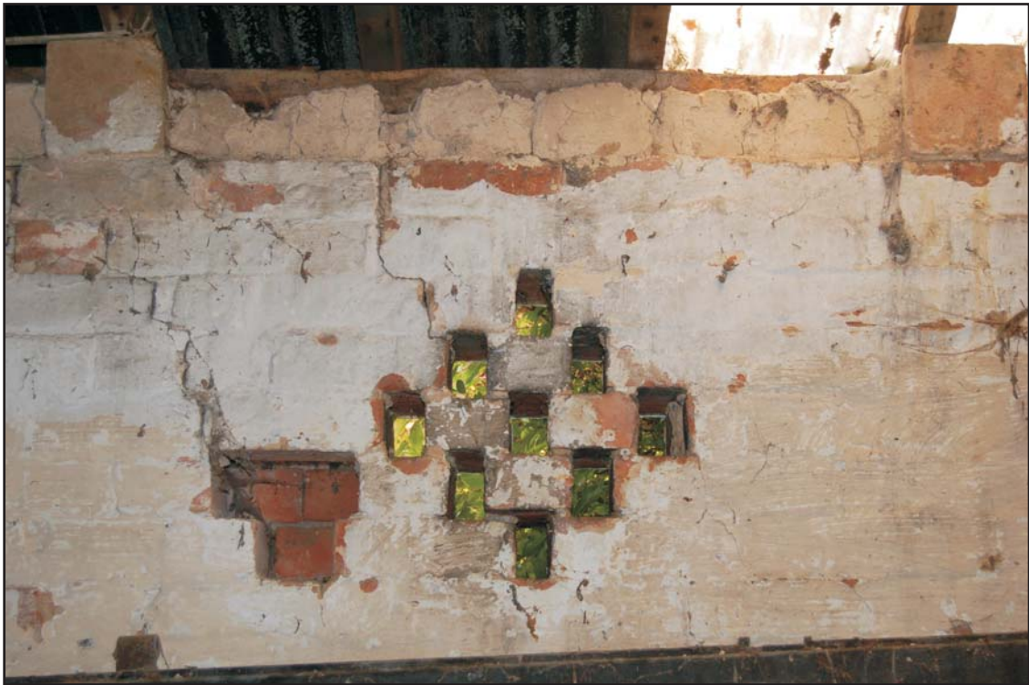
Ventilation grid in south elevation, interior, looking south
