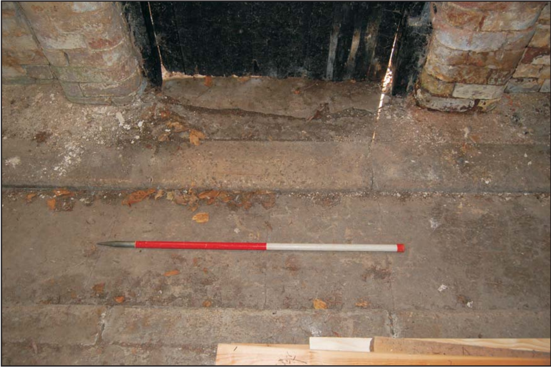
Pre-cast concrete road kerbs used to edge the drainage gully, looking south Plate 8
