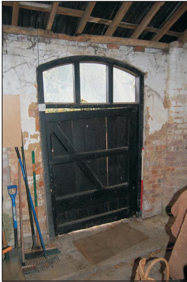
Door in Arch 3, interior, looking south Plate 10
