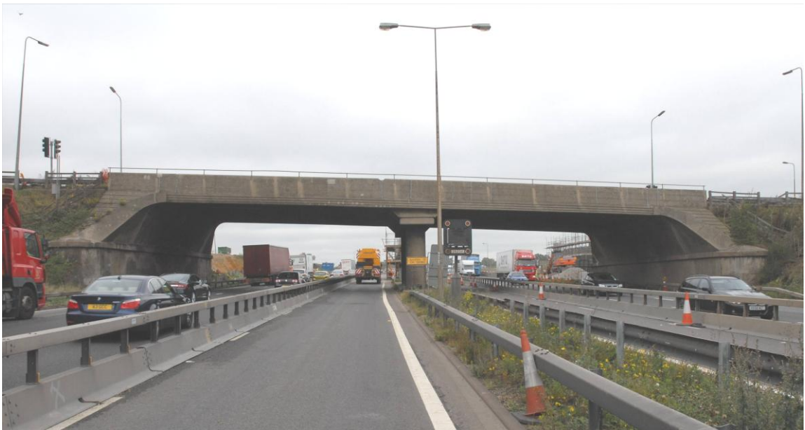
M1 Junction 12 Overbridge, looking north-west
