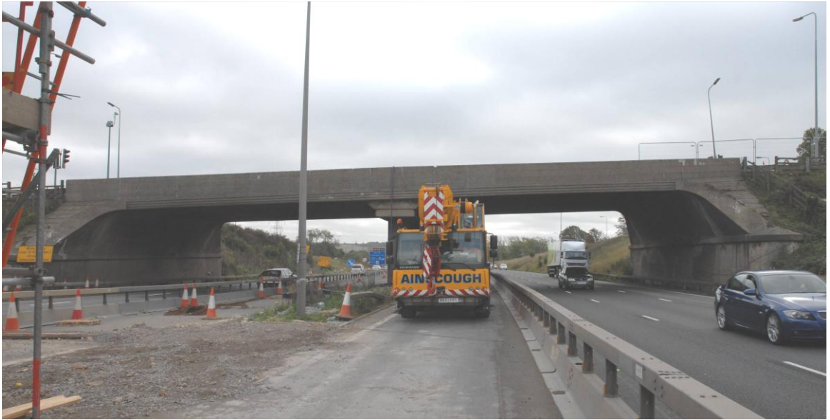
M1 Junction 12 Overbridge, looking south-east
