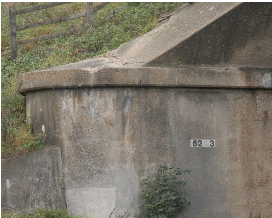
The stencilled bridge number, looking south-west
