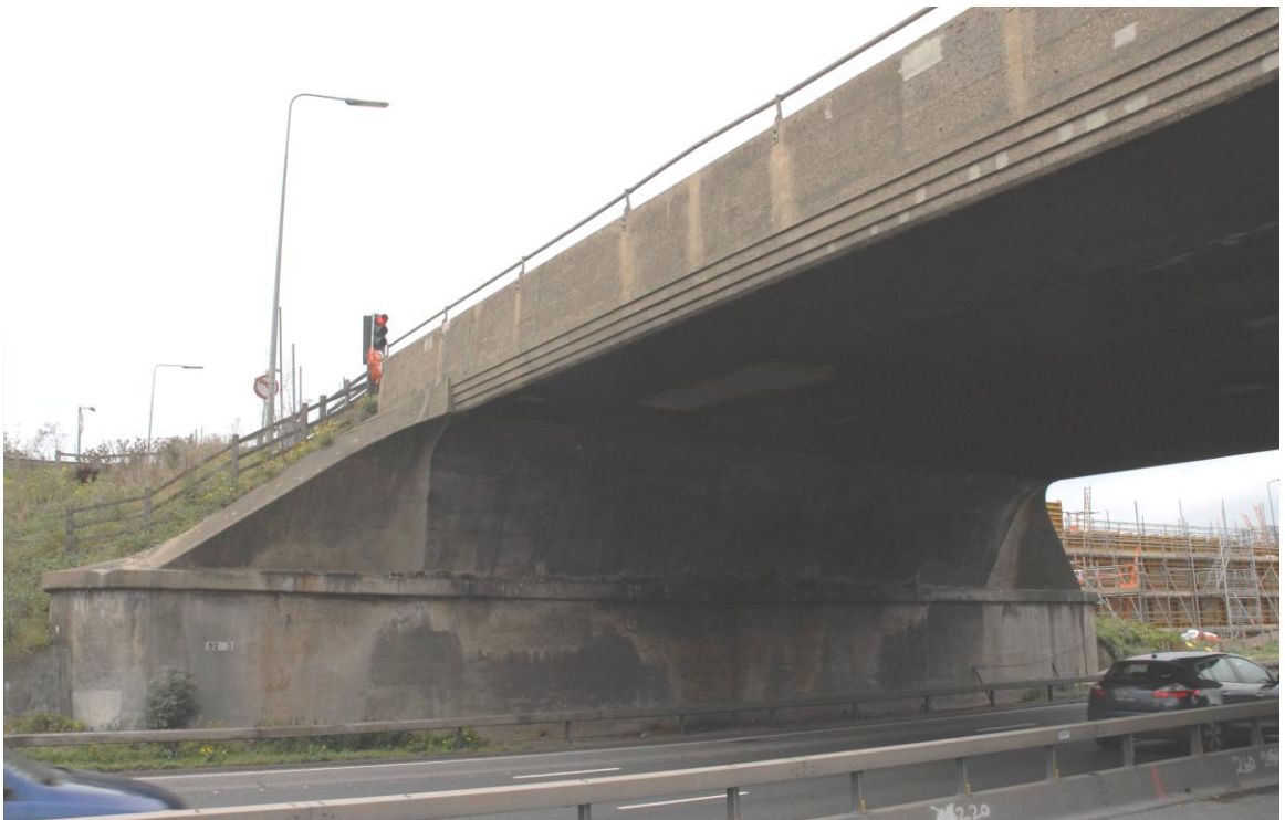
M1 Junction 12 Overbridge, looking west
