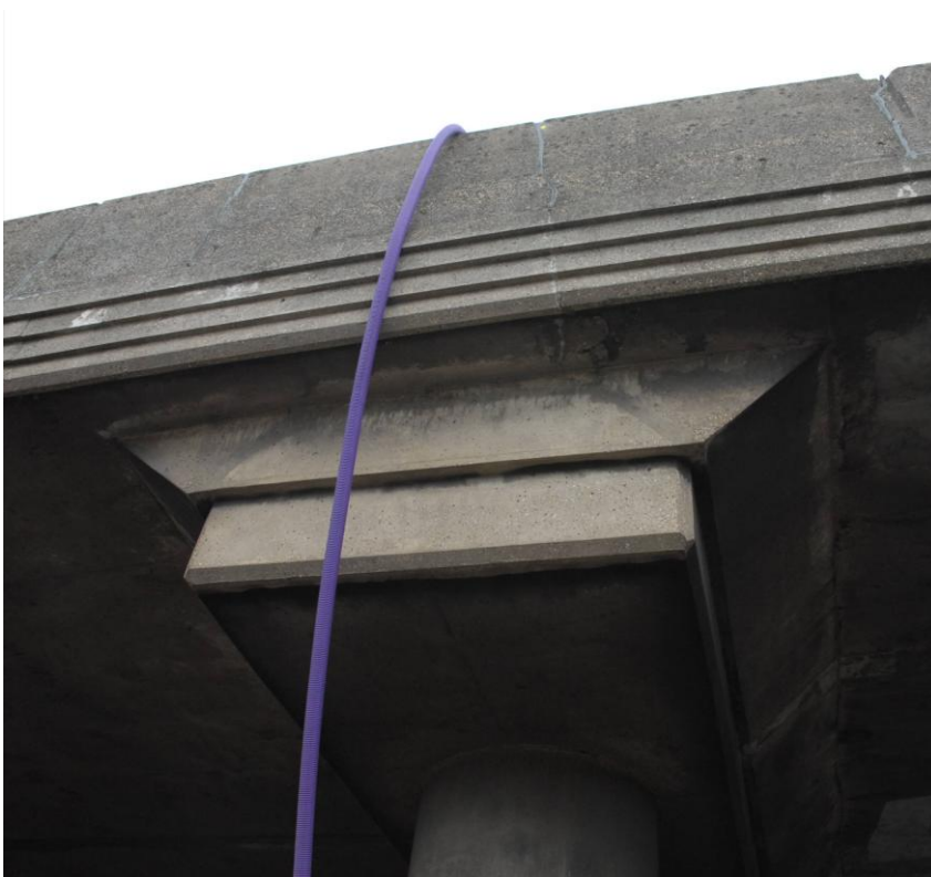
Column capital detail, looking south-east, also showing the corbelled soffit
