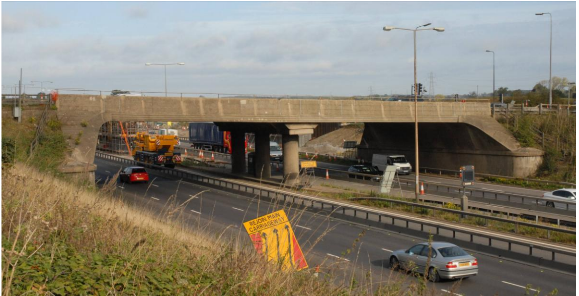
South-eastern elevation, looking north
