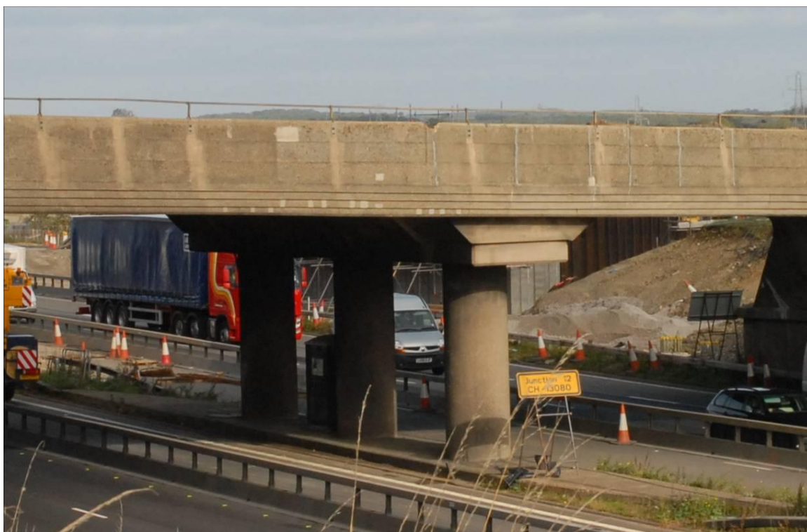
M1 Junction 12 Overbridge, column detail, looking north
