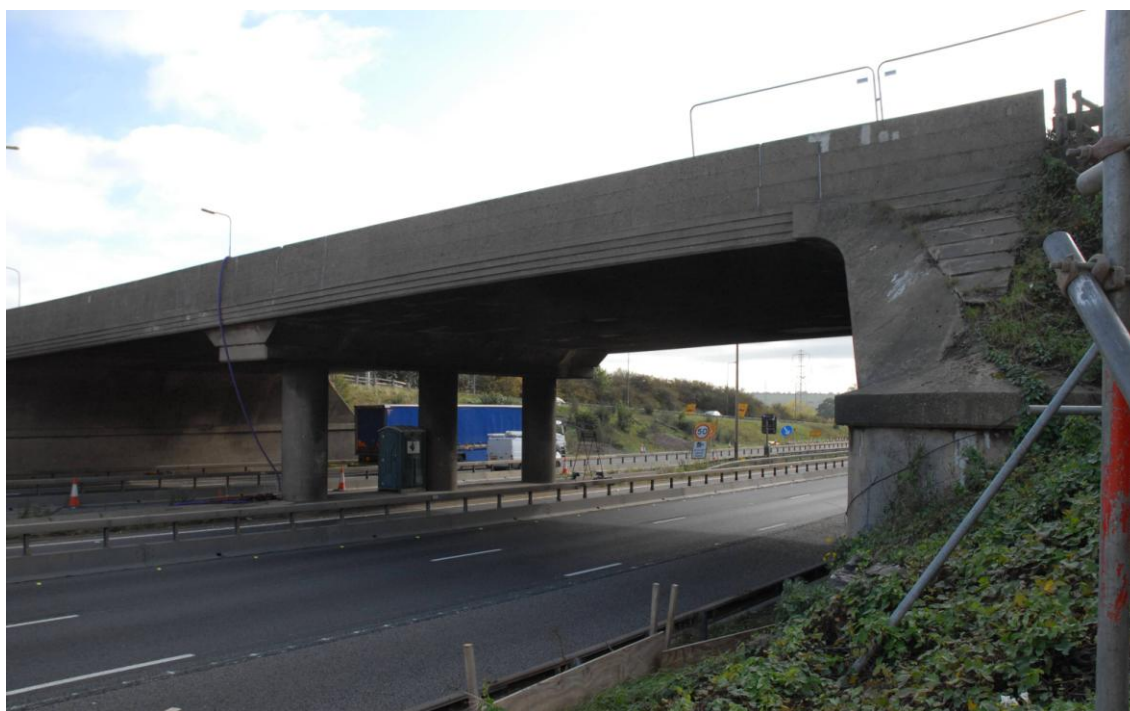
North-western elevation, looking south-east
