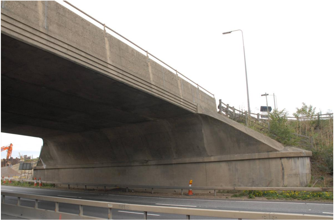
Detail of the inclined tapering haunches, looking north-east
