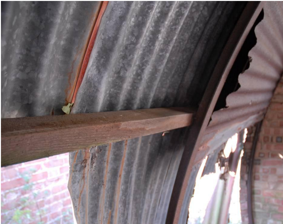
Purlin detail, Hut 143
