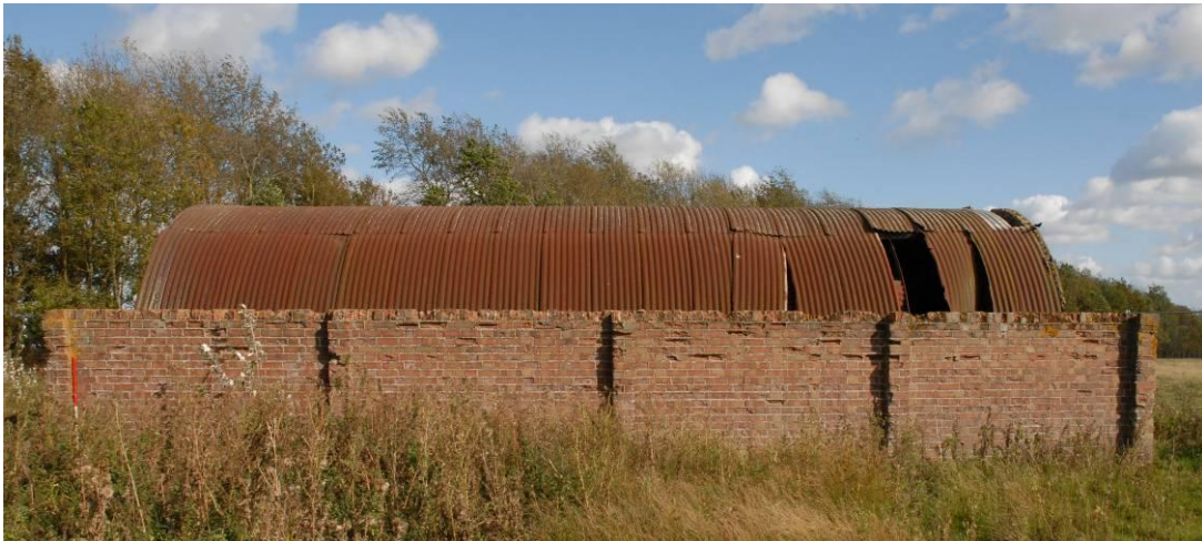
View looking east showing the dividing wall
