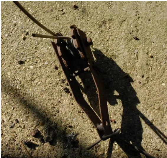
Straining ratchet detail, Hut 143 Fig 18
