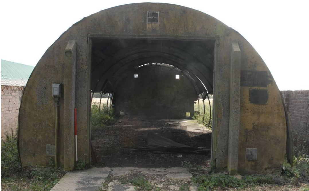
Front wall of Hut 143, looking south Fig 12
