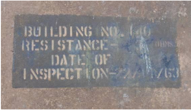
Stencilled panel on Hut 140
