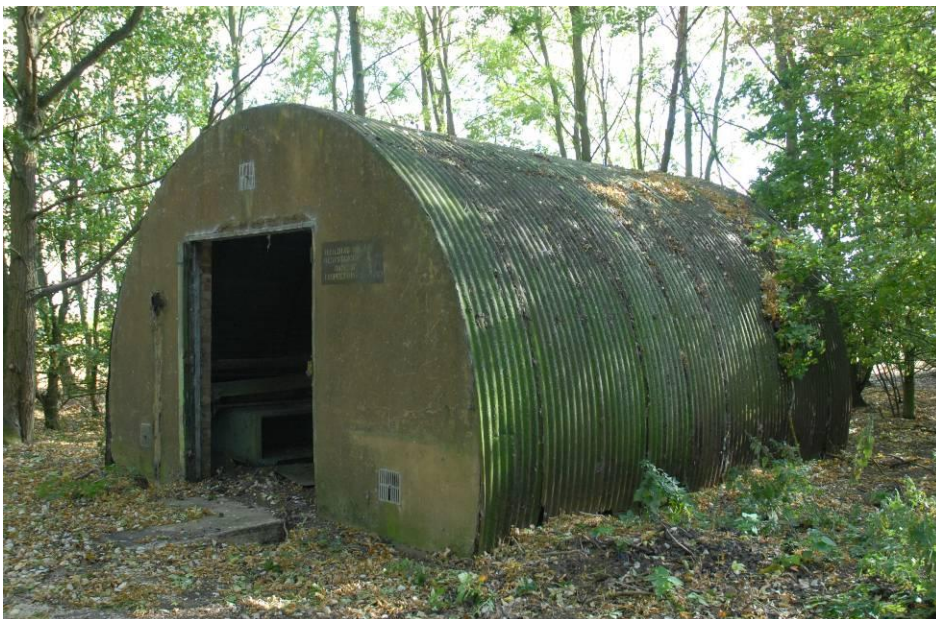
Hut 140, looking south-east
