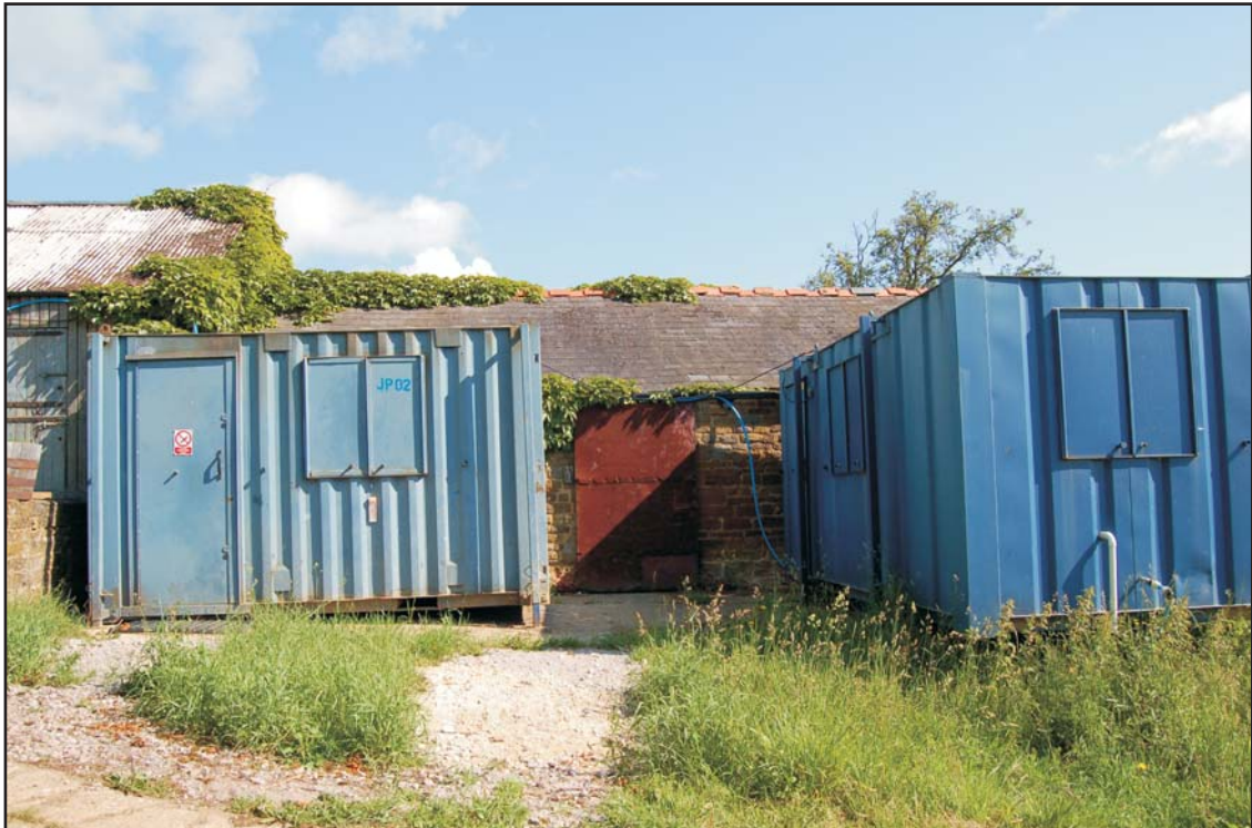
Stock building SB3, looking north Plate 16
