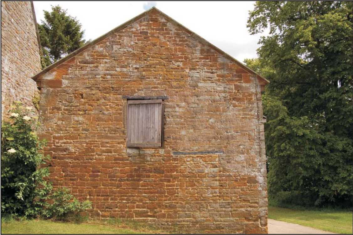
The detached stable west elevation, looking east Plate 3
