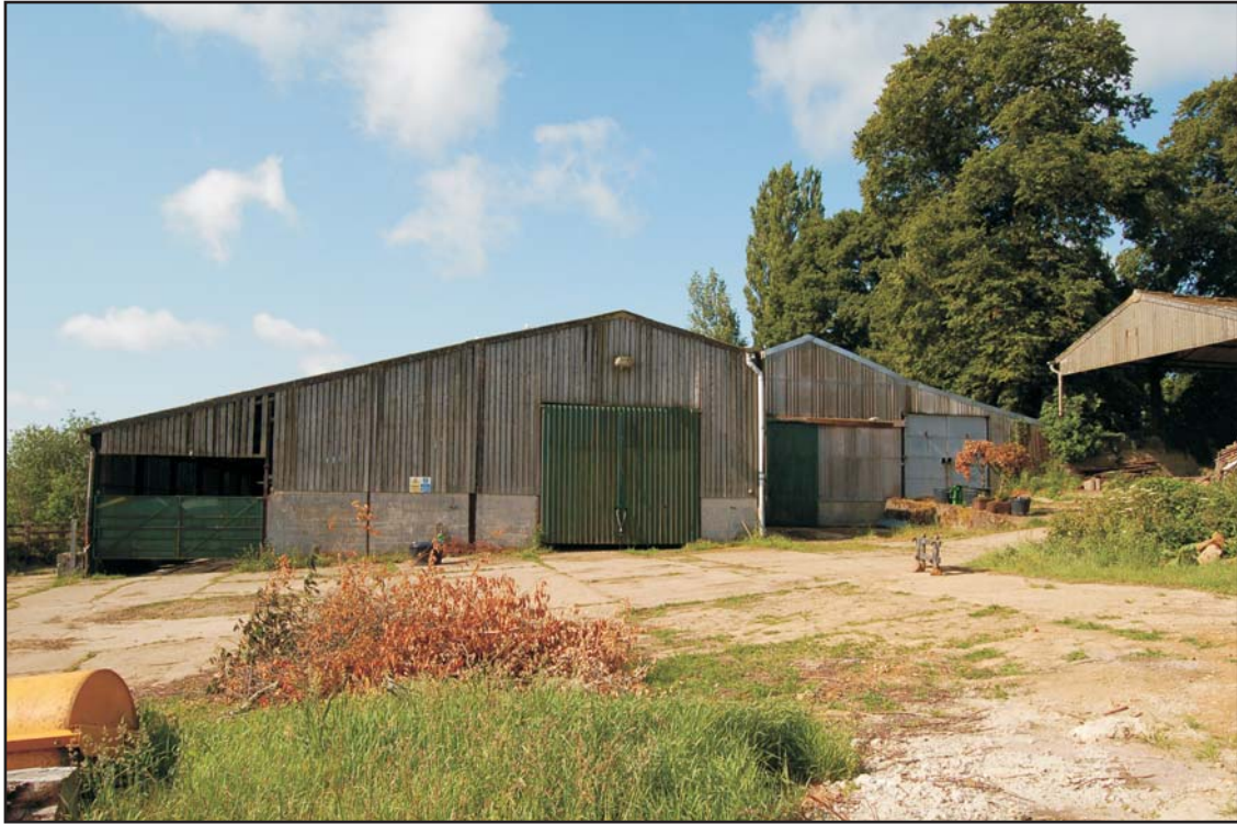
Conjoined steel framed sheds, looking south Plate 19
