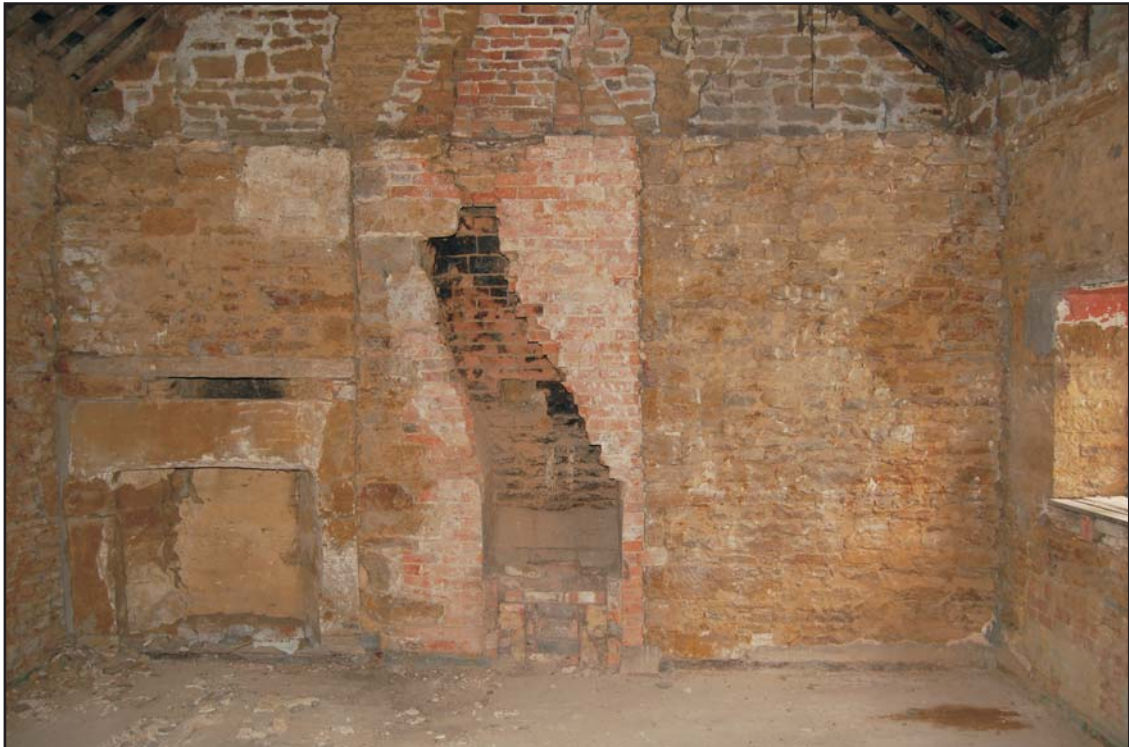
The detached stable, Room F2, east wall, looking east Plate 12
