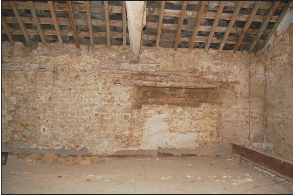
The detached stable, Room F1, blocked window in south wall, looking south Plate 9
