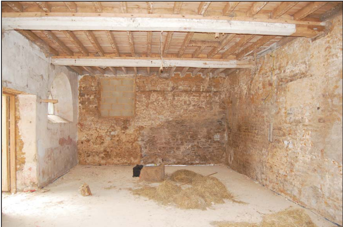
The detached stable, Room G1, looking west Plate 6
