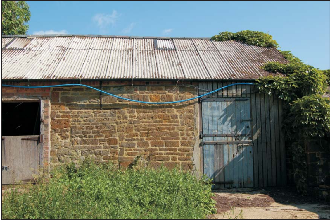
Stock building SB2, looking north Plate 15
