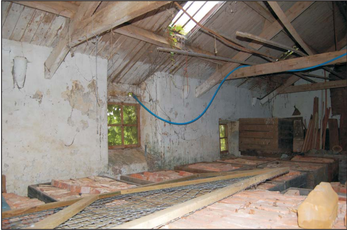
Stock building SB3, interior, looking north-east Plate 17
