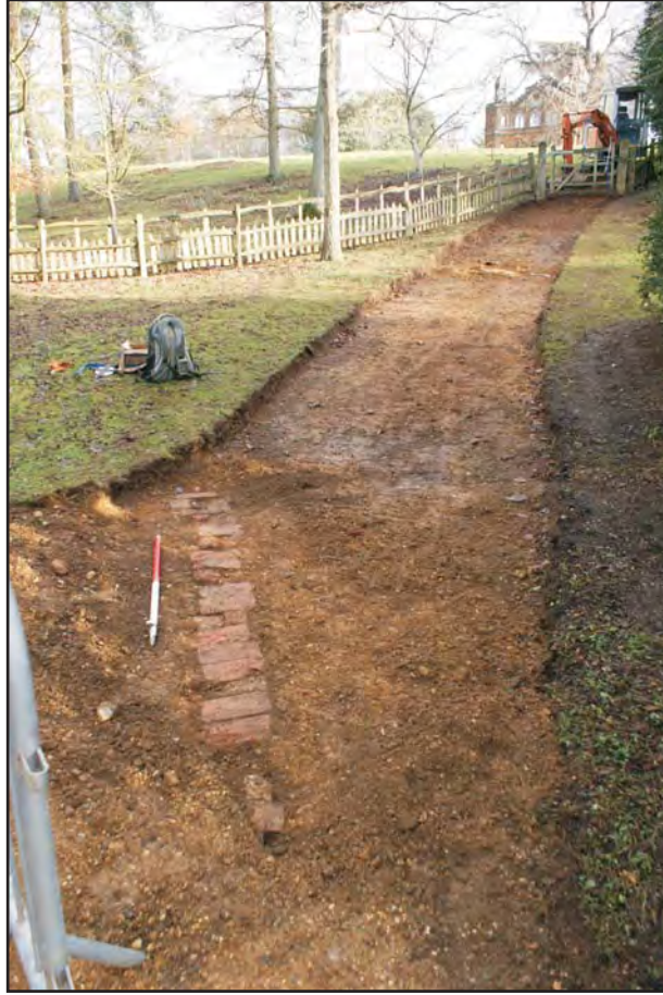
Drain 3, looking north Plate 7
