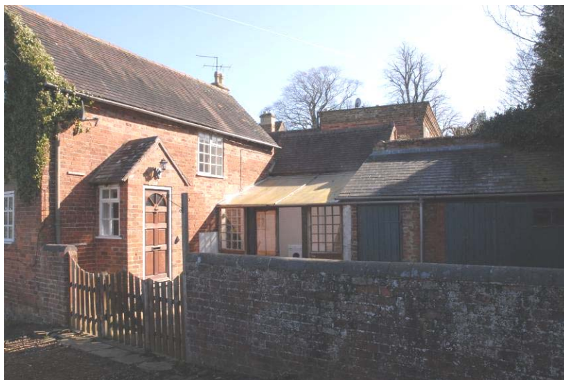
The Cottage, utility room Fig 14
