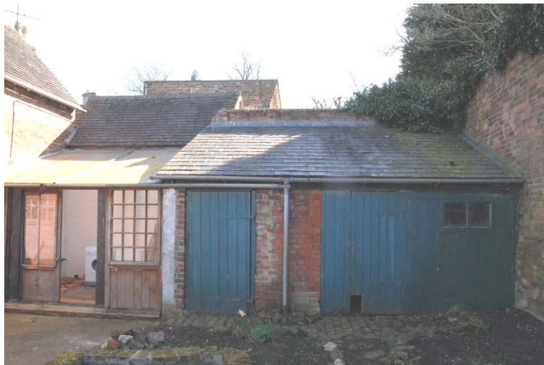
The Cottage, adjacent shed Fig 13
