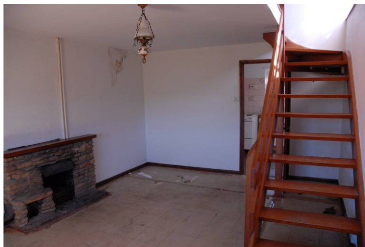
The Cottage, ground floor interior Fig 11
