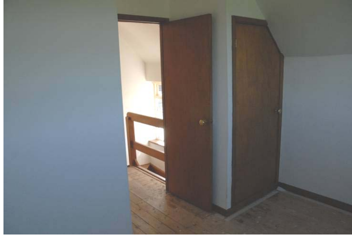
The Cottage, first floor interior Fig 12
