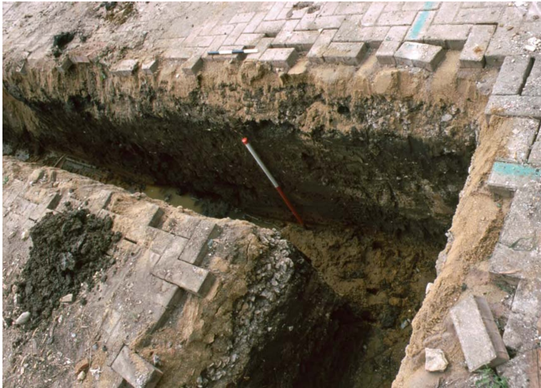
Pit [317] within the foundation of Building 1 Fig 3
