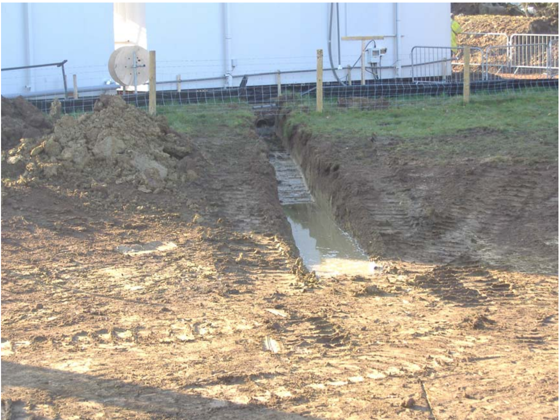
Plate 10: The water pipe trench entering the swale pit
