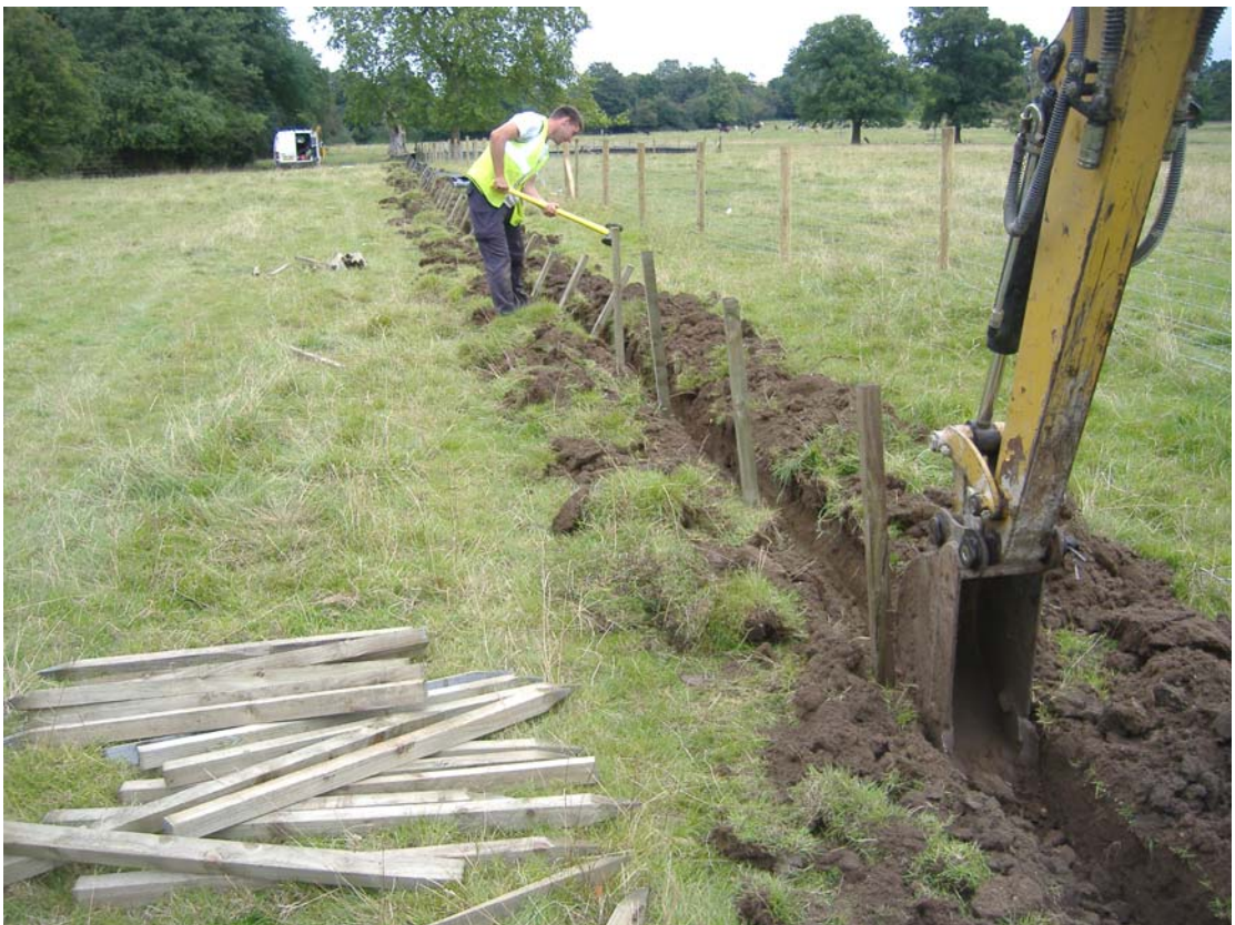
Plate 2: Construction of the newt fence
