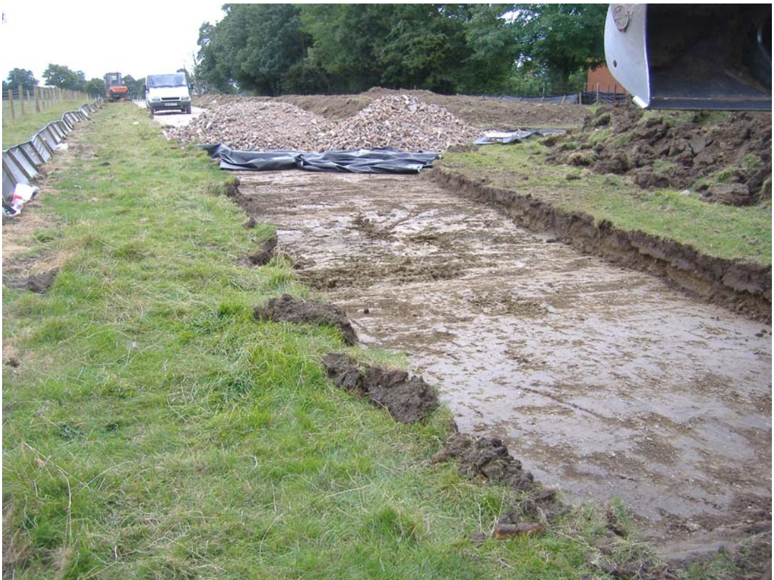
Plate 4: Laying of hardcore along the temporary access road
