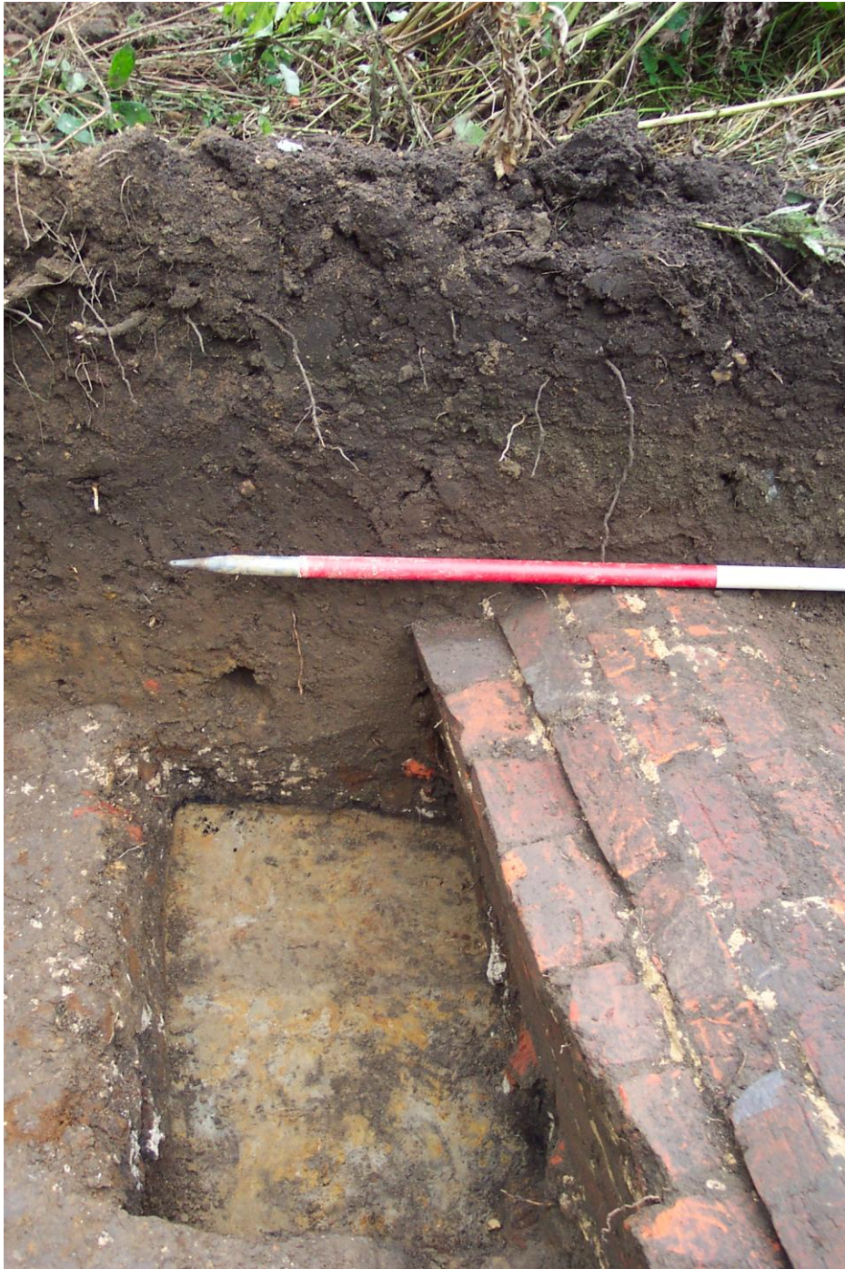
Plate 1: Post- medieval brick built drain showing underlying rubble layer and enveloping sandstone rubble layer
