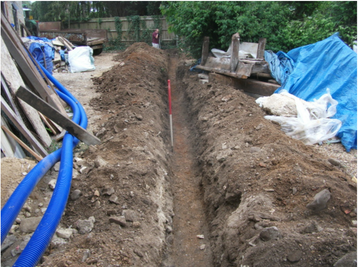
The drainage trench after excavation, looking north-east Fig 6
