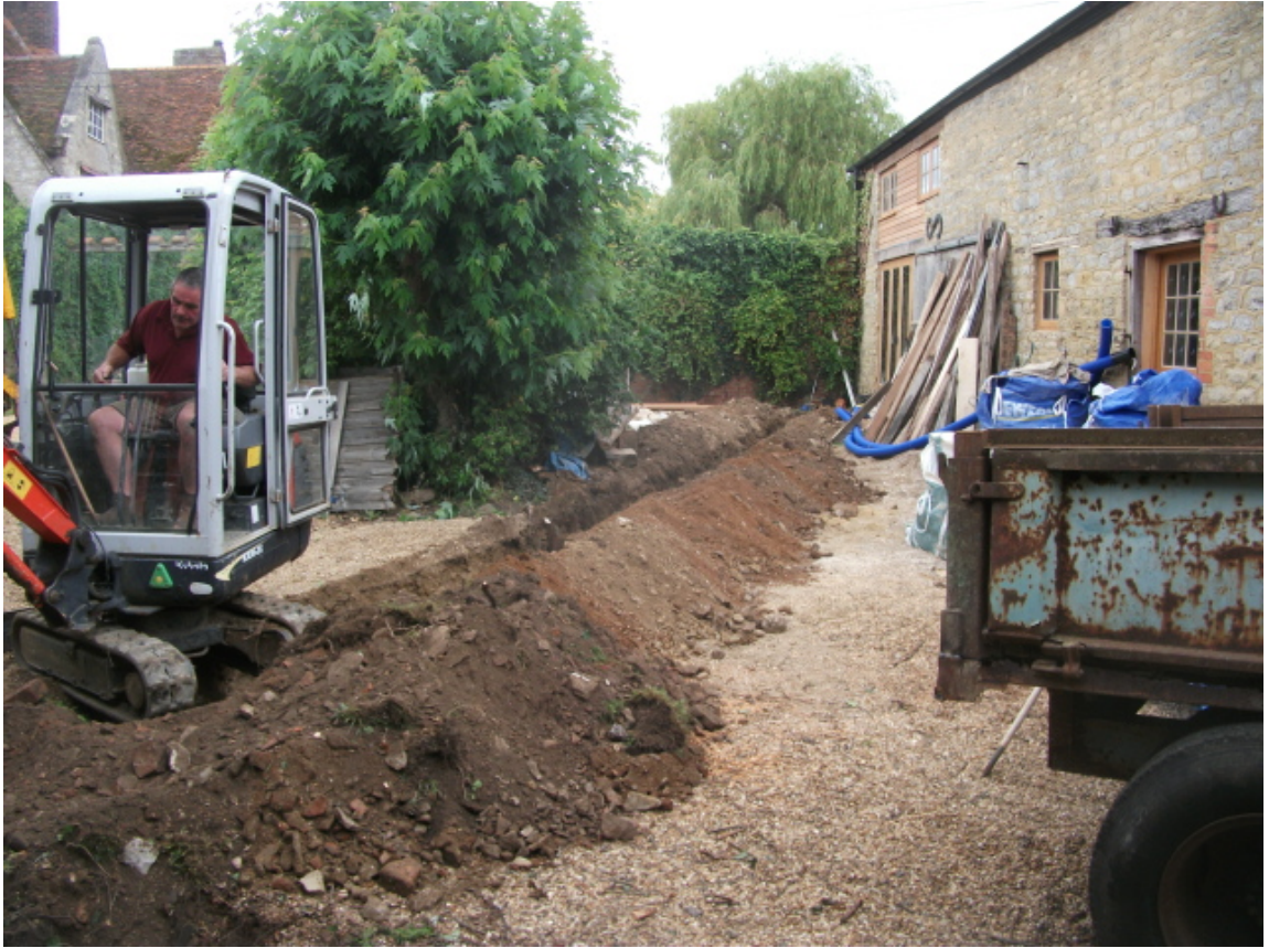
The drainage trench with the carriage house in the background Fig 5
