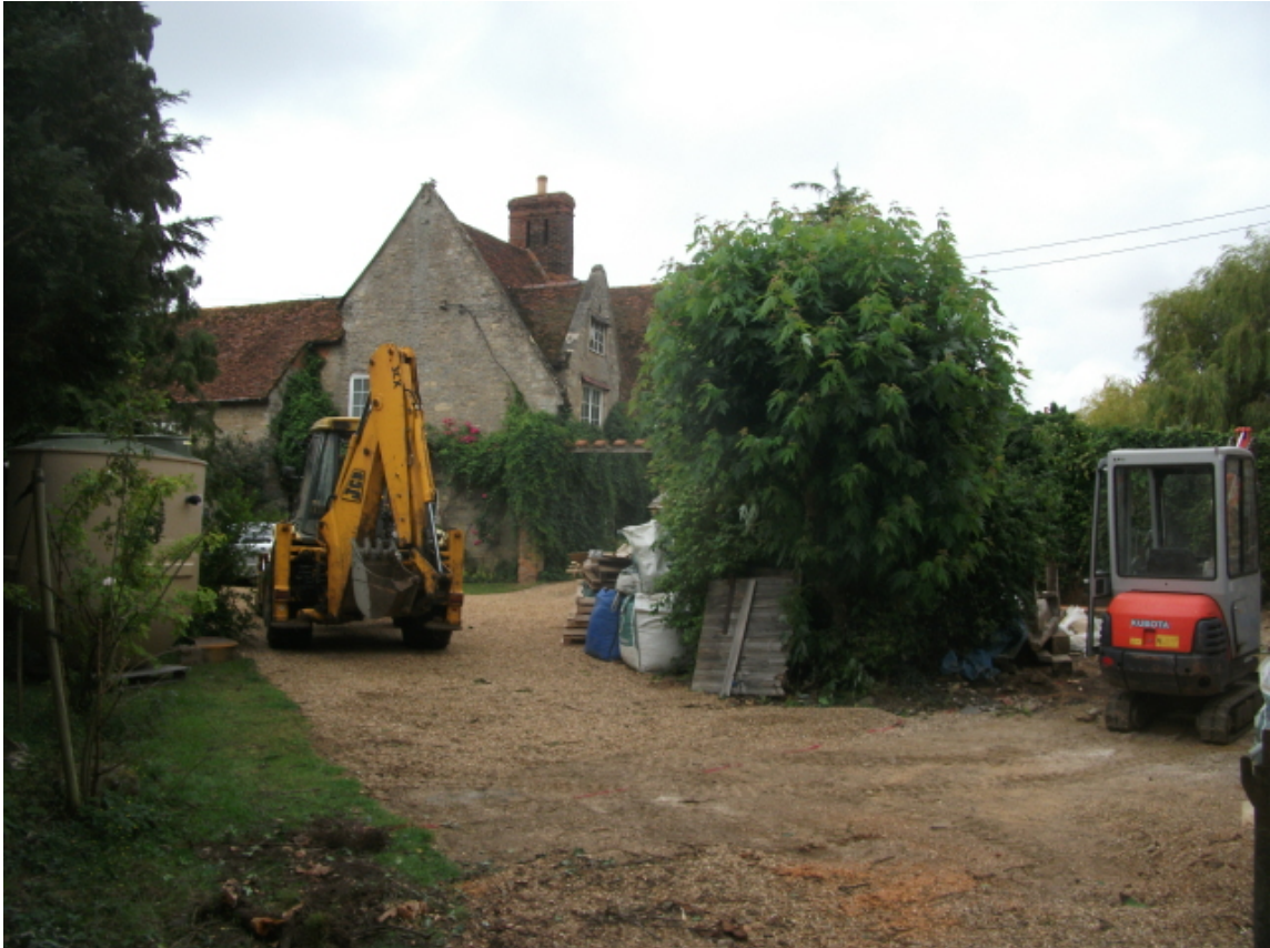
The investigation area at the start of groundworks, looking south-east Fig 3
