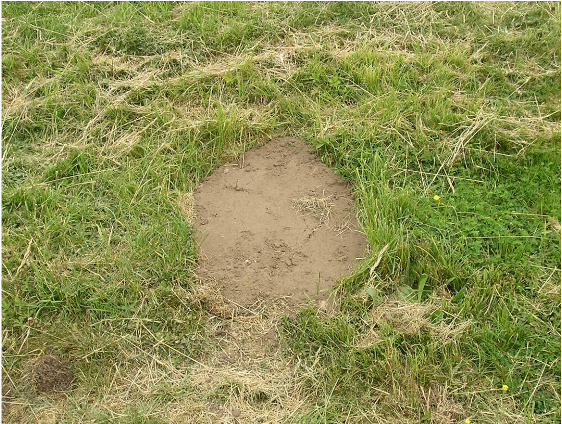
Rabbit damage to the bank filled with excess natural spoil and imported topsoil Fig 9
