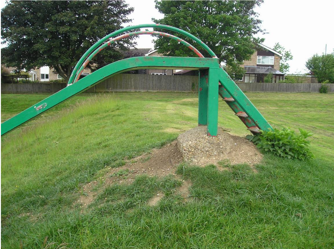
Erosion around the slide Fig 11
