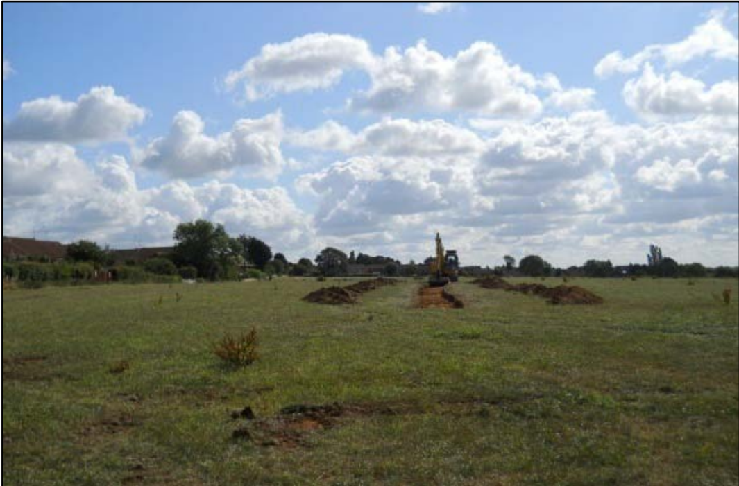
General view of Field 1, with Trench 2 being excavated, looking west Fig 3
