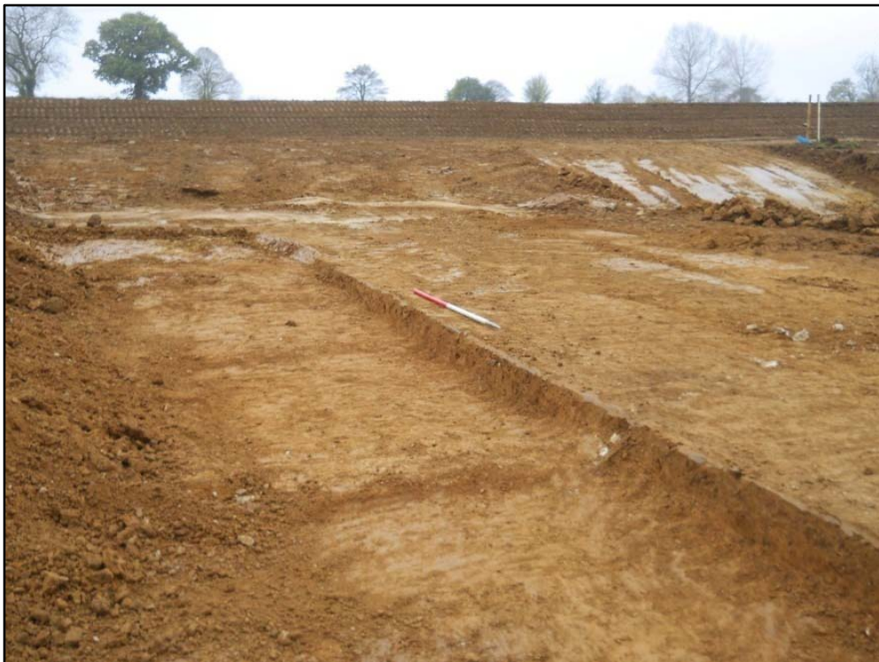
General view of extraction pit [716], looking south-west Fig 8
