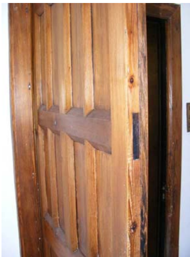
Room G2, the laminated door Fig 28
