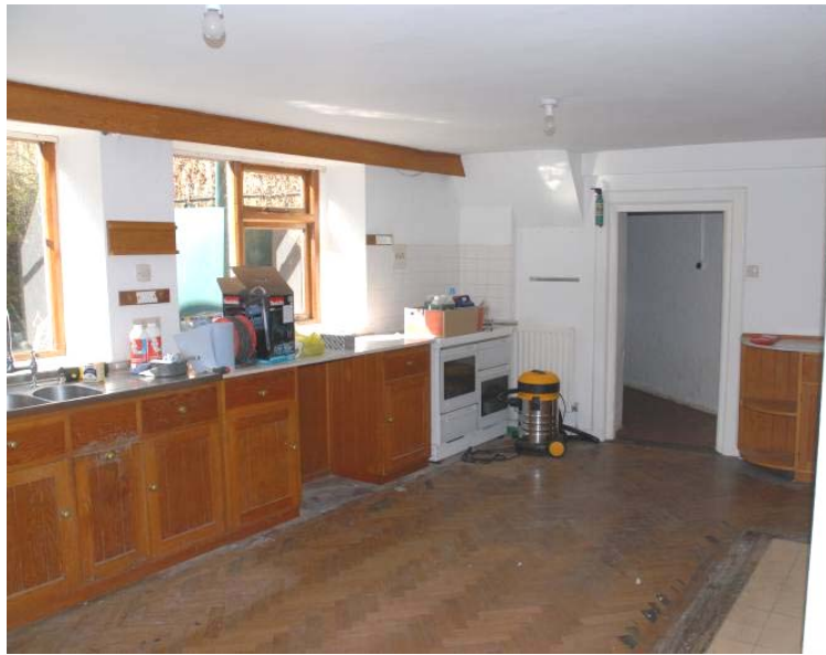
Room G4, looking south-west
