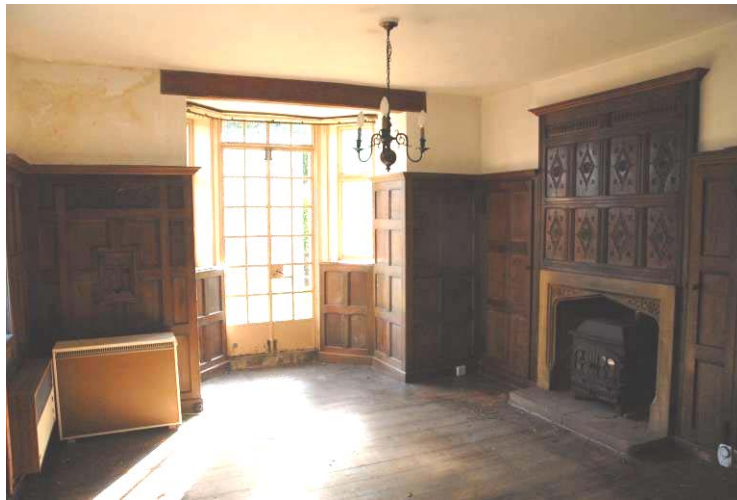
General view of Room G1 Fig 25
