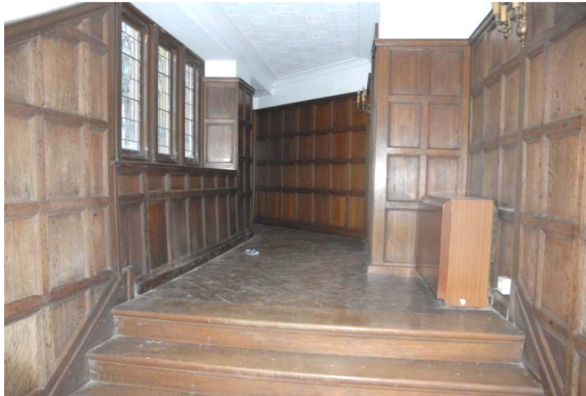
Corridor G8, 1920s panelling inserted Fig 35
