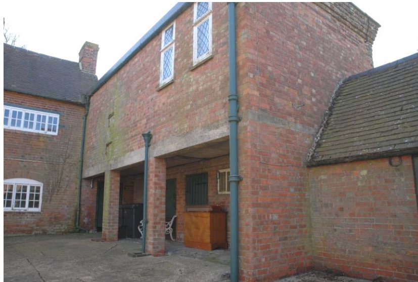
The 1930s store-rooms under the garden room, G15
