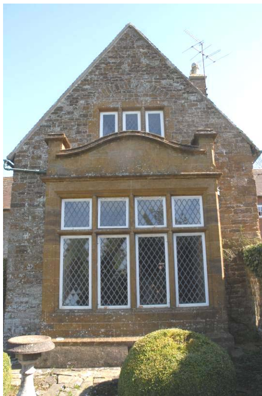
1925-8 Stone bay window on G11 Fig 39
