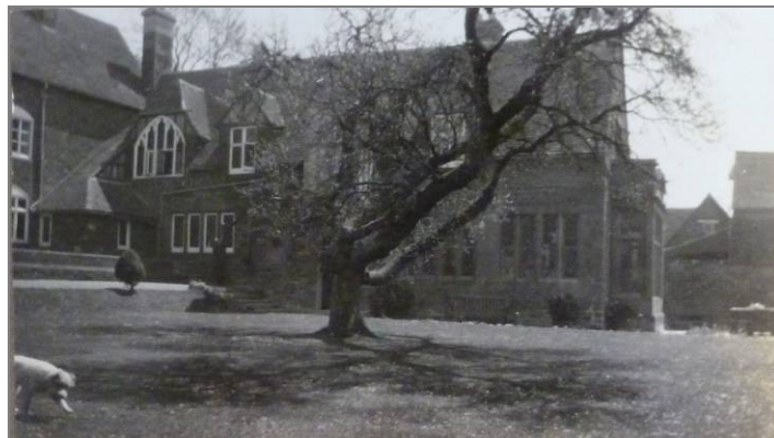
Photograph showing projecting bay window, 1929 (Note too the four-light window on the ground floor) Fig 20
