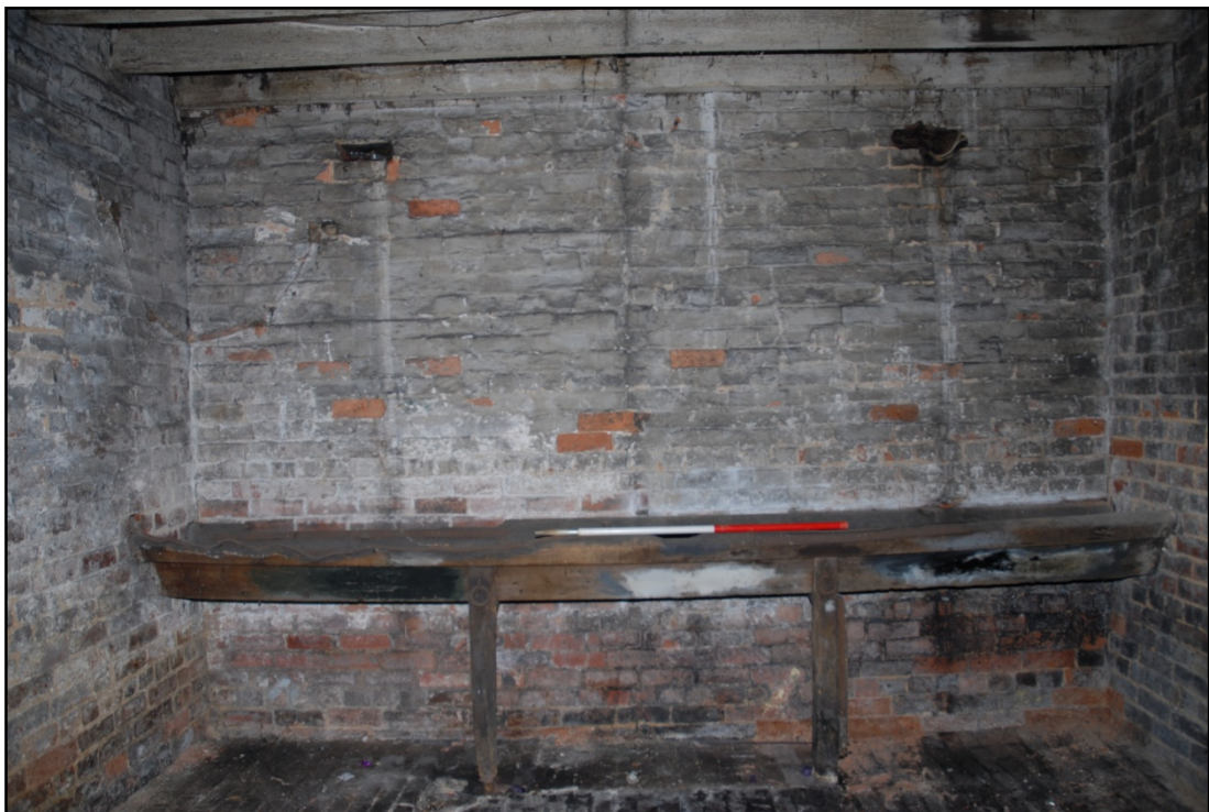
The trough in the stable with tethering rings visible Fig 18
