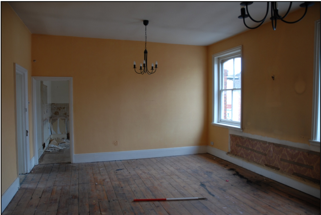
The first floor living room Fig 14
