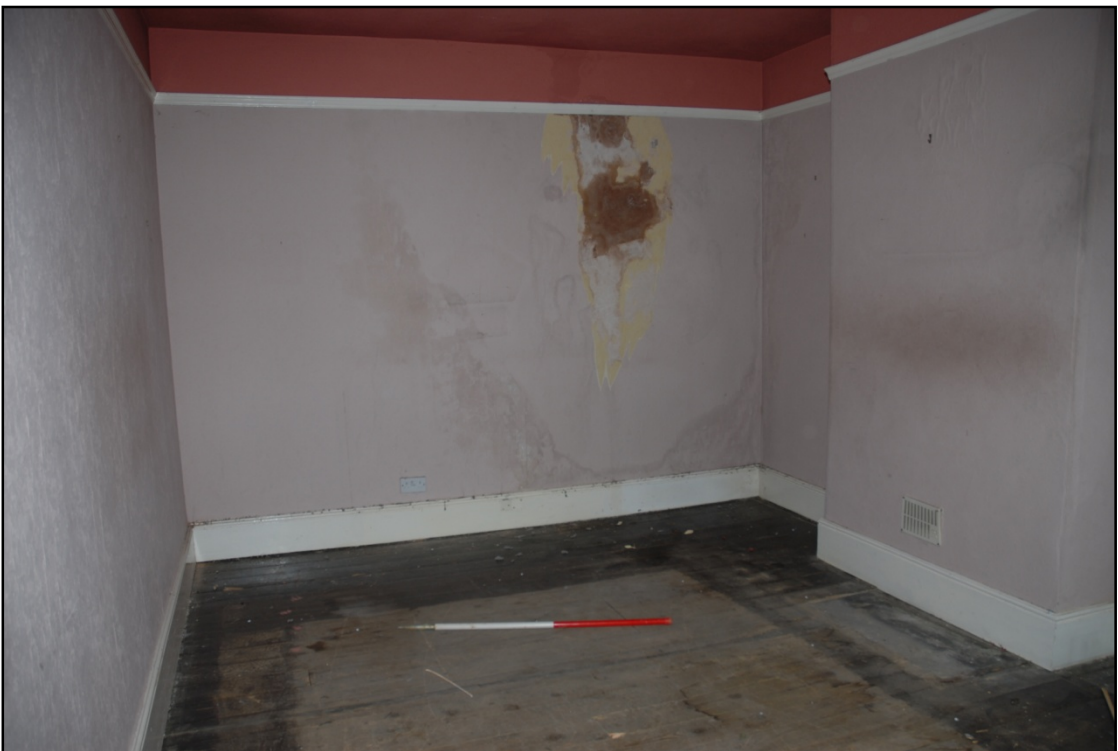
Bedroom 2, showing the blocked fireplace Fig 16
