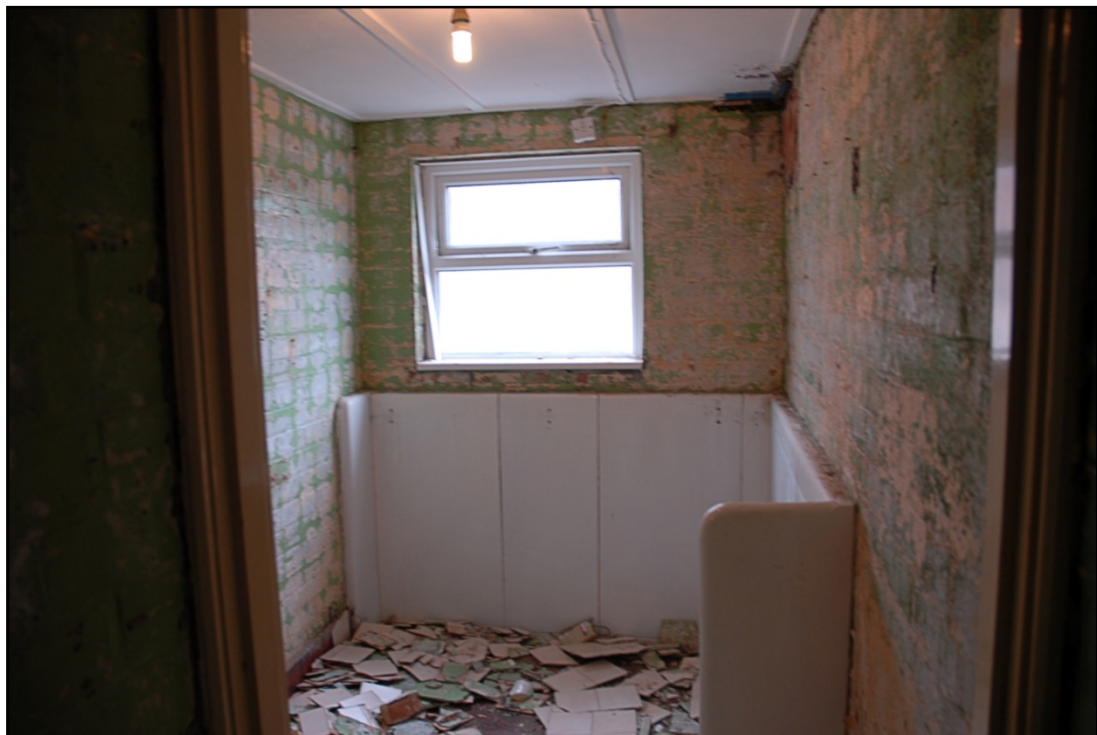
The toilet block Fig 10
