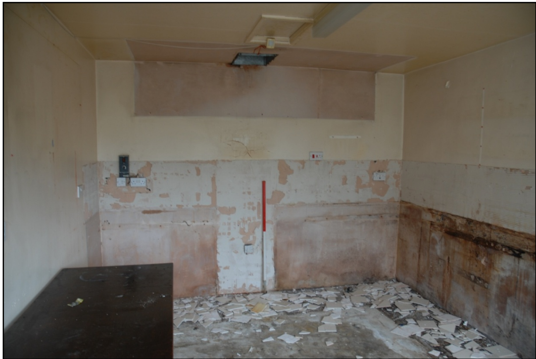
The ground floor kitchen, looking east Fig 8
