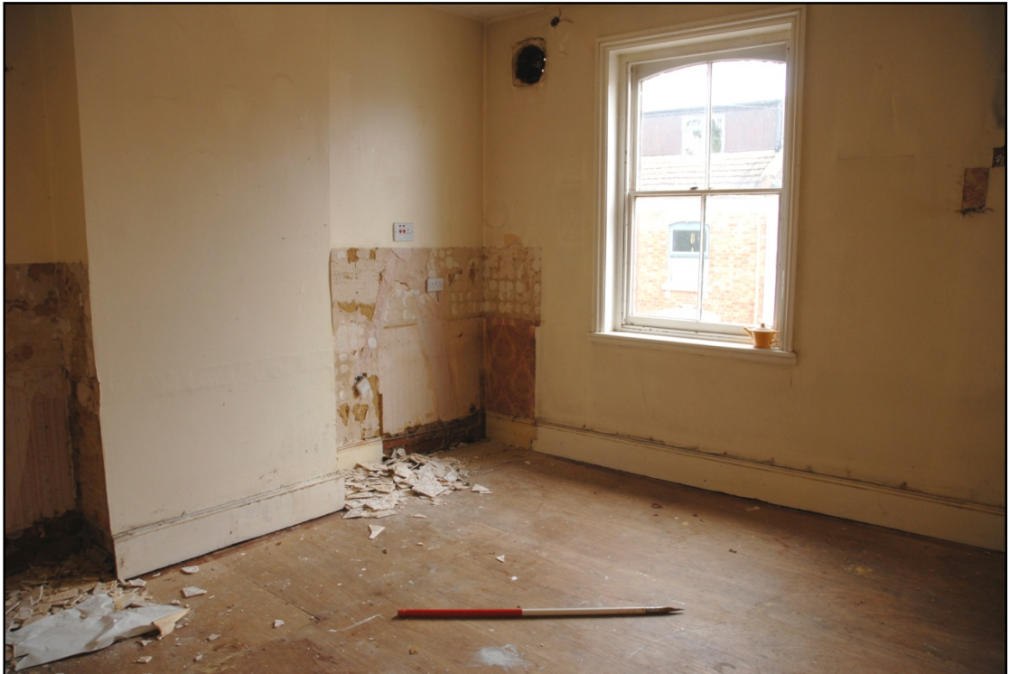
The first floor kitchen Fig 15
