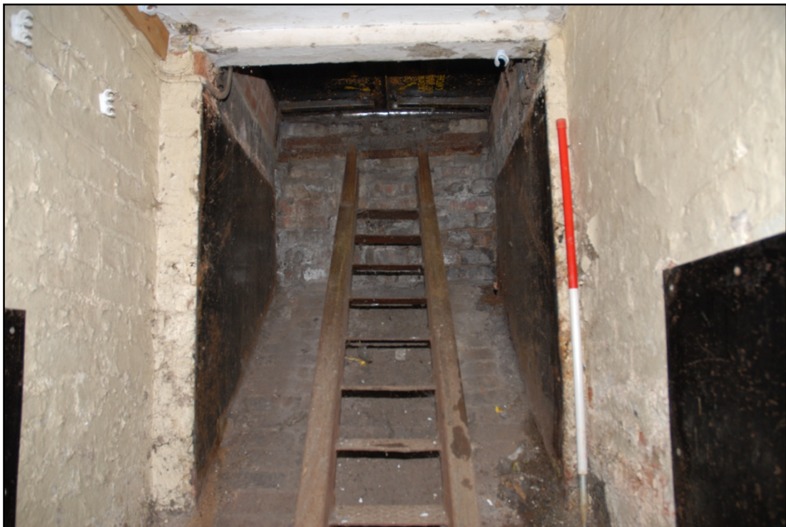
The cellar chute and trapdoor Fig 12
