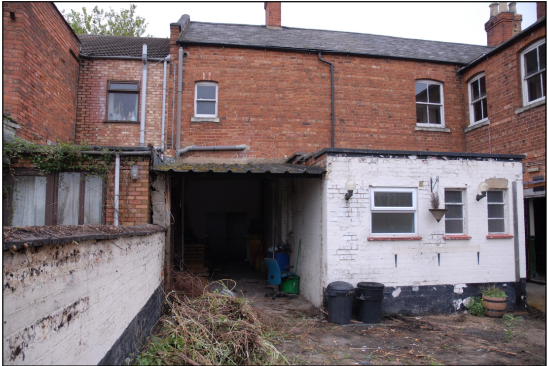
The south elevation showing the toilet block and passageway Fig 19
