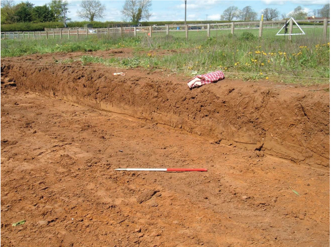
Natural substrate exposed during levelling for the east house, looking north-west Fig 4
