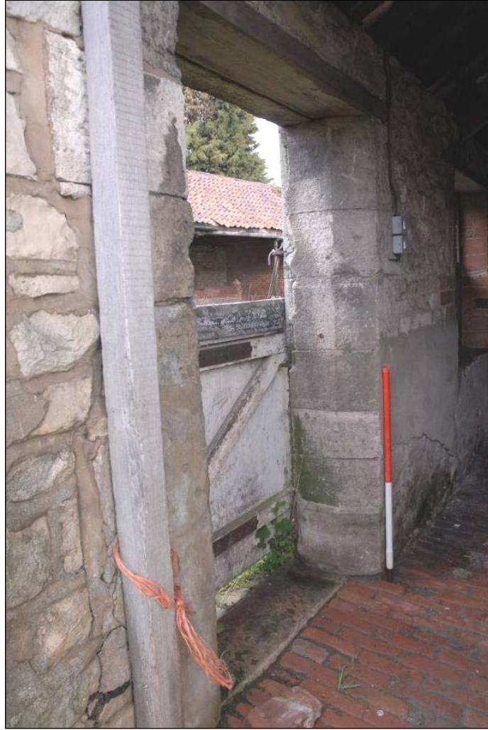
Stable door opening showing chamfered edge
