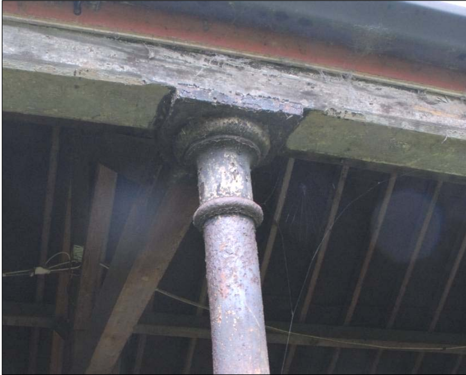
Cast iron capital, Units 3, 4 and 6
