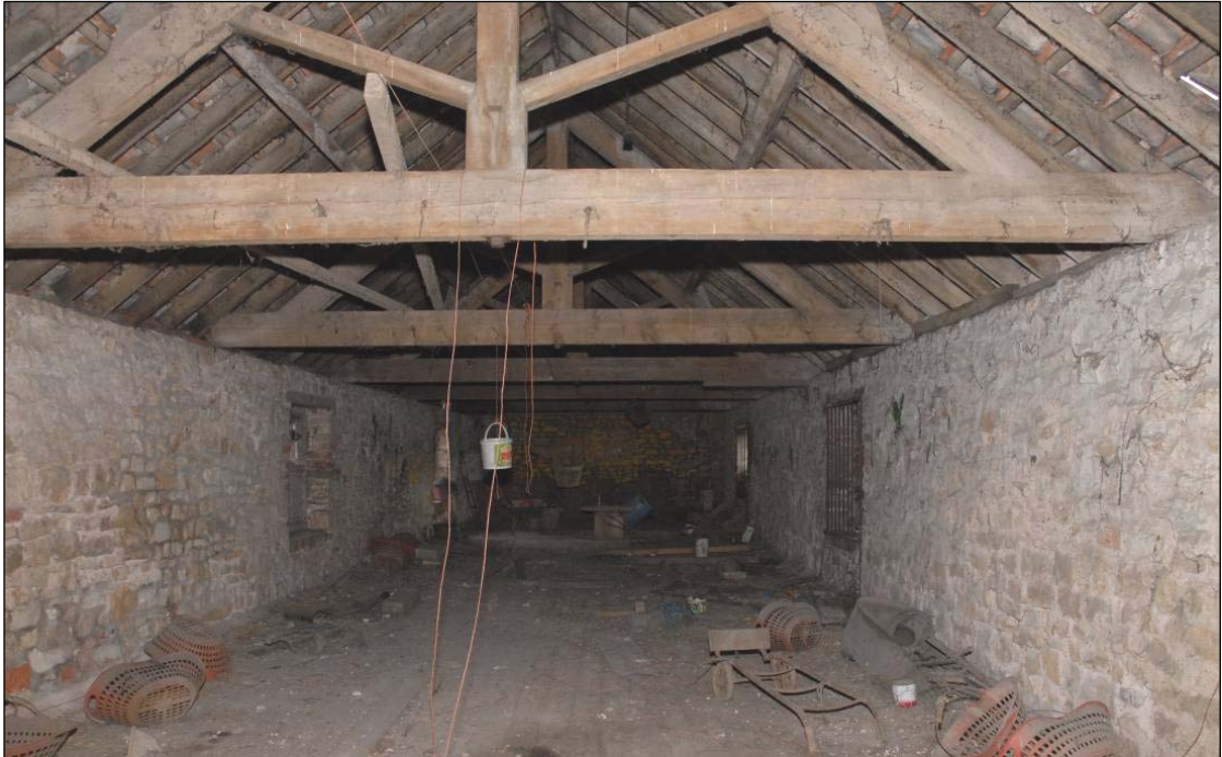
Unit 7, loft space
