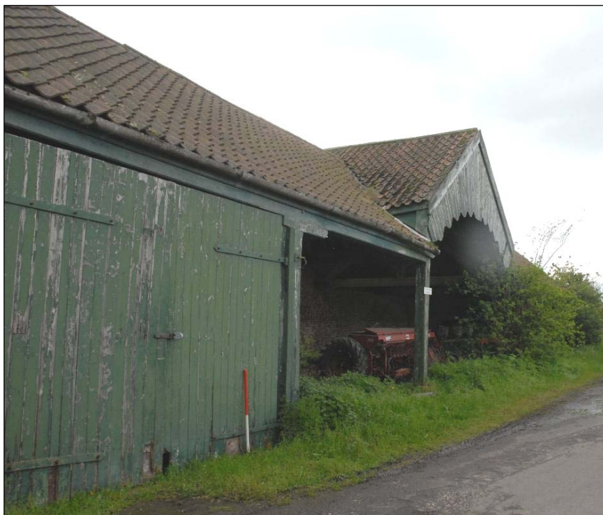
Unit 1, north-western elevation, looking south
