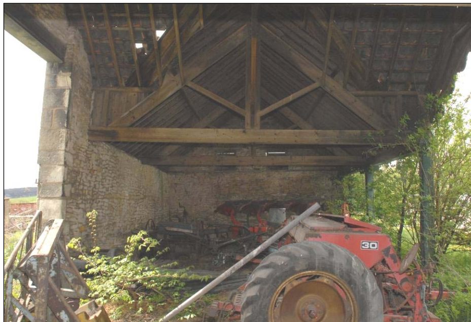
Interior of Unit 1 showing the kingpost truss
