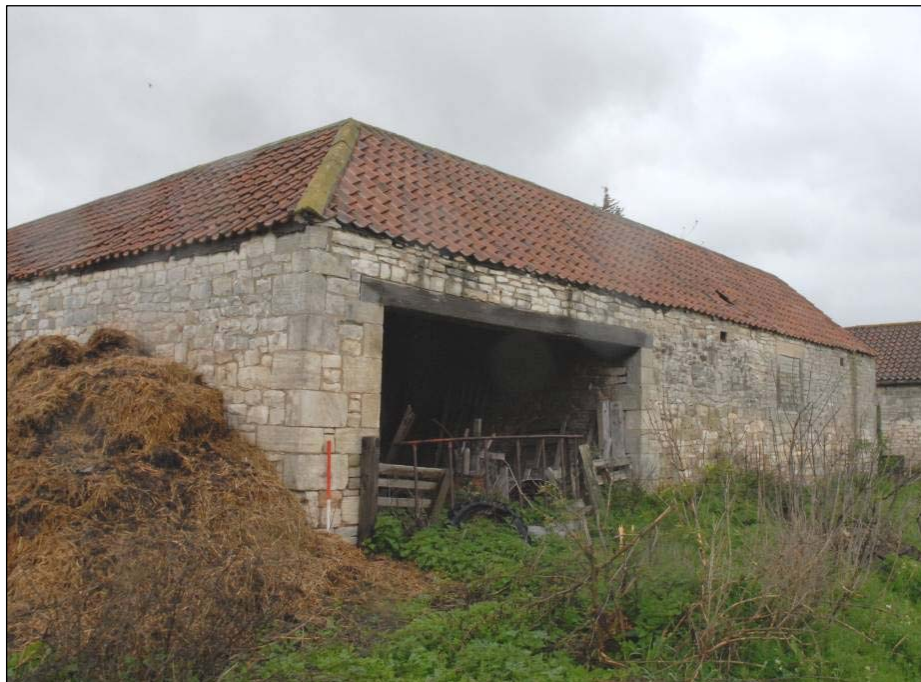
Unit 4, cart shed
