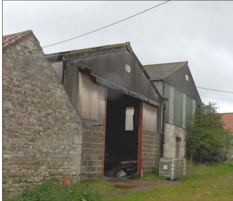
Unit 2, modern barn
