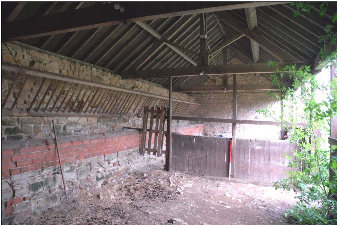
Interior of Unit 3
