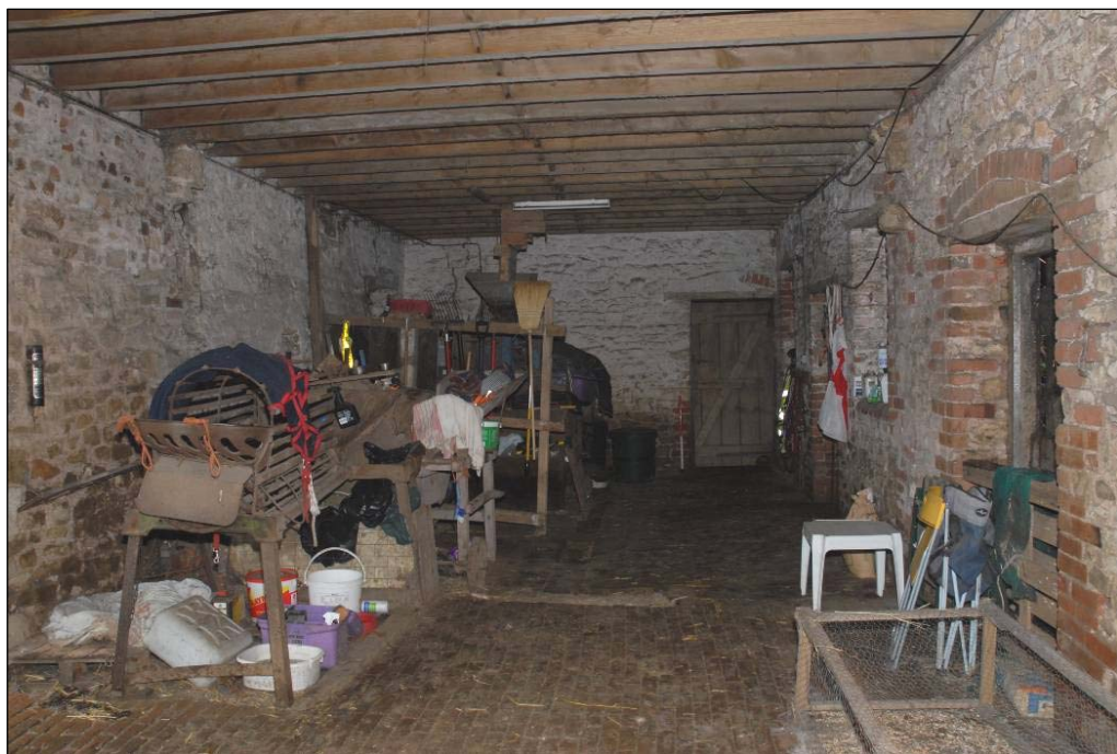
Unit 7, ground floor looking north-west
