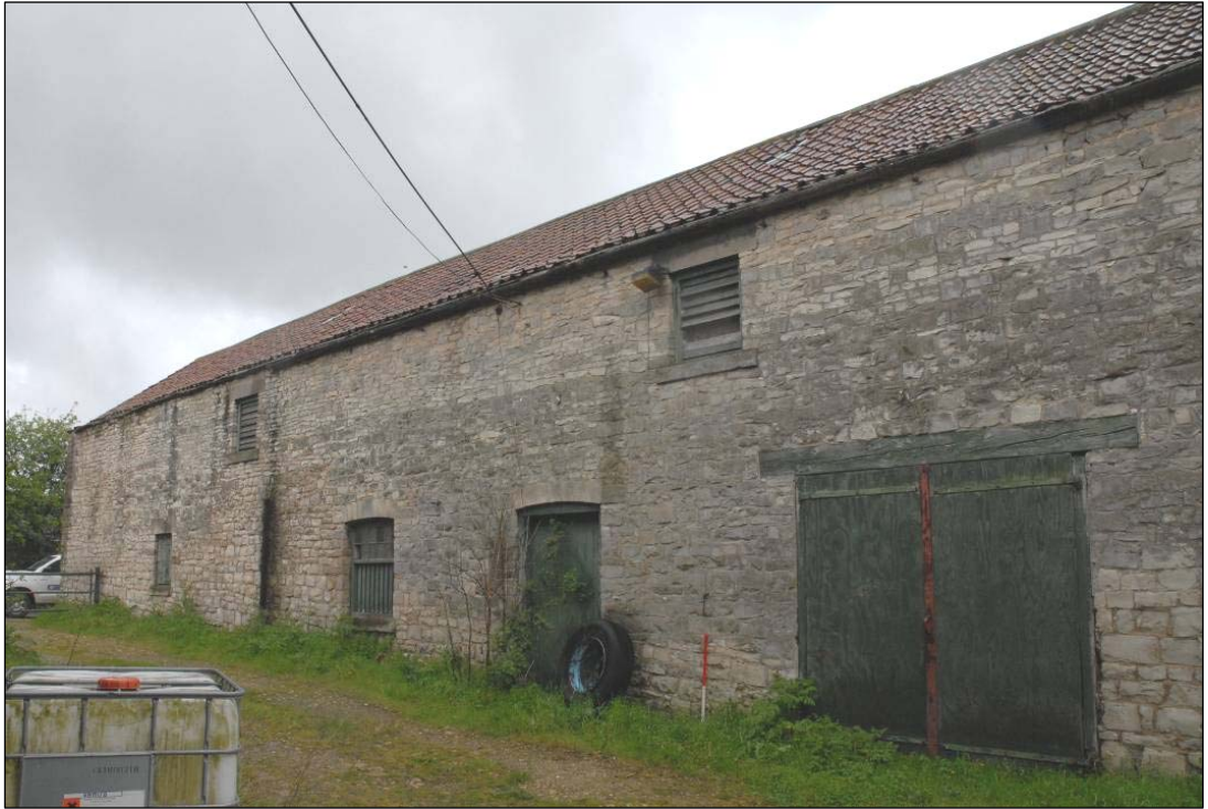
Unit 8, barn and stable
