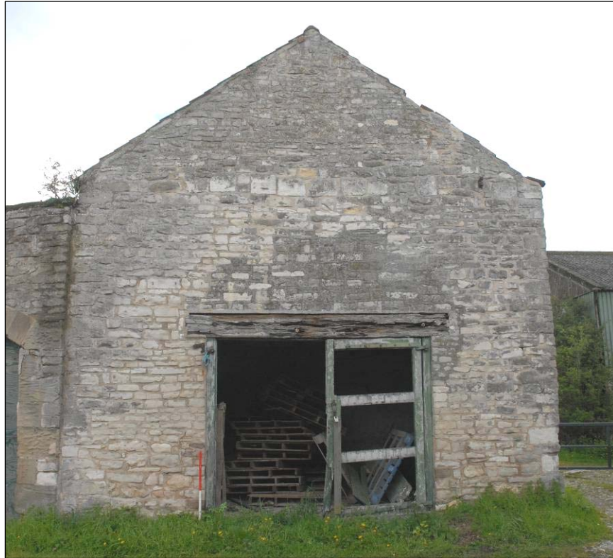
Unit 8, cart shed
