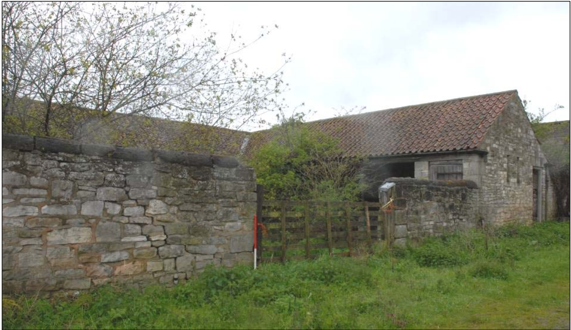
Unit 4 showing enclosed yard
