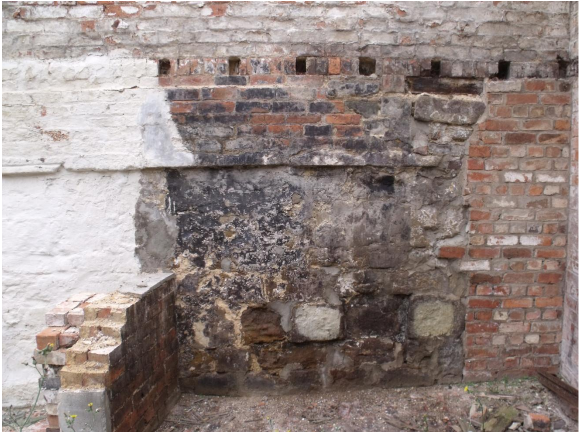
The rear wall of demolished ancillary buildings, looking east Fig 19
