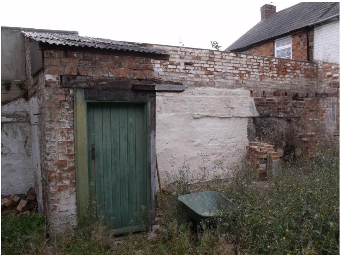
Lavatory building, looking east Fig 20
