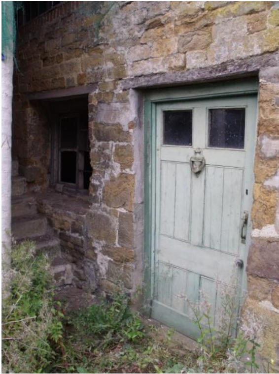
Second extension door Fig 16
