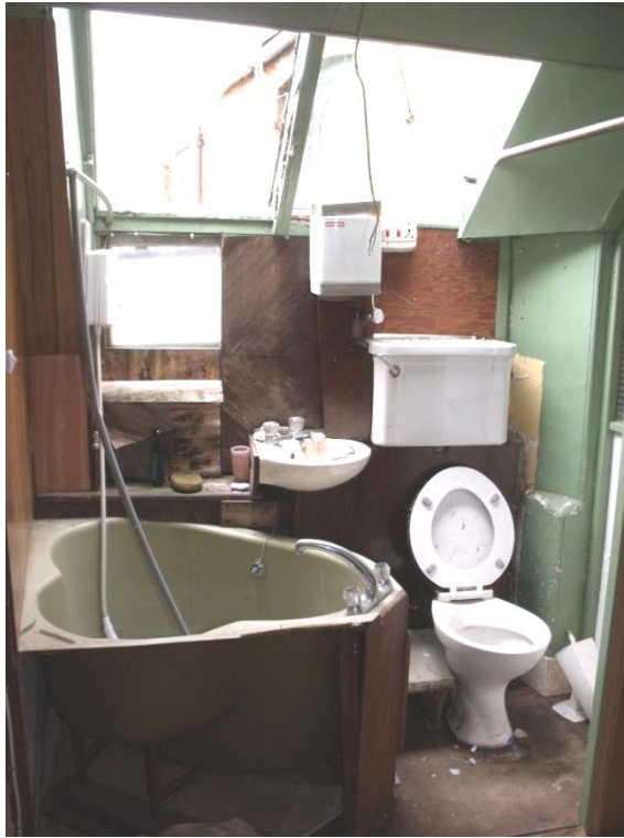
Room F5, looking south Fig 27
