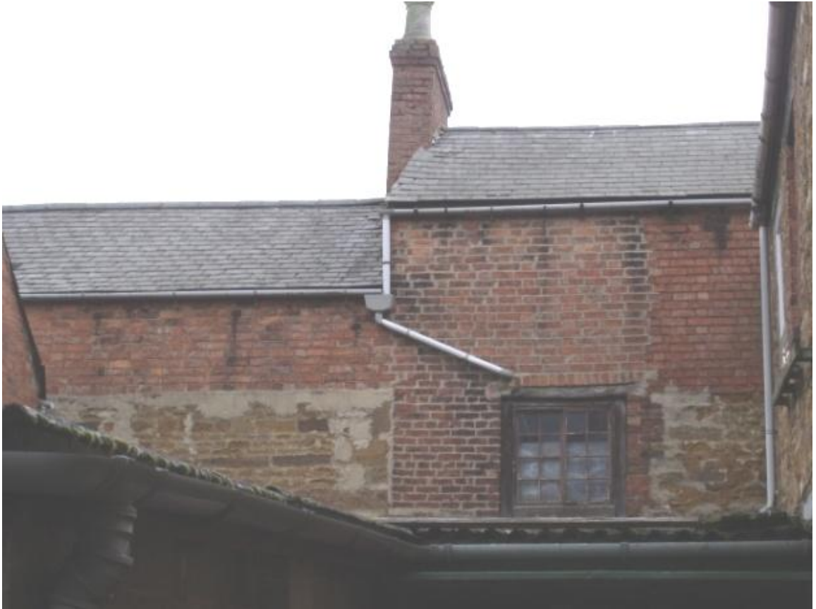
Rear extension of Vine House from the west side Fig 14
