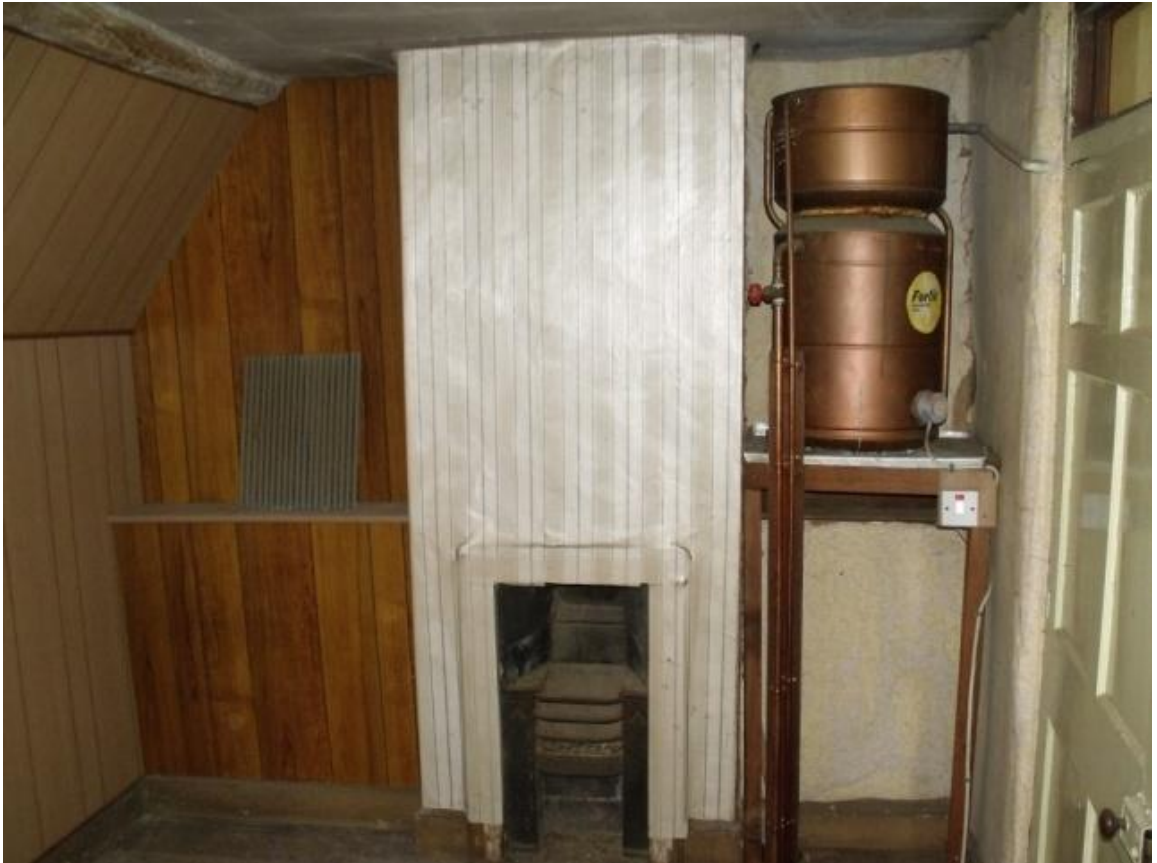
Room F6, looking east Fig 29
