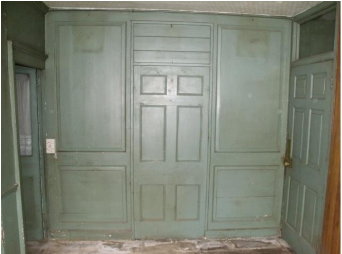
Room G7, looking south Fig 21
