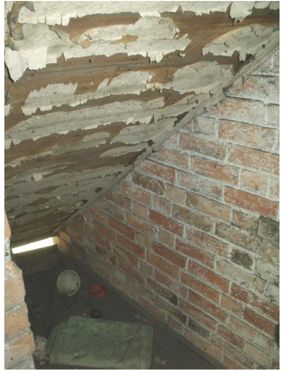
Room S3, looking north-east Fig 45
