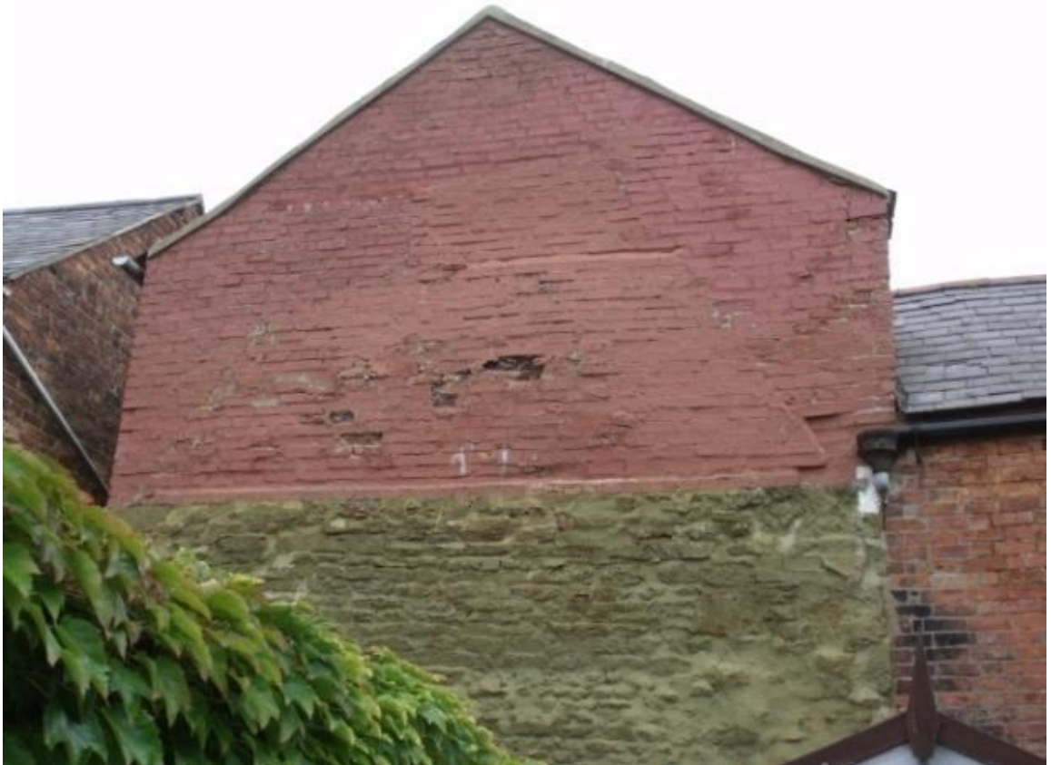
Rear extension of Vine House, south gable Fig 15
