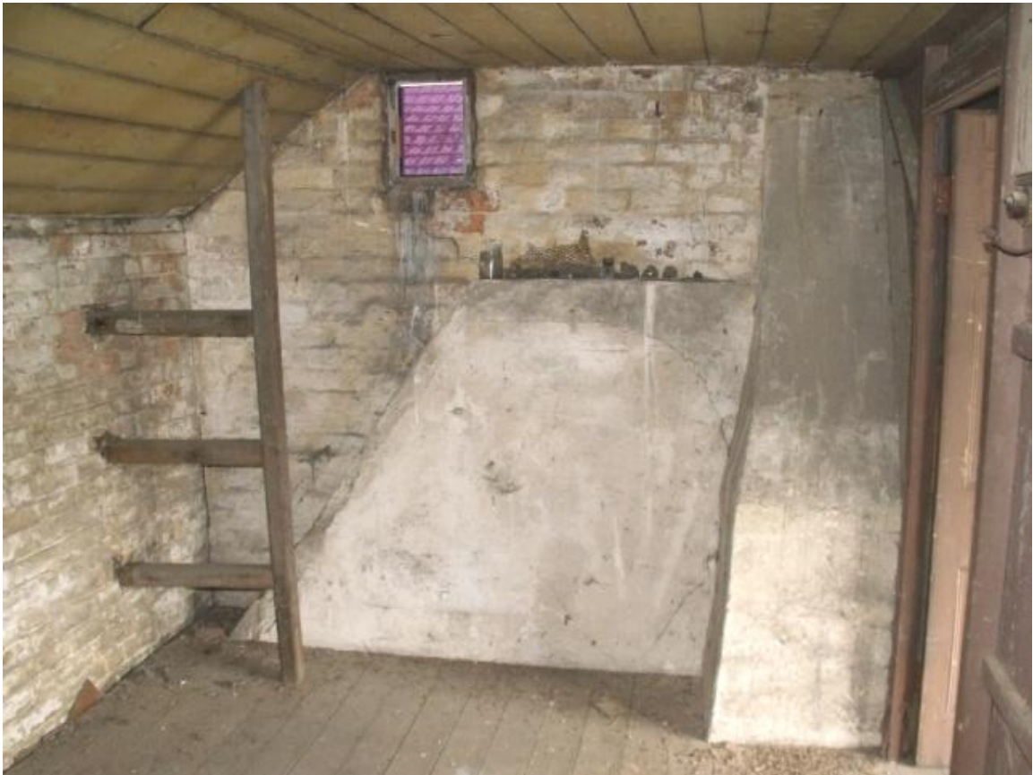
Room S1, looking north Fig 44
