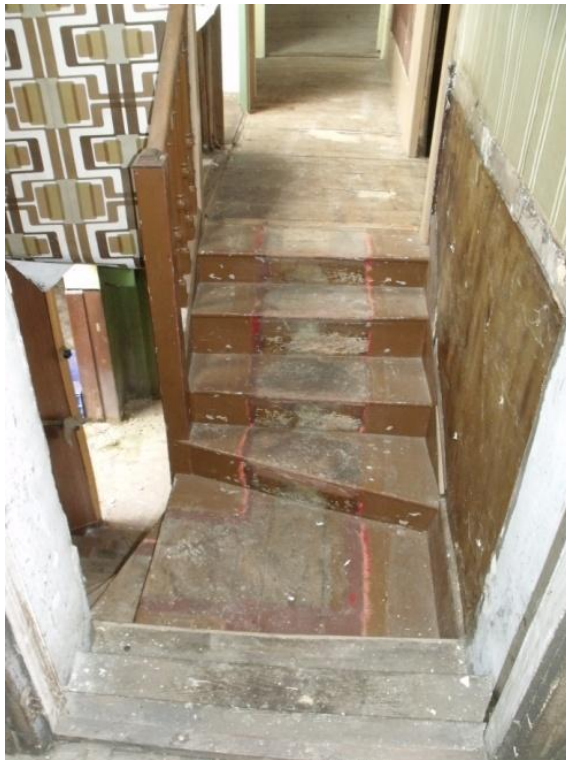
Stair G6, looking west Fig 25
