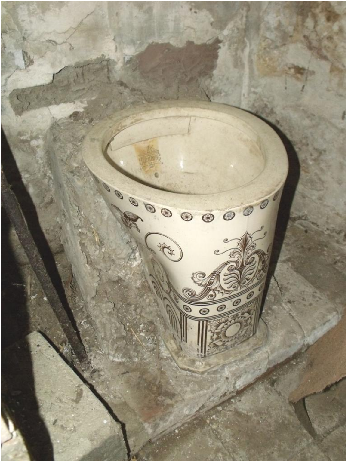
Room G13, toilet Fig 47
