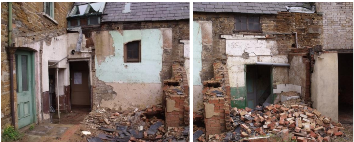
Rear of frontage after demolition of modern extensions Figs 9-10
