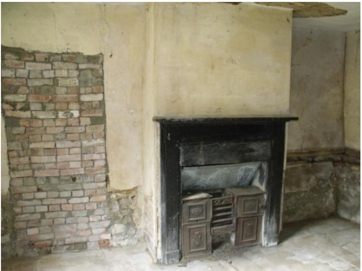
Room G9, looking south Fig 36
