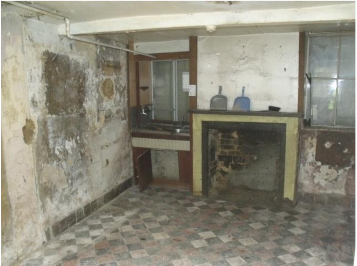
Room G5, looking south-west Fig 35
