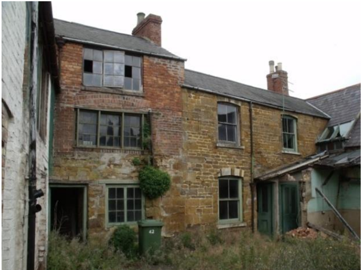
Rear extension of Vine House, looking west Fig 13
