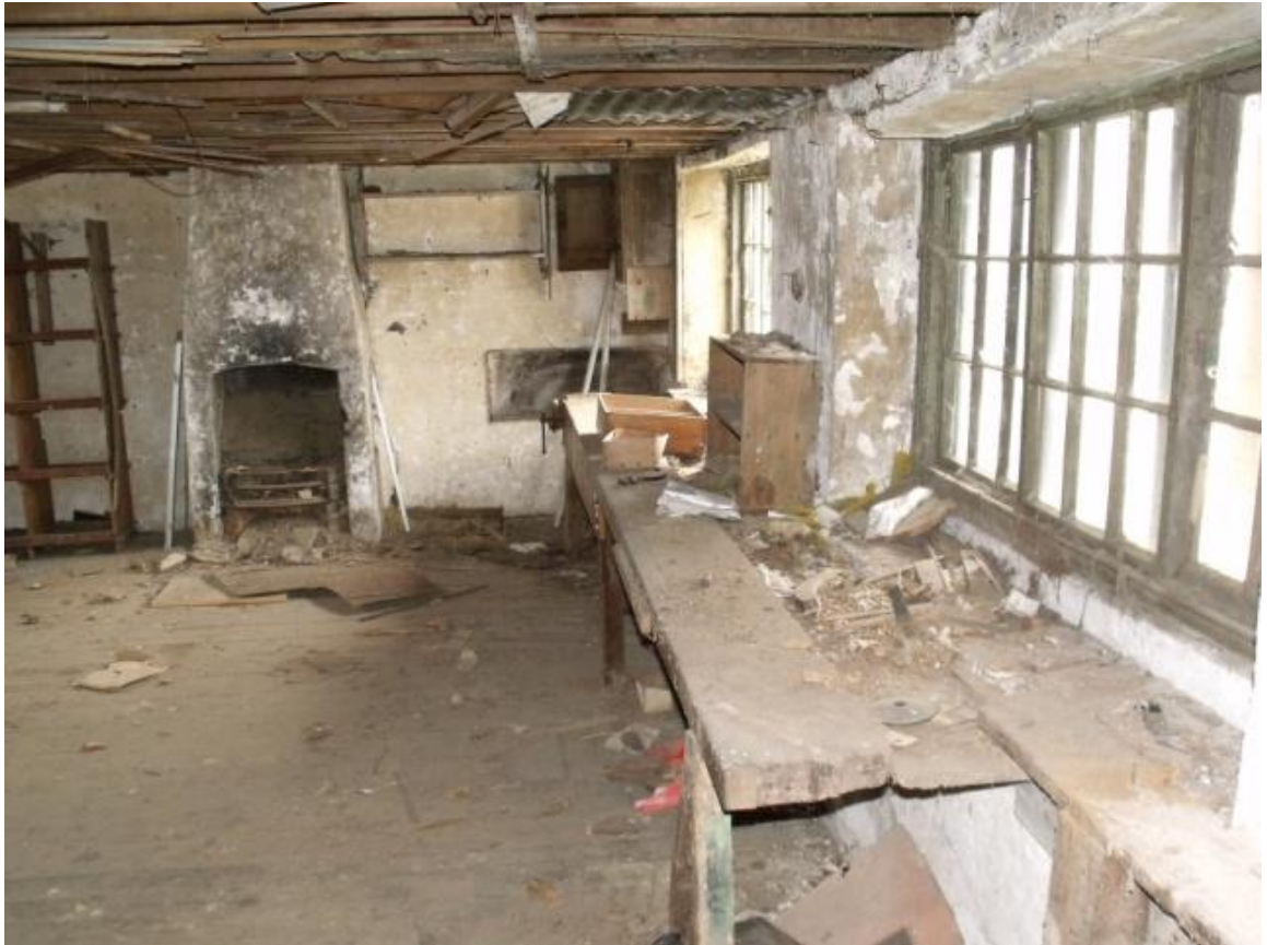
Room F11, looking north Fig 42
