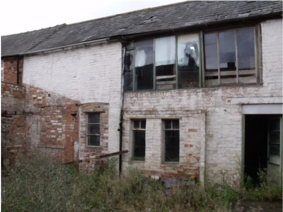
Carpentry workshop, looking south Fig 18
