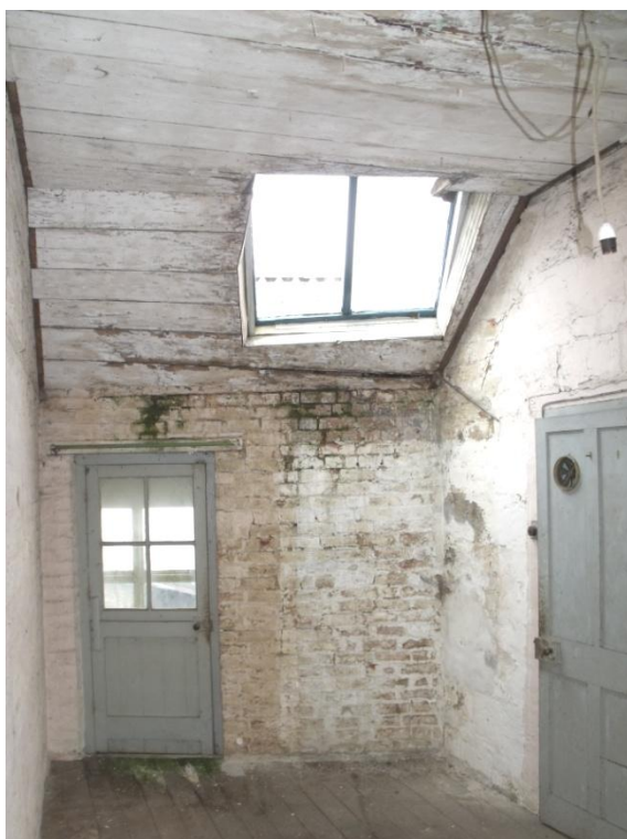
Room F2, looking south Fig 49
