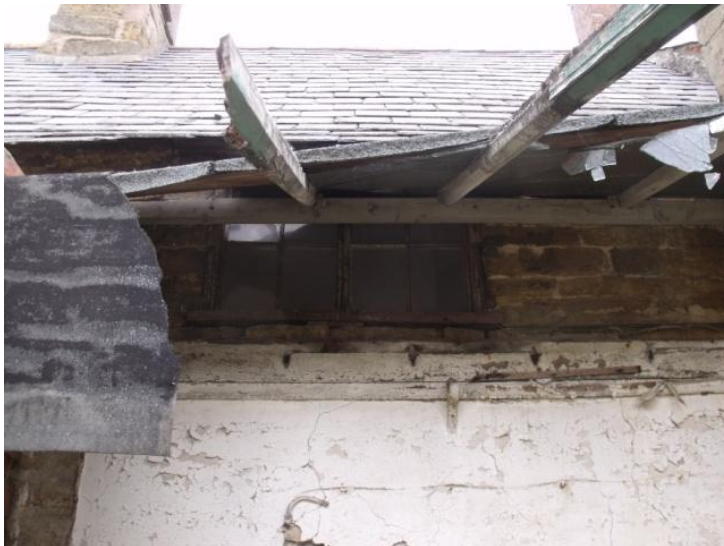
Room G3, roof Fig 51
