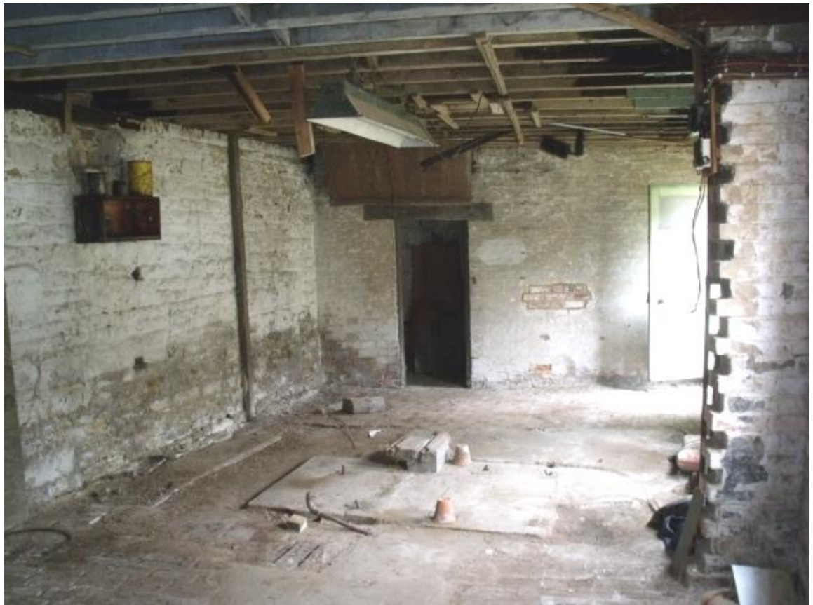
Room G13, looking west Fig 46
