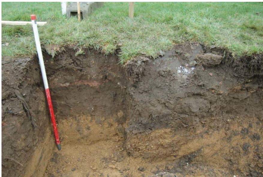
Levelling layer [7] under topsoil at the north-west corner of the foundation Fig 7
