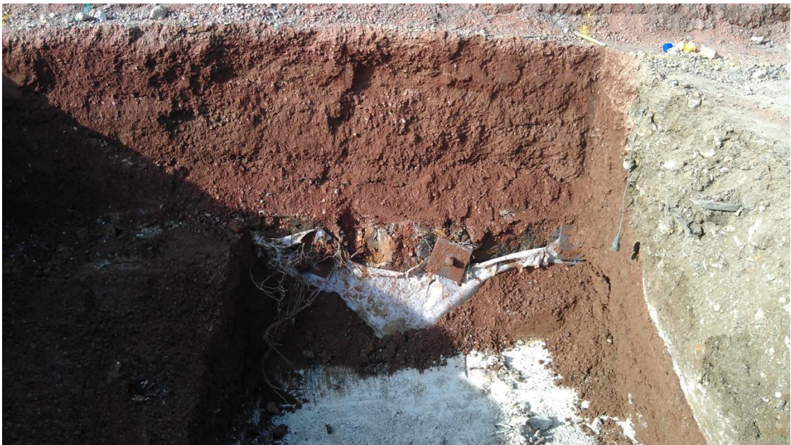
Layers above the chalk within the vortex separator trench, looking west Fig 4
