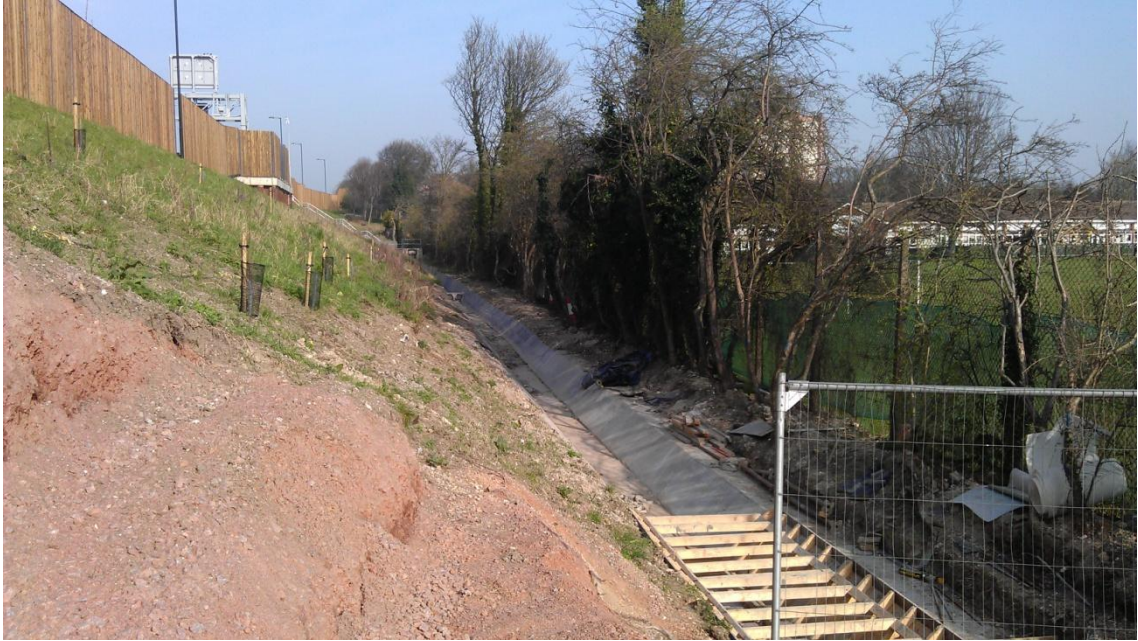
Drainage ditch, cleaned and concreted, looking north Fig 3
