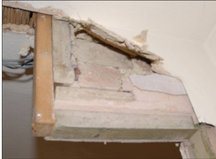
Room F2, Detail of surviving brick on edge construction Fig 18
