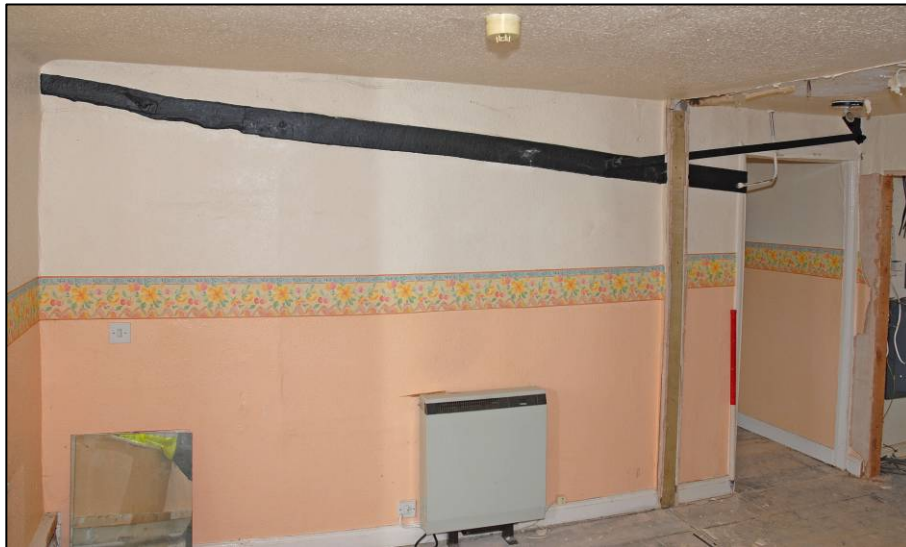
Room S10, repaired tie beam
