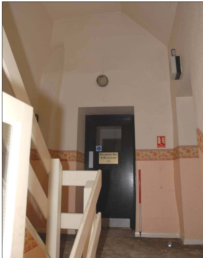
Modern stair inserted into Room F4
