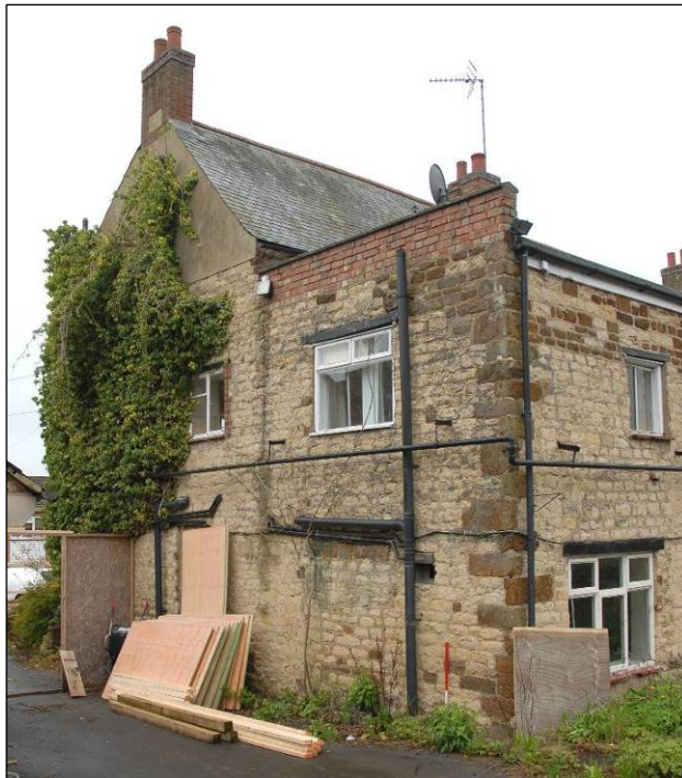
The extension to the rear of the former Gate Inn Fig 14
