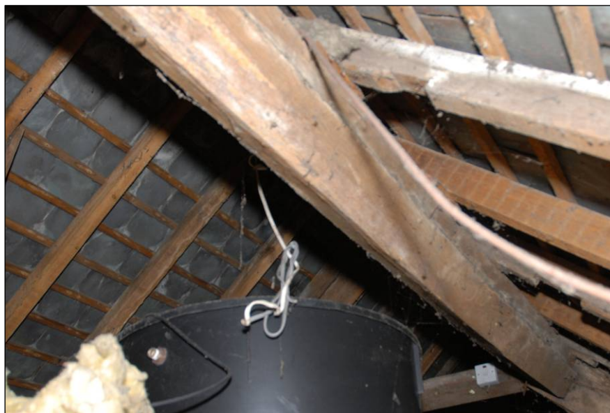
Roof structure above Room S10
