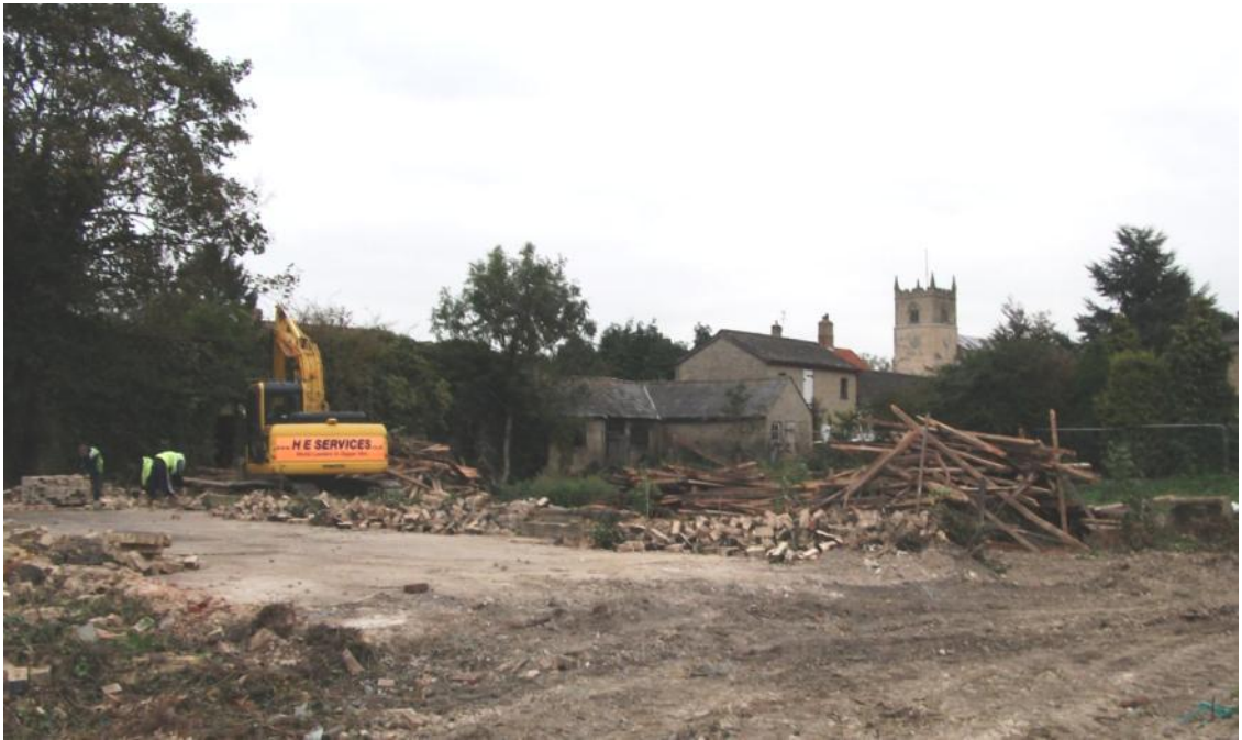
Demolition and clearance, looking north-east Fig 23
