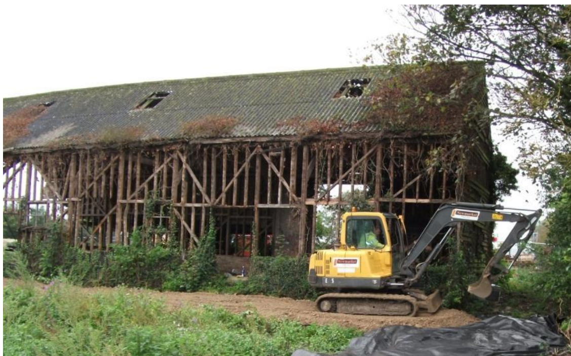
The 19th-century timber-framed barn, looking west Fig 20
