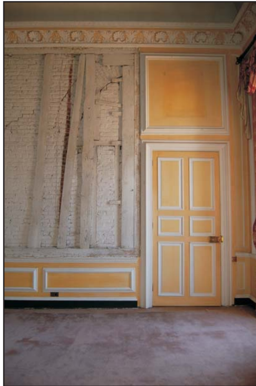
South wall of Master Bedroom Three showing the location of the arch to the left (east) of the door and the frame of the former tapestry, looking south
