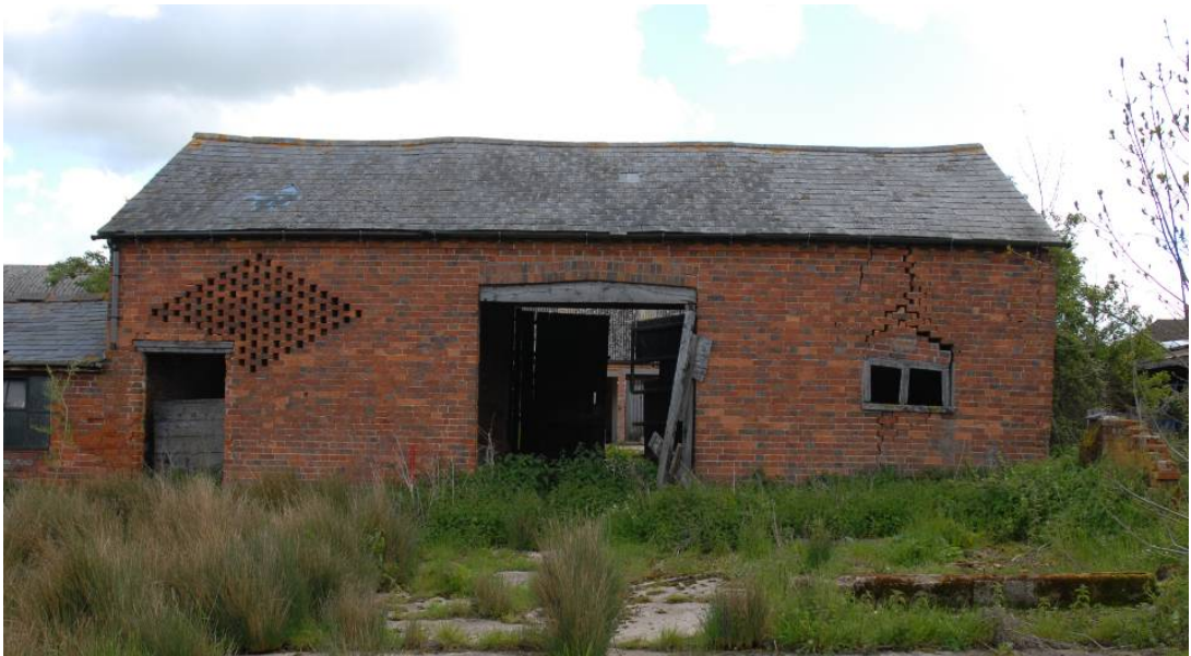
Building 5, looking east
