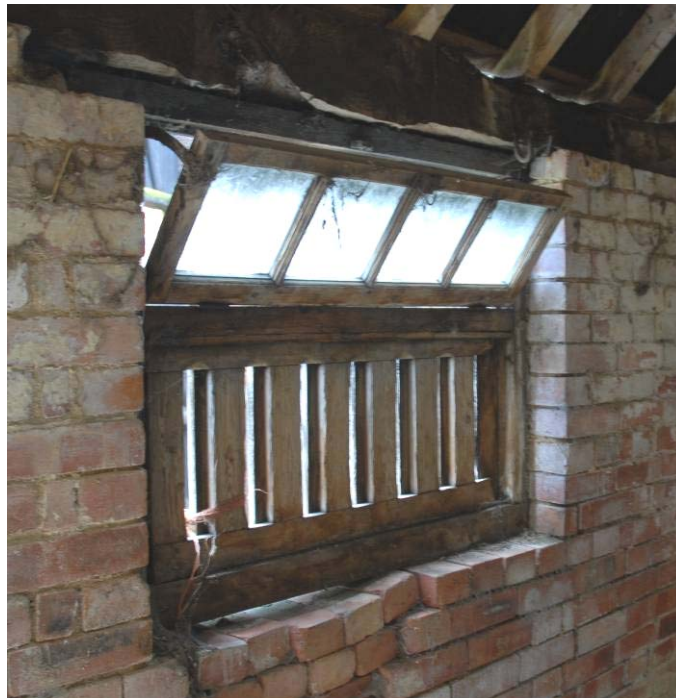
Building 10, horizontal sliding hit-and-miss ventilator window
