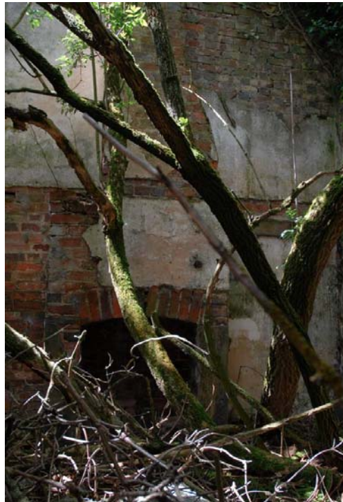
Fireplace and chimney breast, Building 7, looking west
