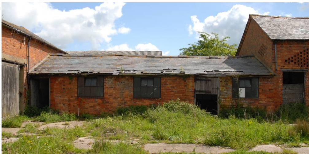
Building 4, looking east
