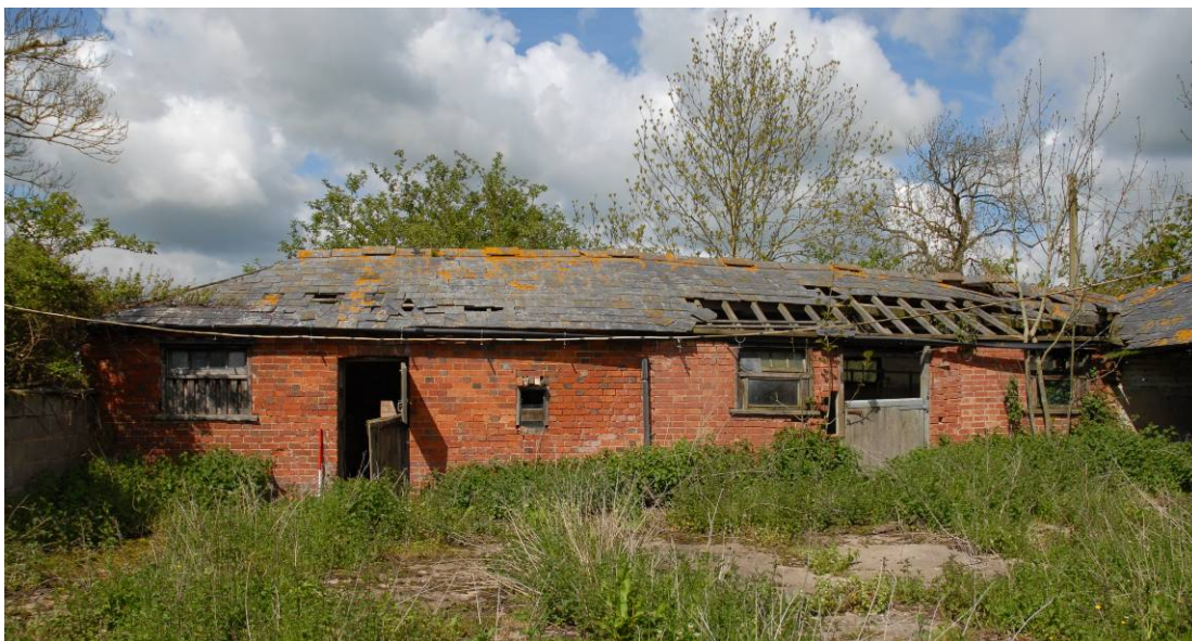
Building 1, looking west
