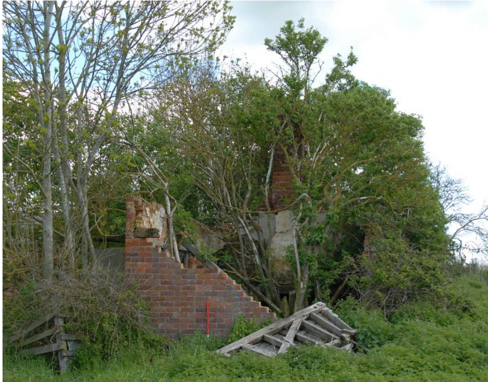
Building 6, looking north-east
