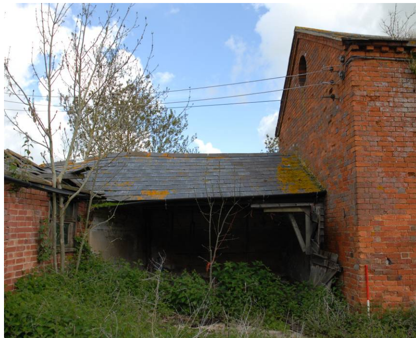
Building 2, open cattle shelter shed, looking north
