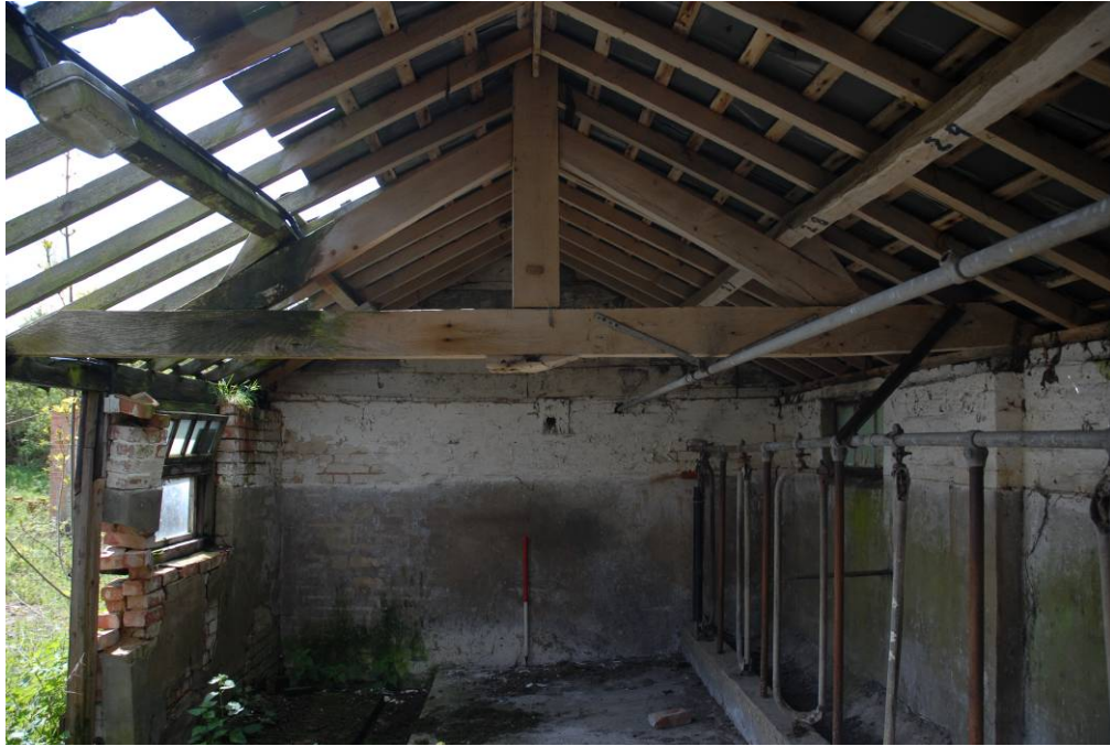
Interior of Building 1 showing the kingpost truss
