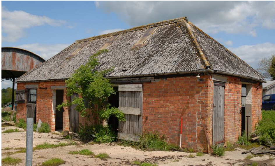
Building 9, looking north-east
