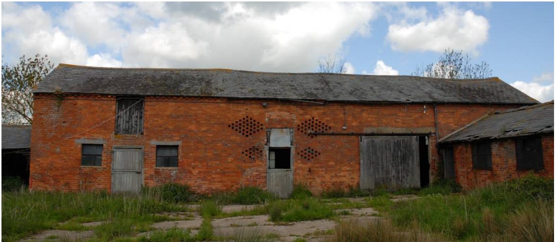
Building 3, looking north
