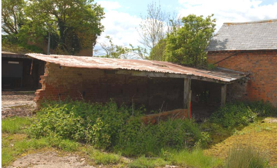
Building 11, looking south-west
