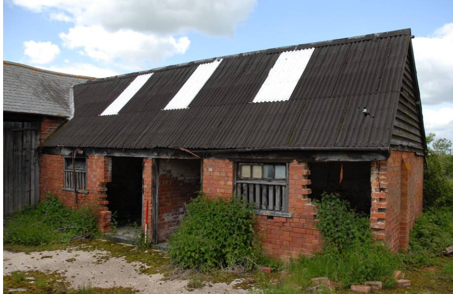
Building 10, looking north-west
