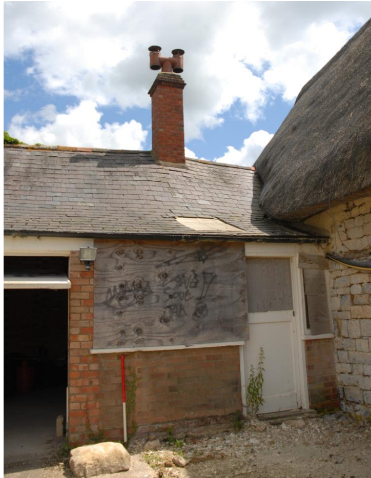
The chimney and modern lobby area
