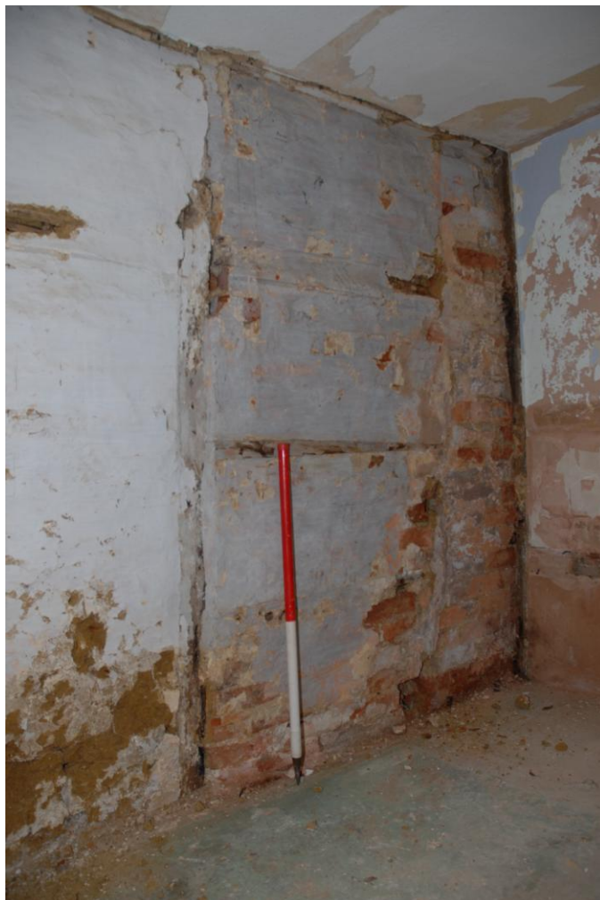
The internal partition wall
