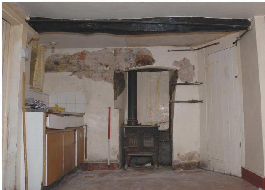
The fireplace opening for the chimney in the kitchen
