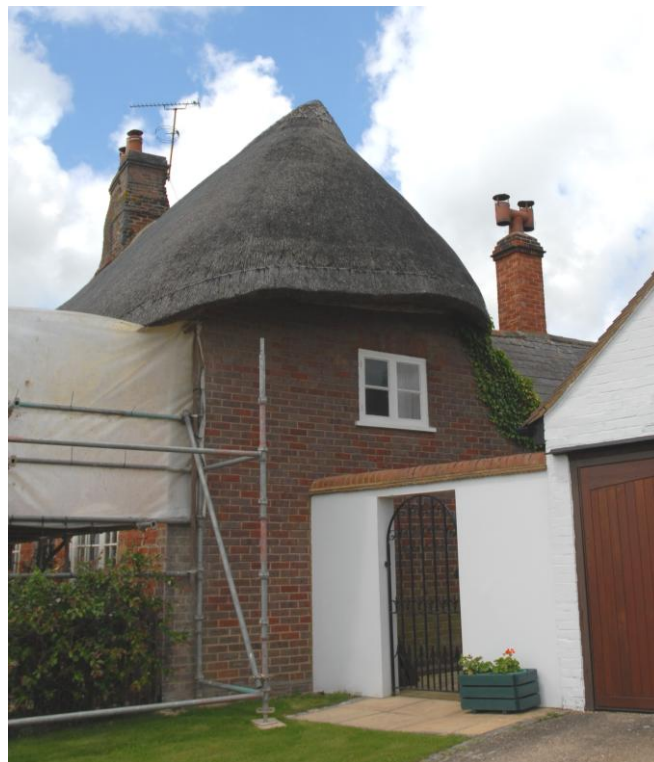
The eastern gable end
