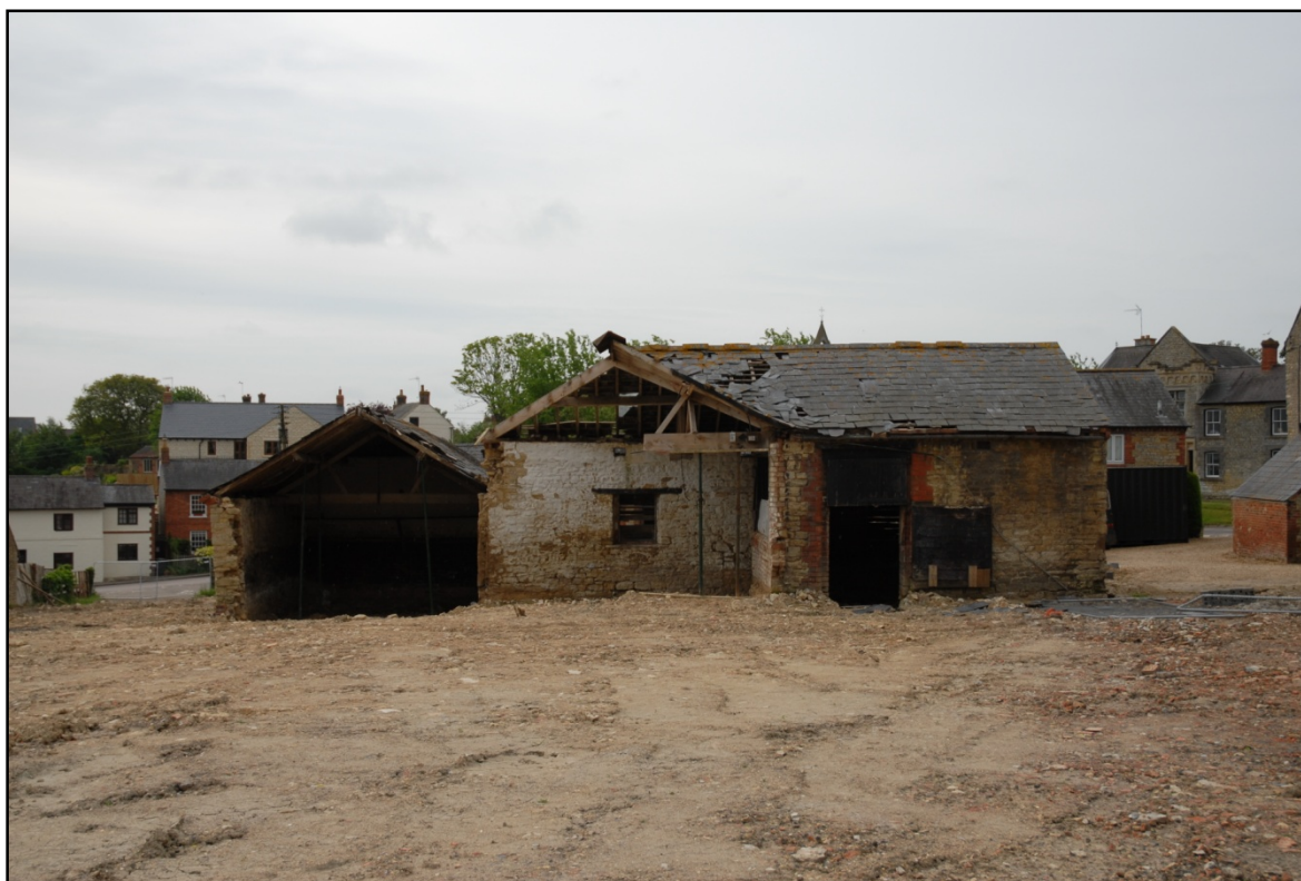
The northern elevations of buildings B3 and B2, looking south-east Fig 11
