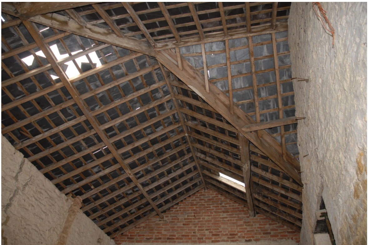
The roof structure above room G2 Fig 23
