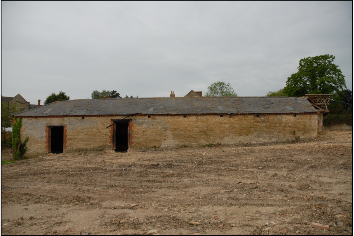
The eastern elevation of buildings B2 and B1, looking south-west Fig 12
