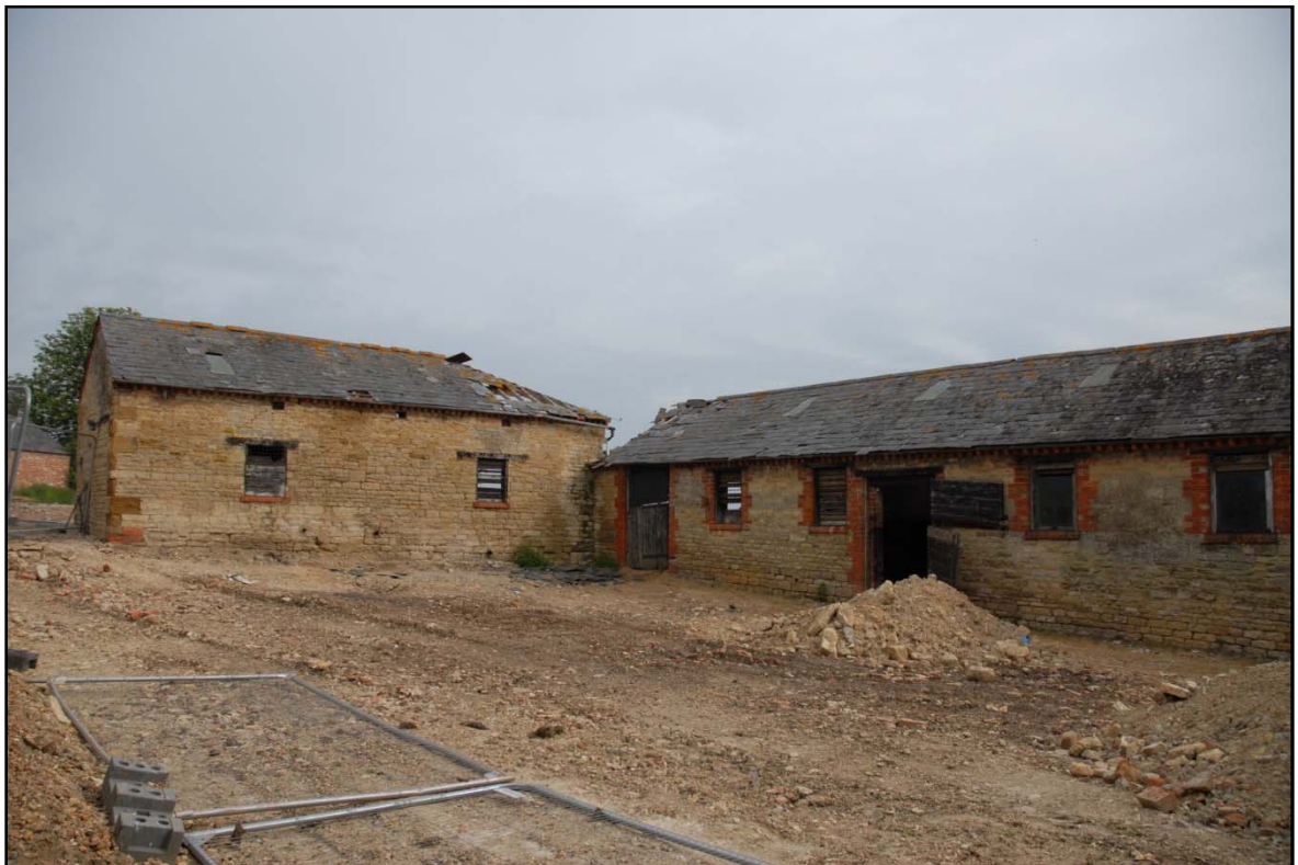
Buildings B2 and B3, looking north Fig 9
