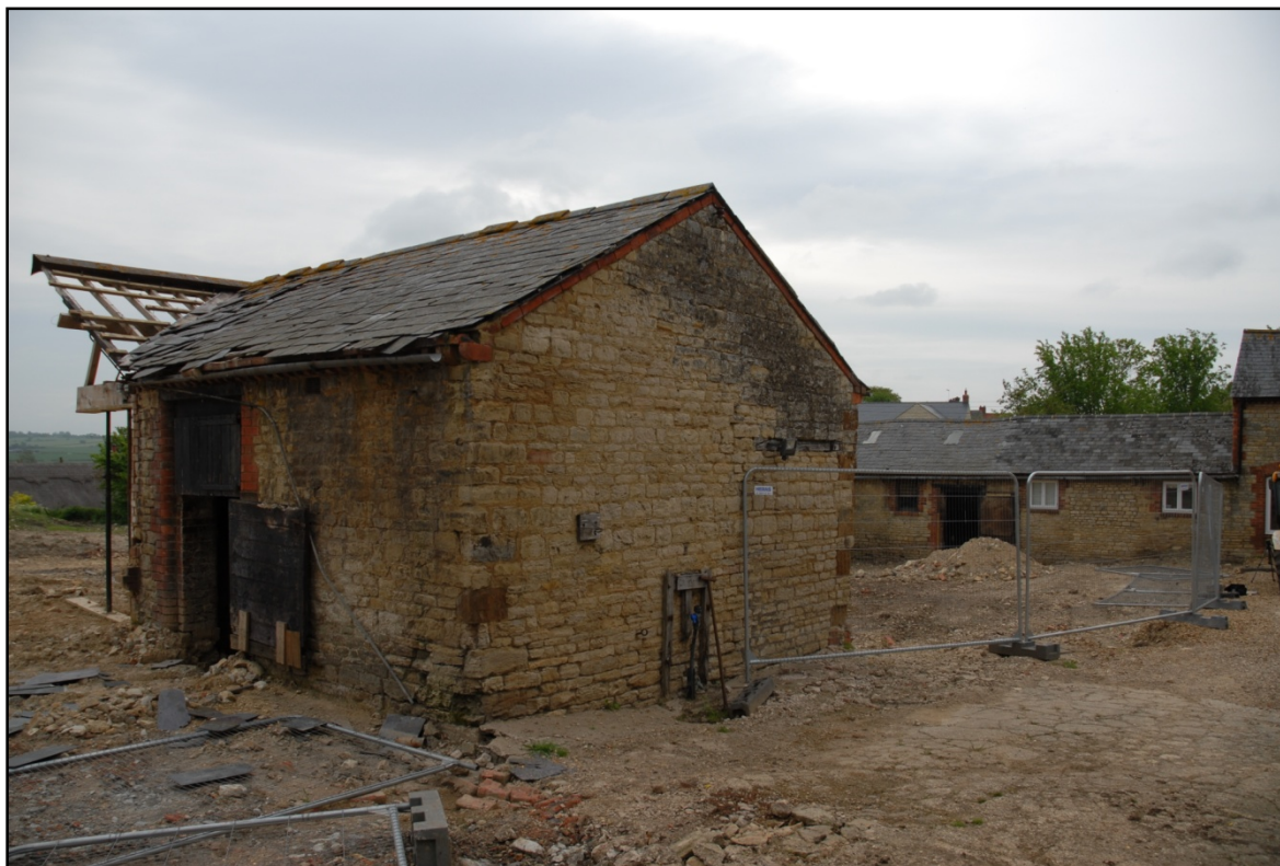
The western elevation of building B3 with sandstone quoins visible to the right, looking east Fig 10
