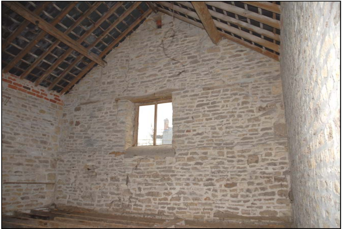
Room F2, the western elevation Fig 26
