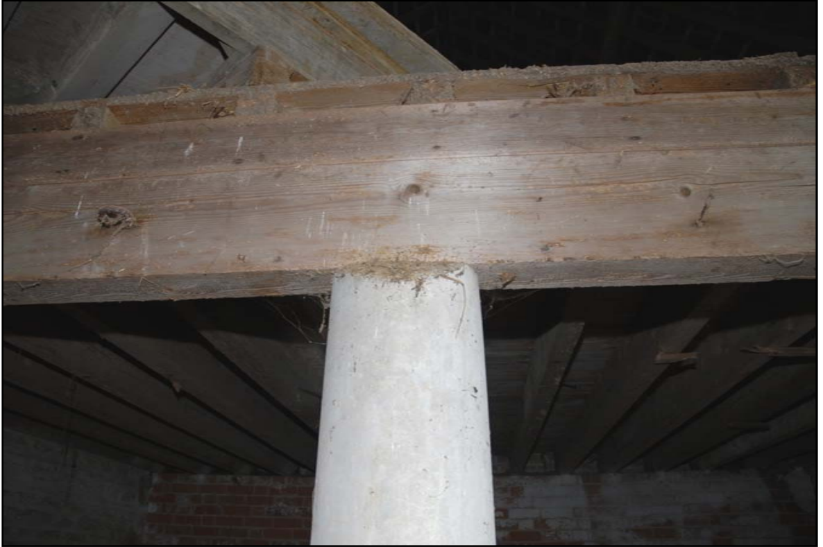
The top of the column Fig 14
