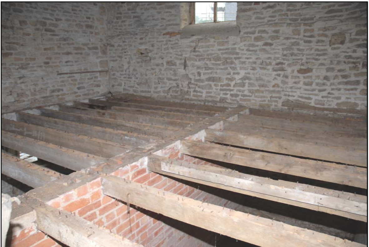
The brick partition supporting joists above rooms G2 and G3 Fig 19
