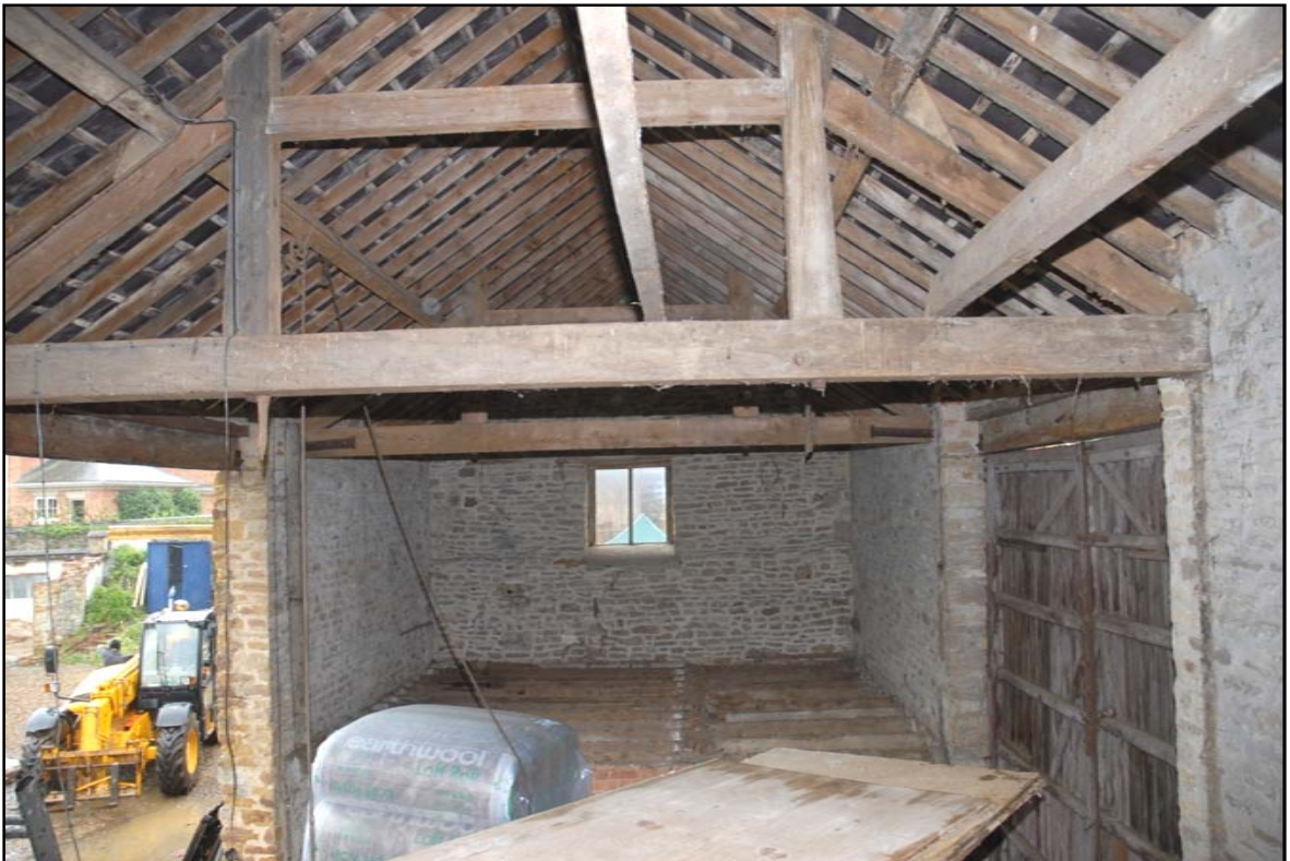
View across the barn into F2, looking west Fig 25
