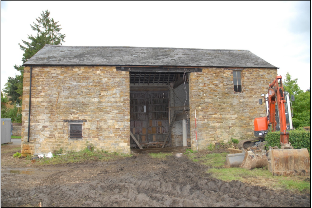
The southern elevation, looking north Fig 6
