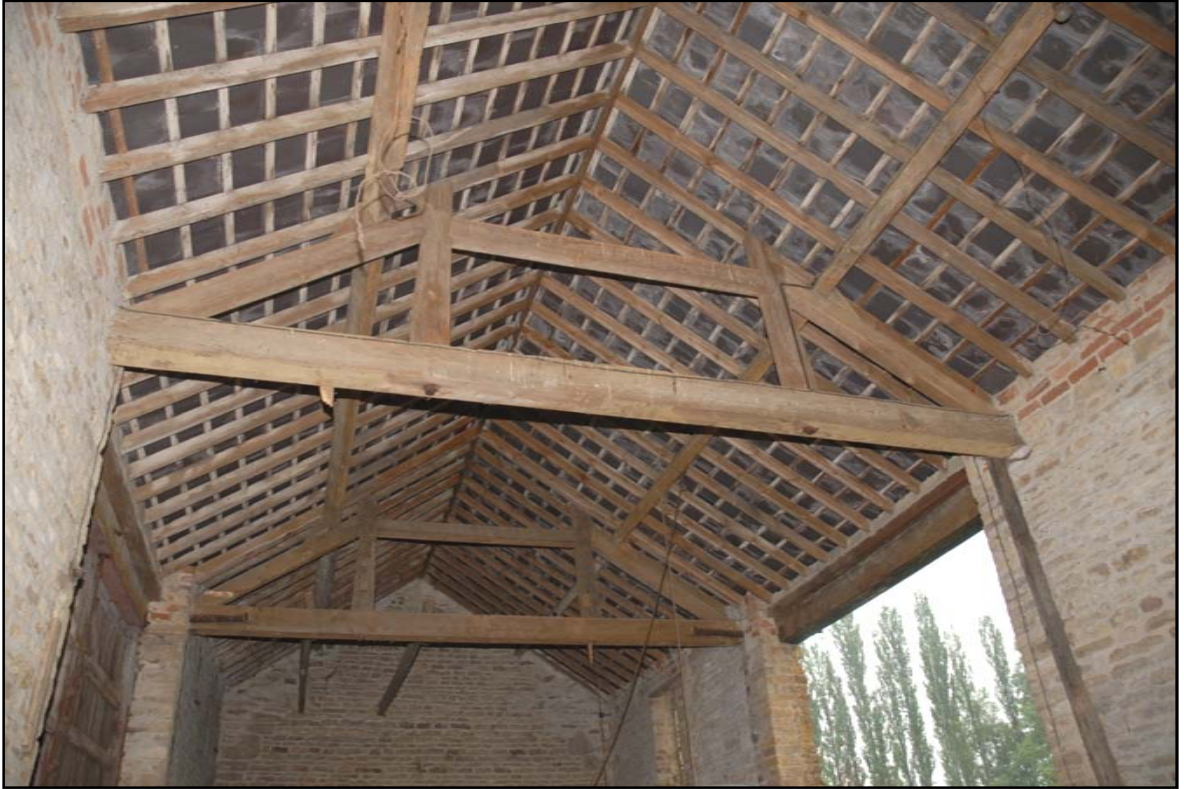
The roof structure, looking east Fig 22
