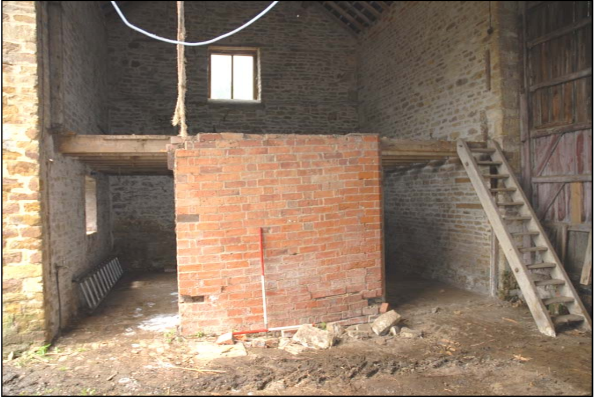
Rooms G2 and G3 with brick partition, looking west Fig 16
