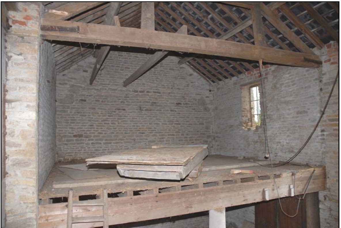
Room F1, looking east Fig 23
