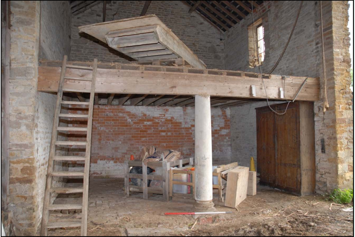
Room G1, looking east Fig 12
