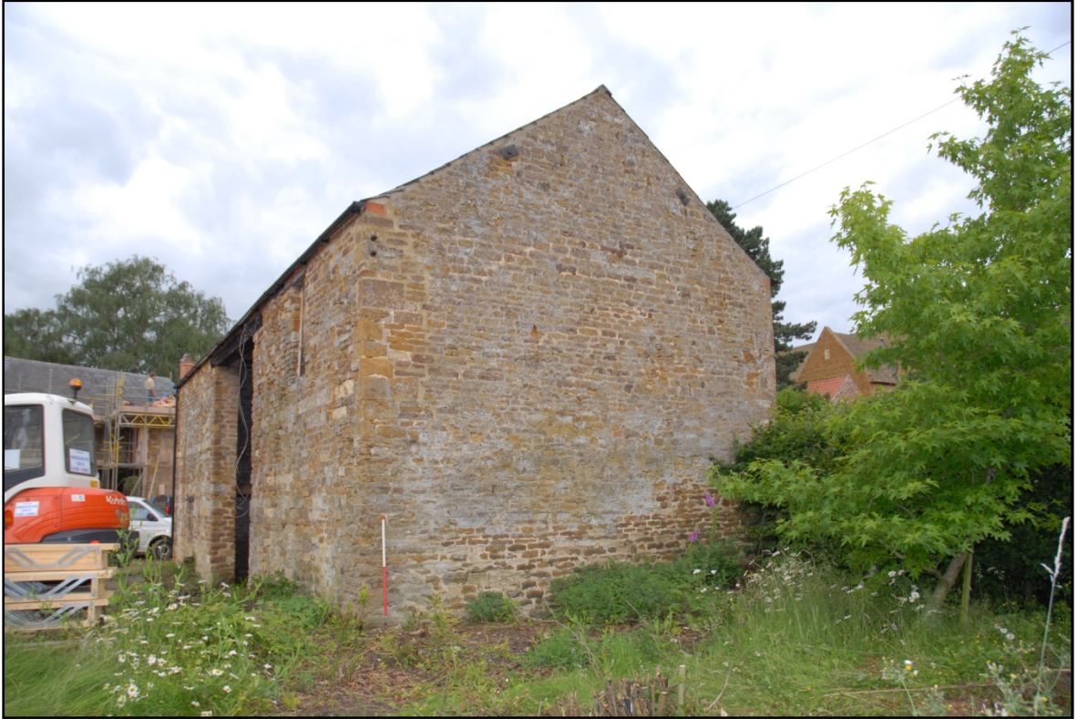
The eastern elevation, looking west Fig 8
