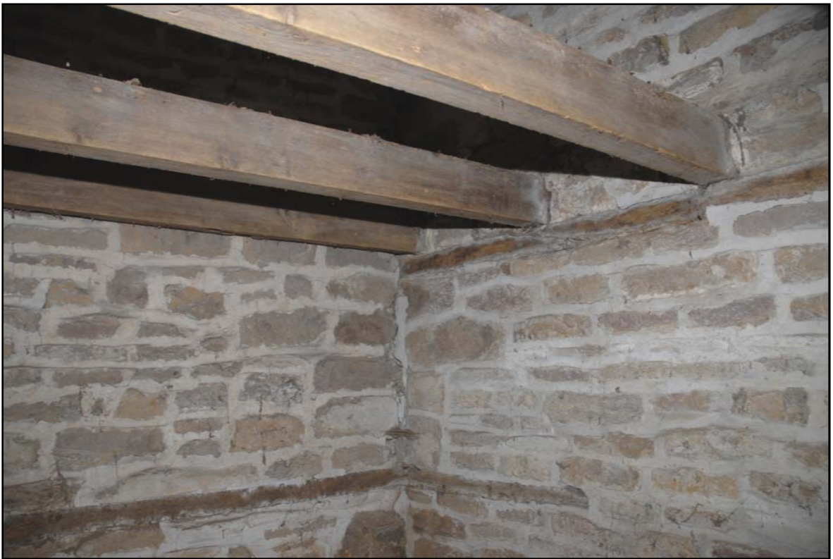
Room G3 showing joists supported by timber beams Fig 21
