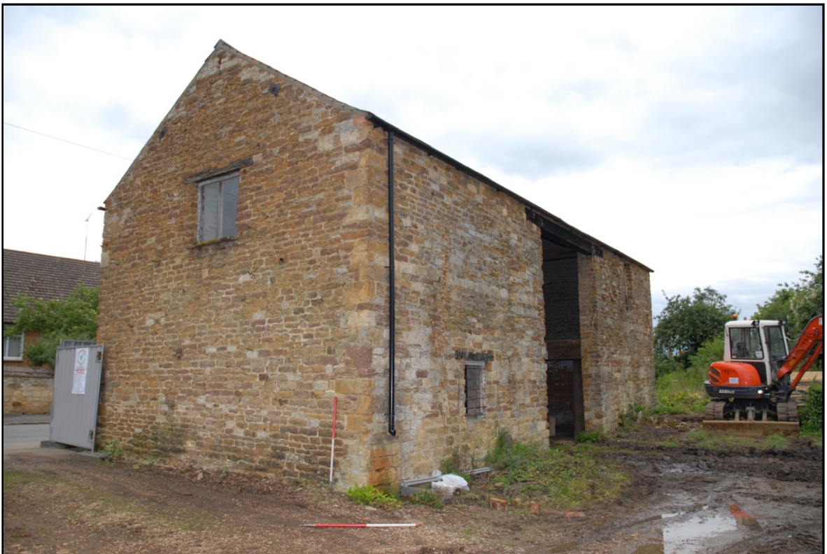
The western elevation, looking north-east Fig 9
