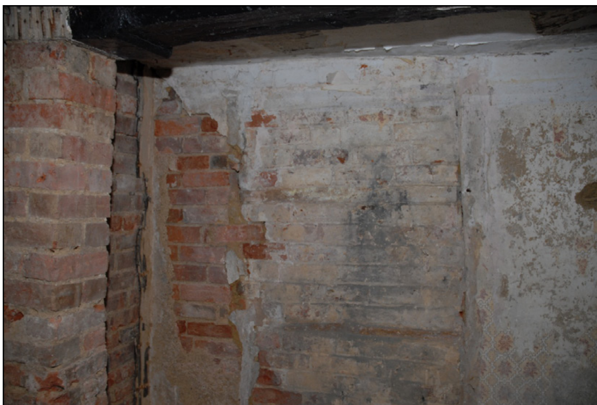
The partition showing the join between the 1842 brickwork and the earlier brick with timber bond Fig 45
