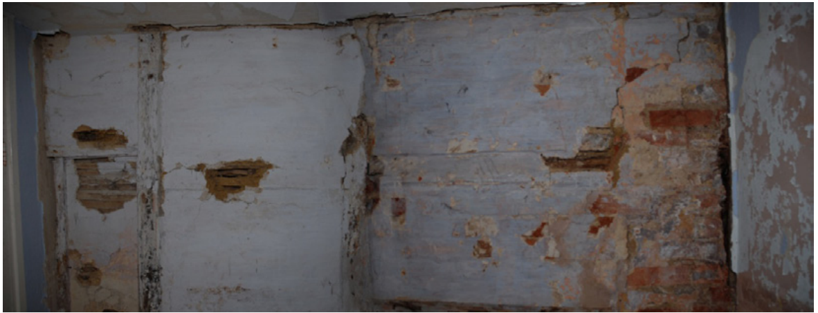
Composite of the east partition within the Bathroom Fig 36
