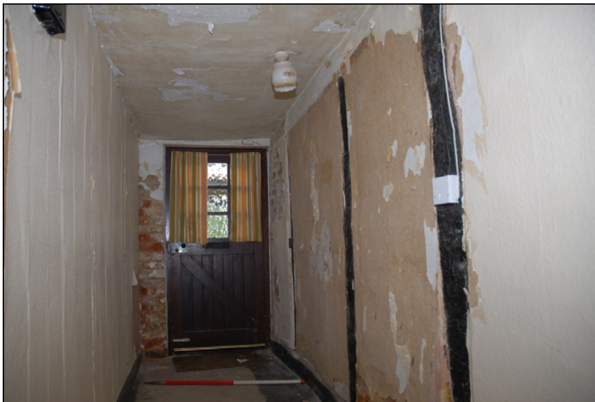
View down the Hall towards the south wall, showing the brick nogging Fig 24
