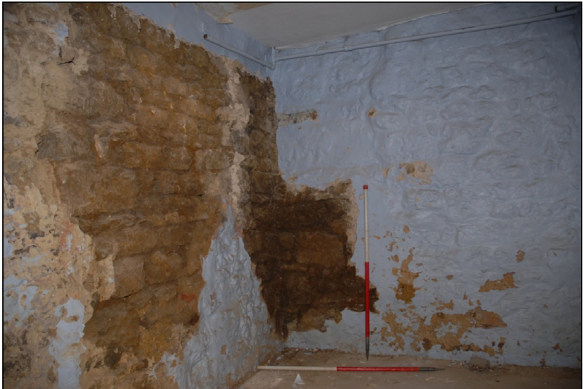
The north and west walls of the Dressing Room Fig 37
