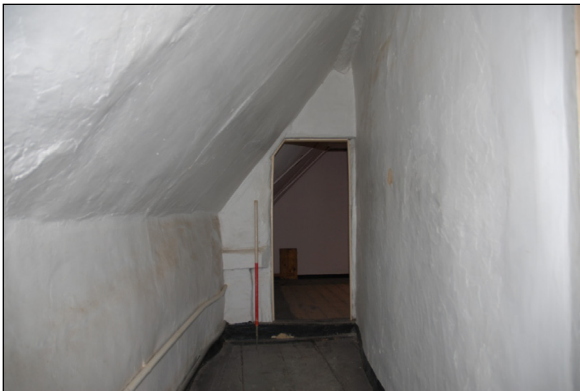
The first floor corridor, looking east Fig 48
