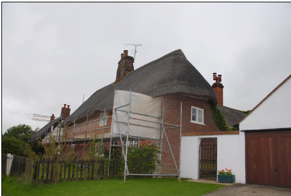
The eastern, brick-built elevation, looking north-west Fig 7
