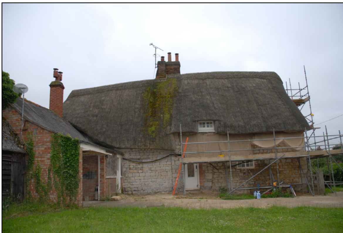
The northern elevation showing central join and change in roof structure Fig 12
