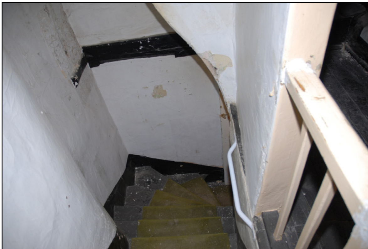
The staircase with chimneys to the left Fig 47
