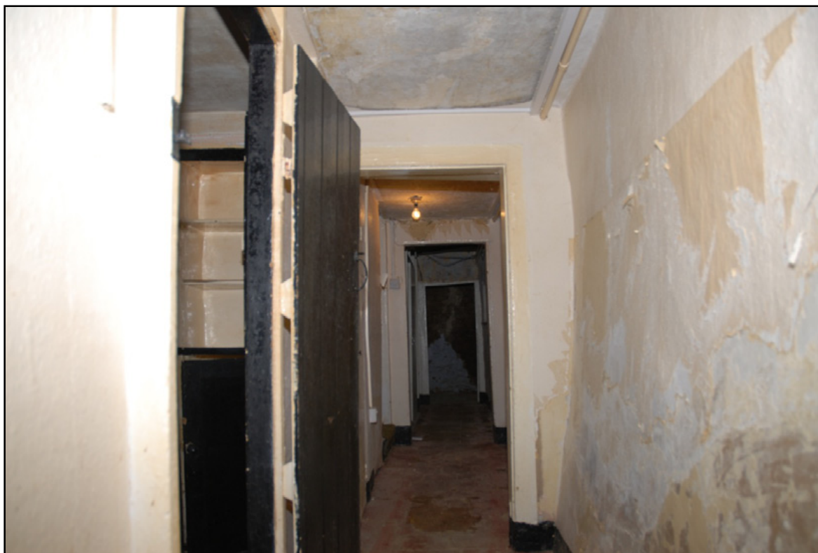
View down the Corridor, looking west Fig 25
