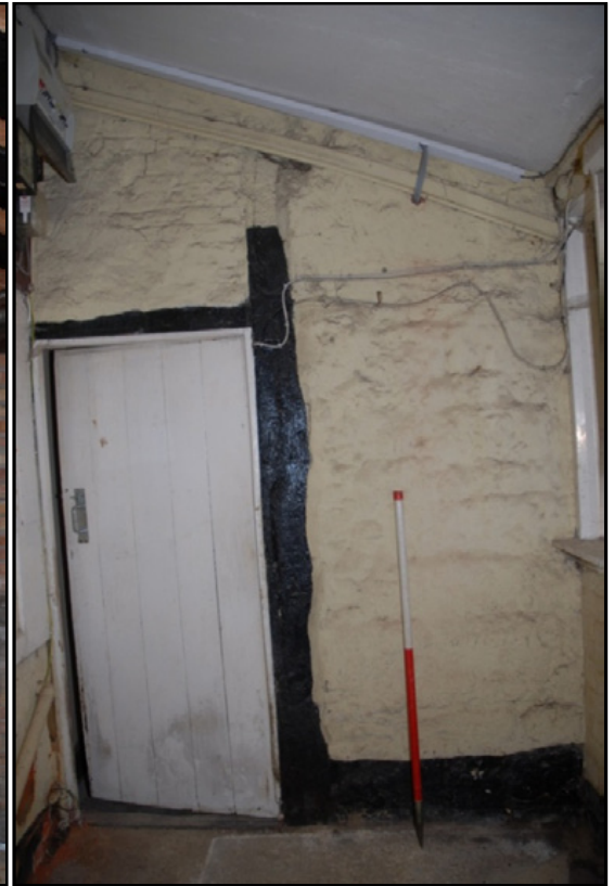
The south wall of the Lobby Fig 19
