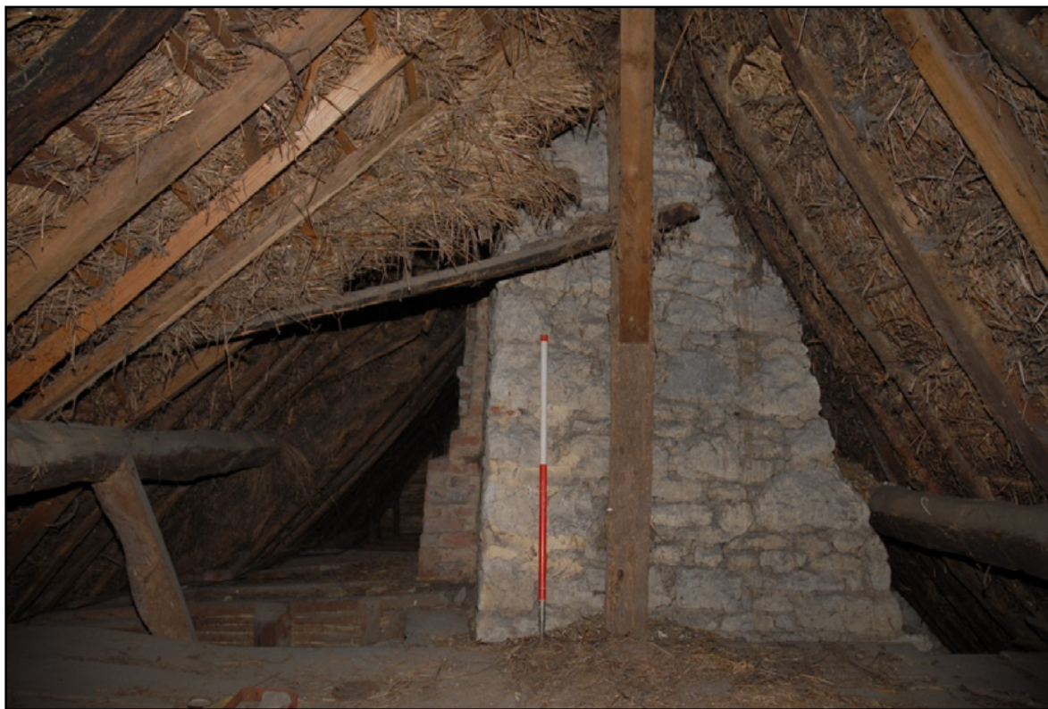
The west face of the central chimneys, looking east Fig 67
