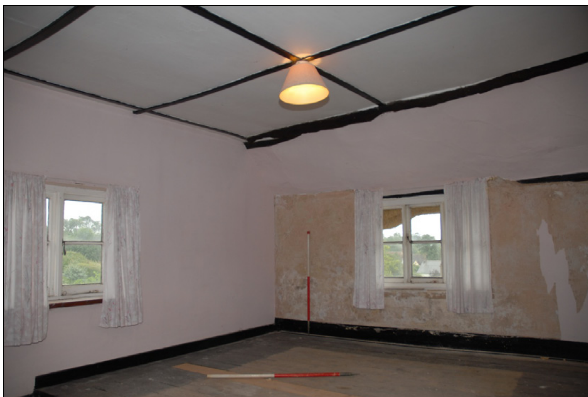
Bedroom 1 showing the timber frame in the ceiling, looking south-east Fig 52
