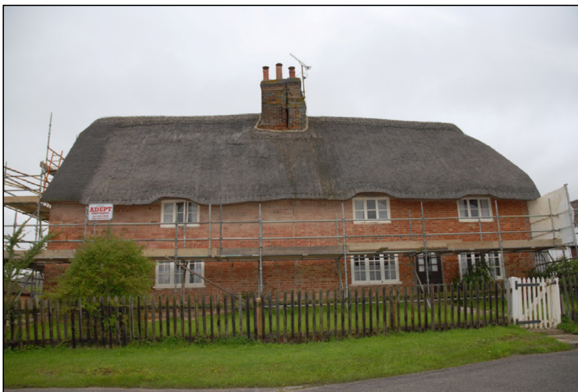
The southern elevation showing the central join Fig 8
