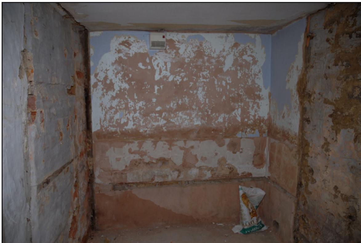
The south wall of the Bathroom Fig 40
