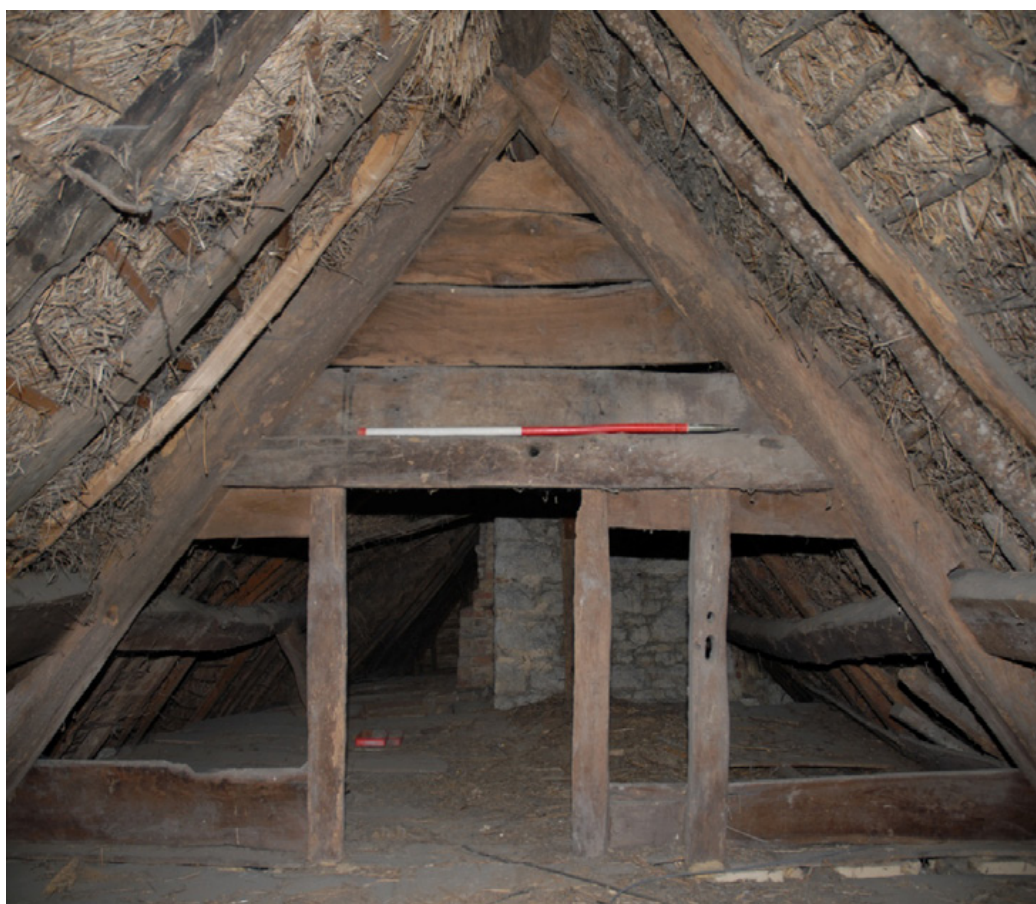
The modified queen post truss, looking east Fig 66
