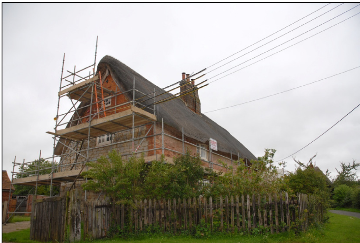
The south-western corner of the farmhouse, looking north-east Fig 9
