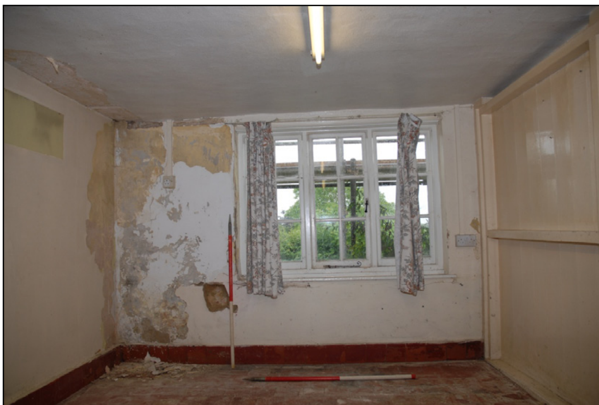
The south wall of the Dining Room Fig 23
