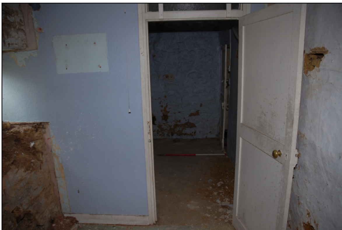
The central partition looking through into the Dressing Room Fig 41
