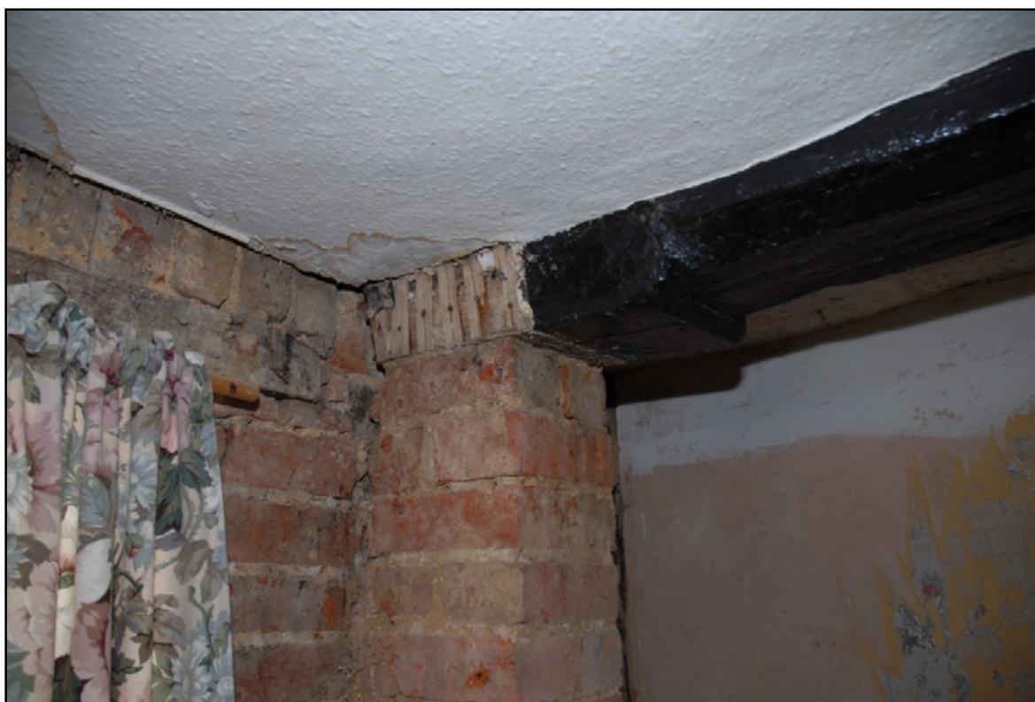
Beam resting on the brick plinth abutting the south wall Fig 34
