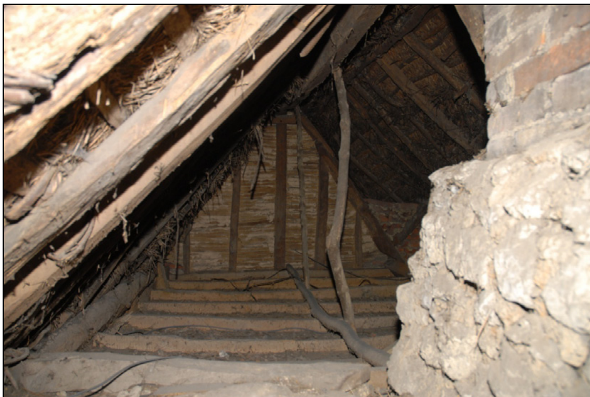
The eastern roof partition above Bedroom 1, looking east Fig 68
