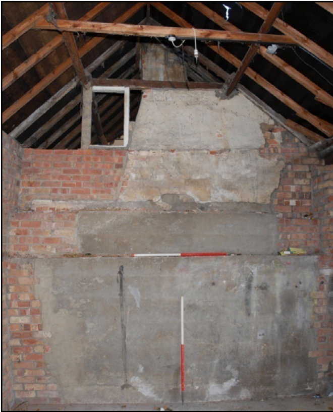
The north elevation of the chimney in the Garage Fig 18
