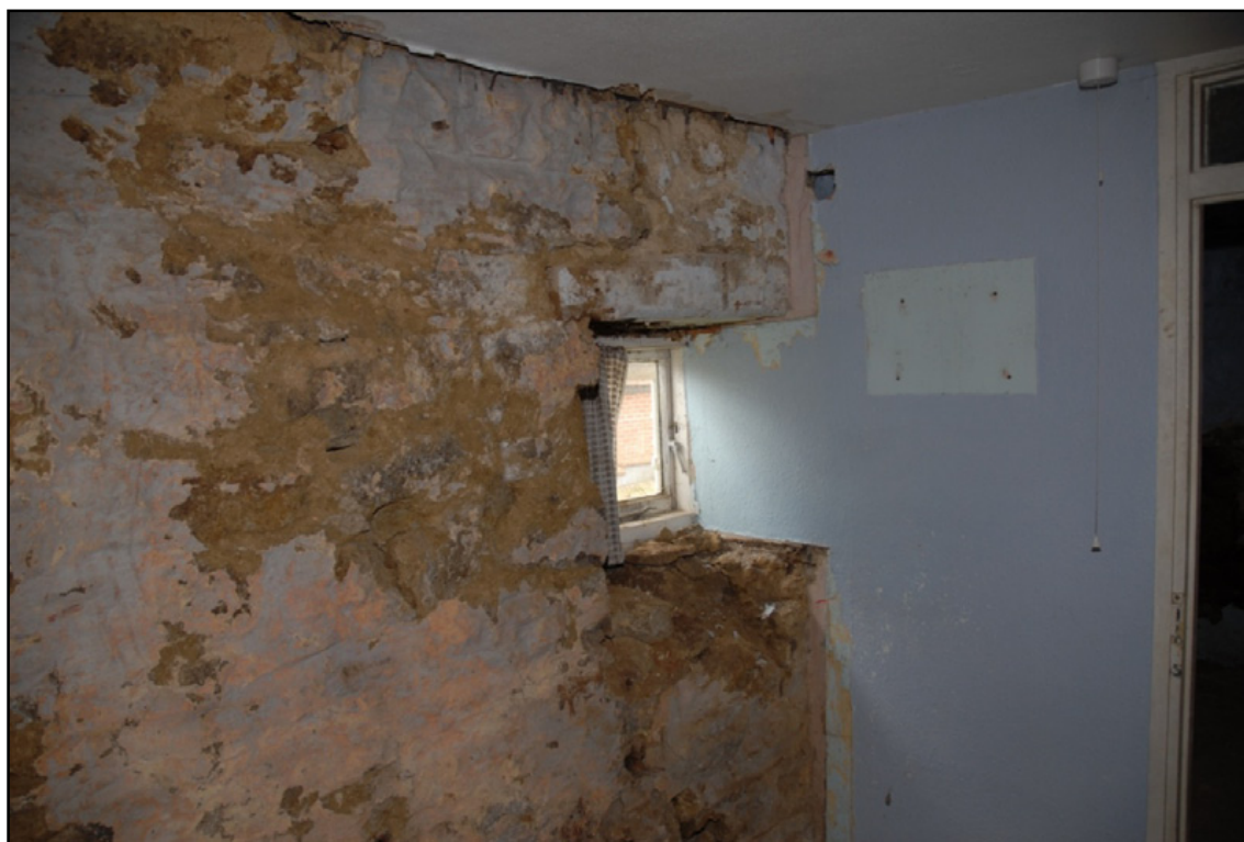
The window in the west wall of the Bathroom Fig 42
