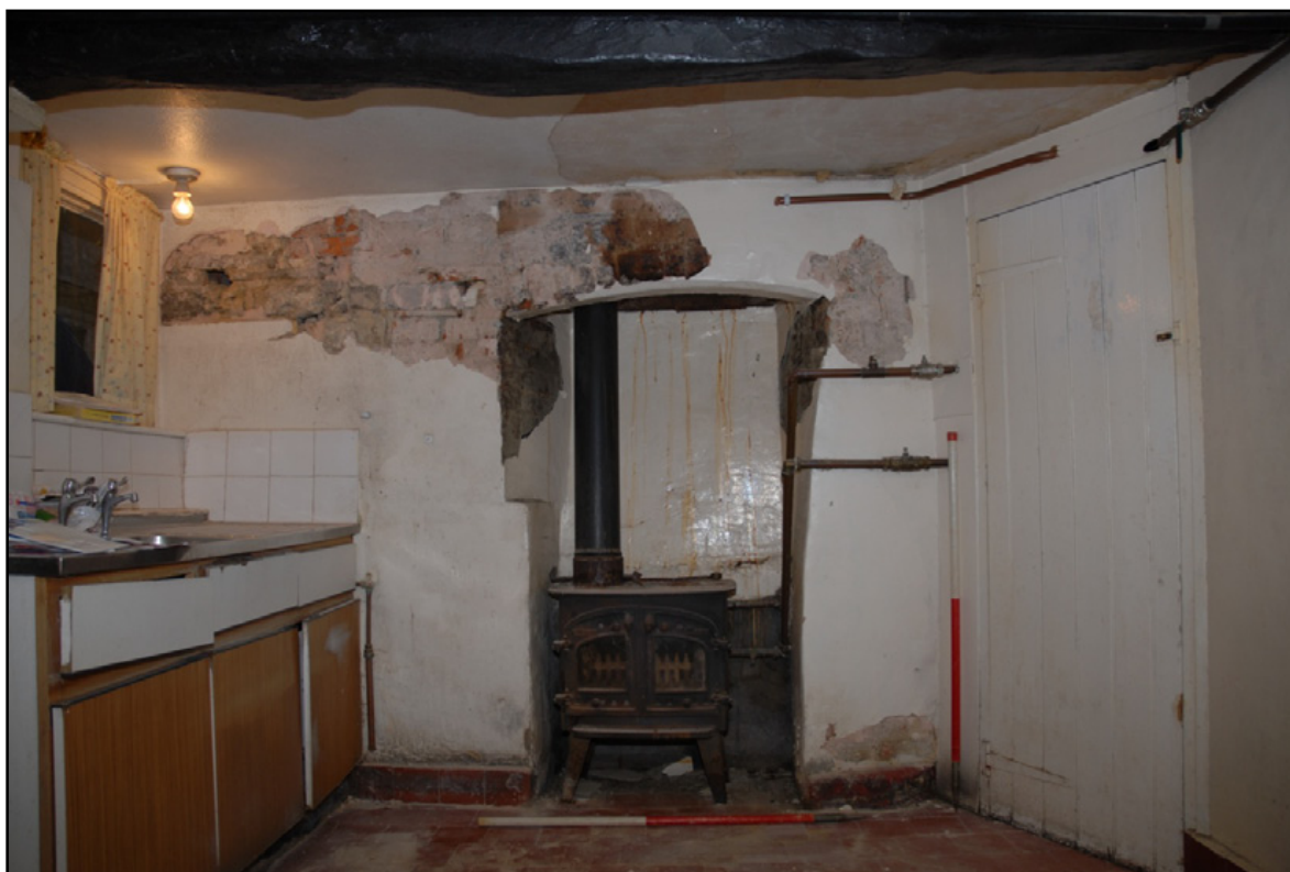
The north wall of the Kitchen showing the fireplace Fig 22
