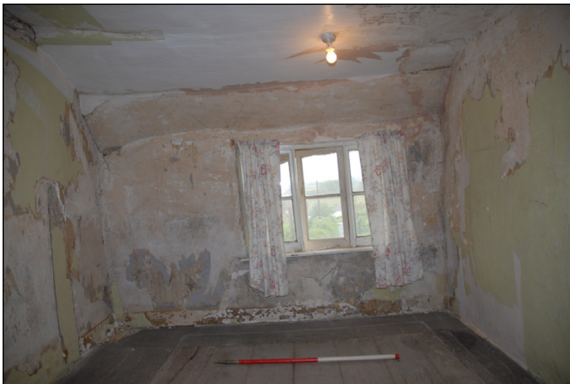
Bedroom 3, looking south Fig 59
