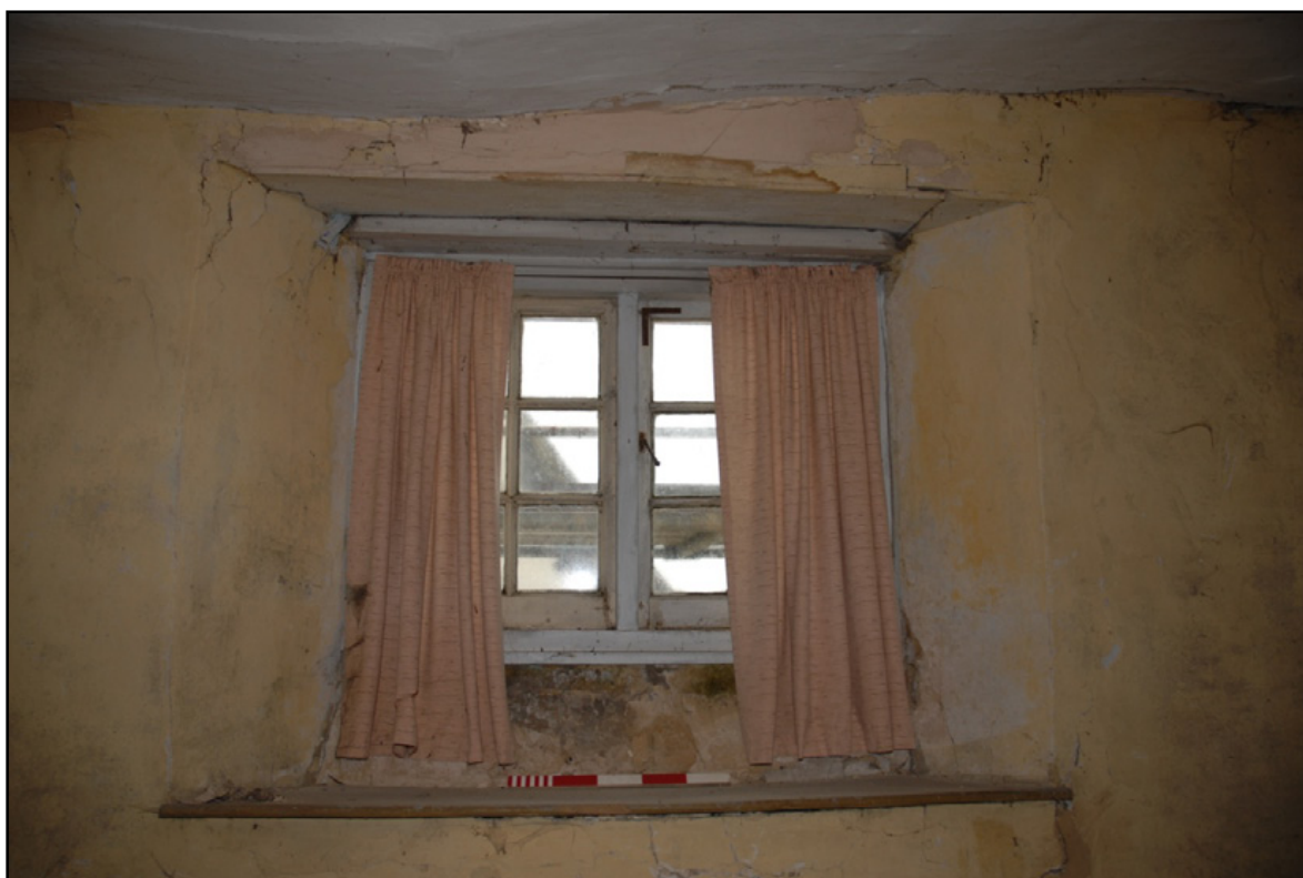
The window in the west wall of Bedroom 4 Fig 63
