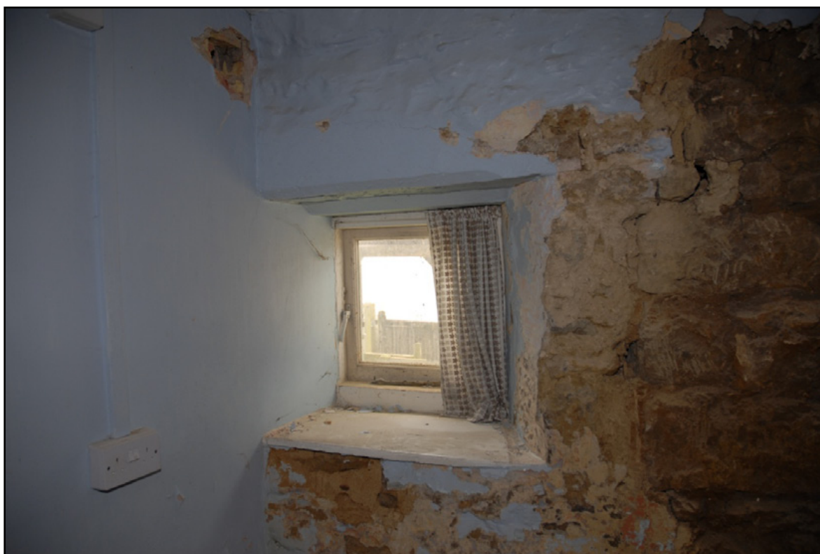
The window in the Dressing Room Fig 39
