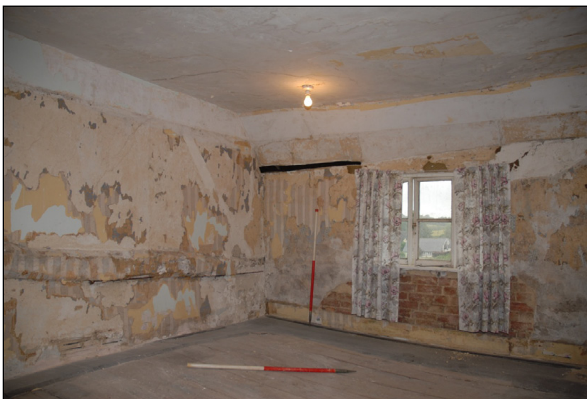
Bedroom 2, looking south-east showing the timber beam in the east wall Fig 54
