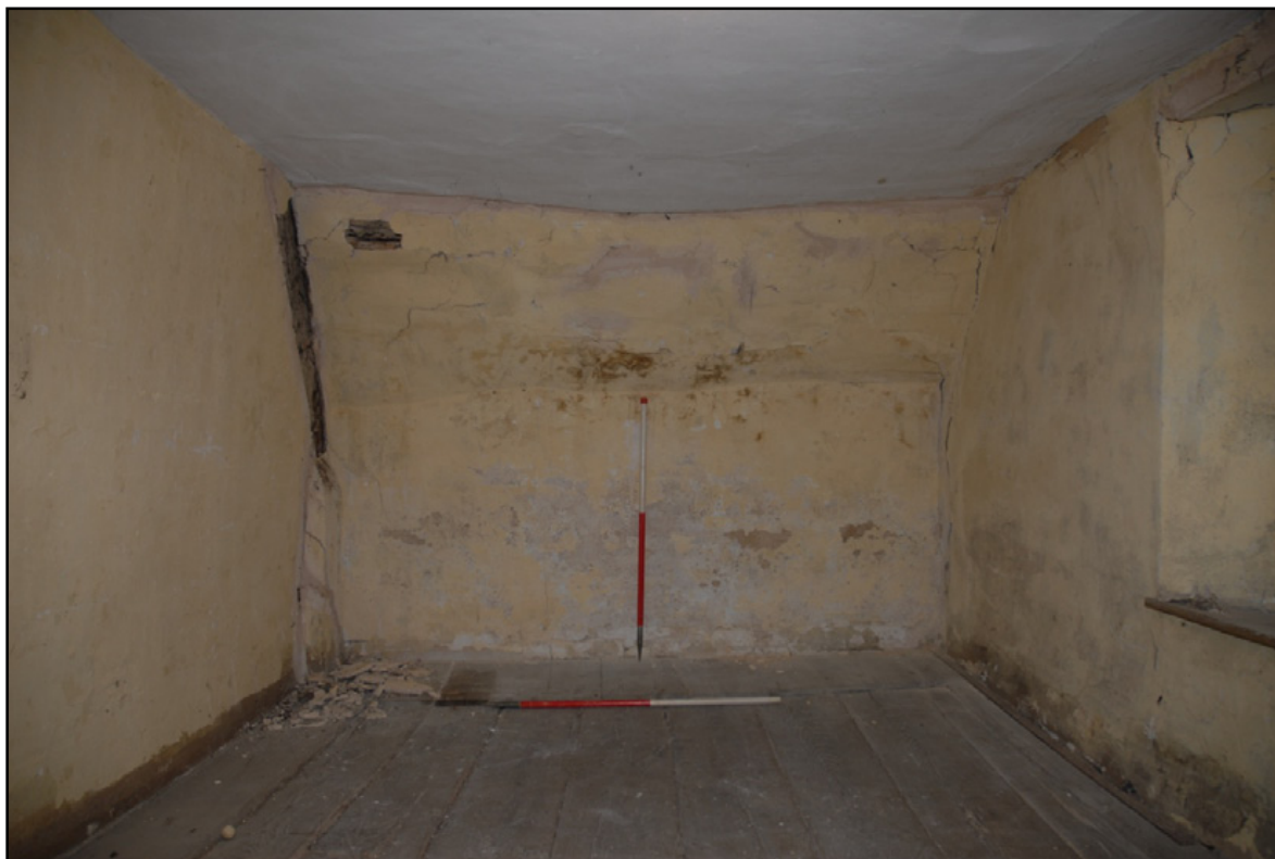
Bedroom 4, looking south Fig 62
