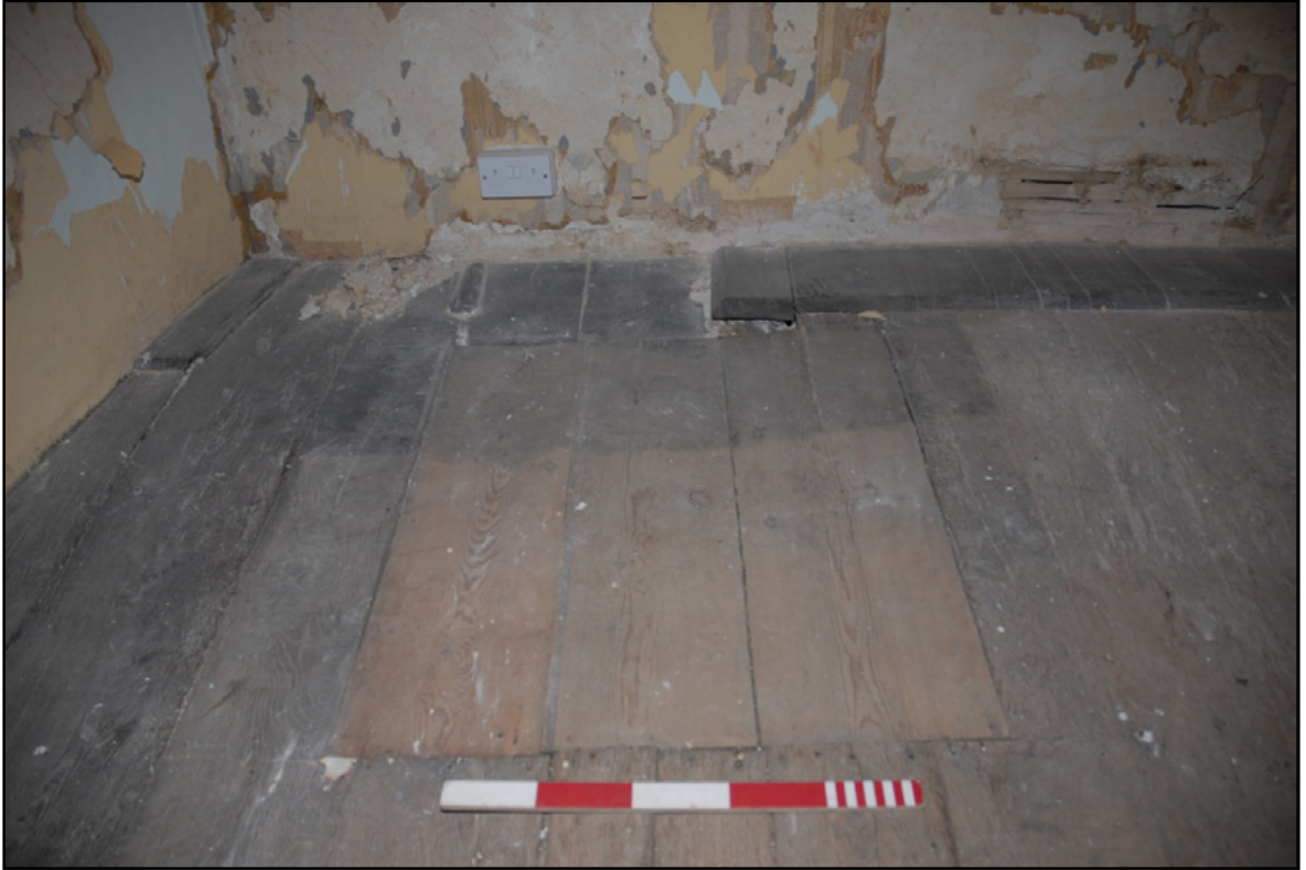
The trapdoor in Bedroom 2 showing the chamfered border Fig 57
