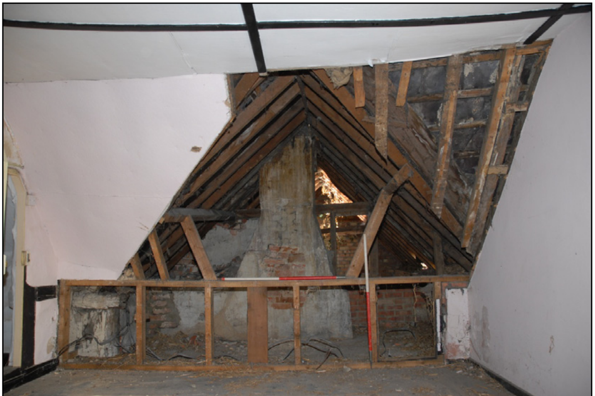
The south face of the chimney as seen from Bedroom 1 Fig 20
