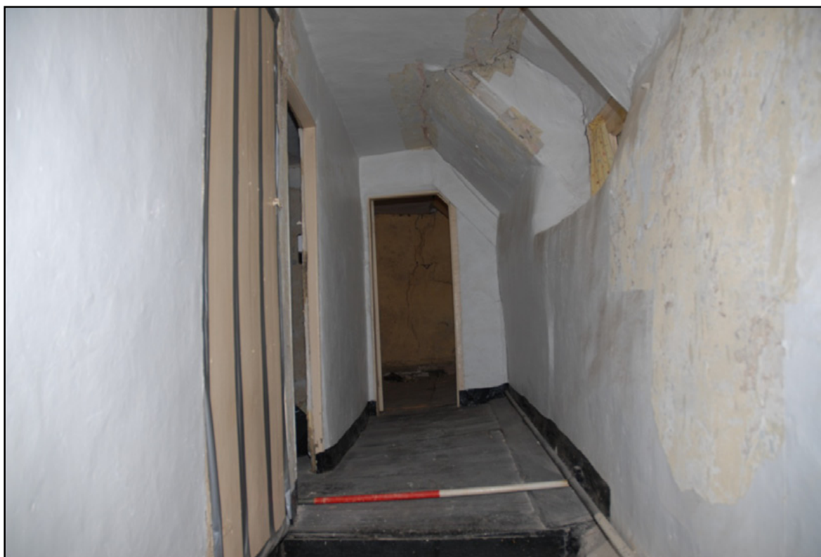
The first floor corridor, looking west Fig 49
