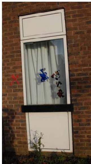
Block 4, Children's ward window Fig 24
