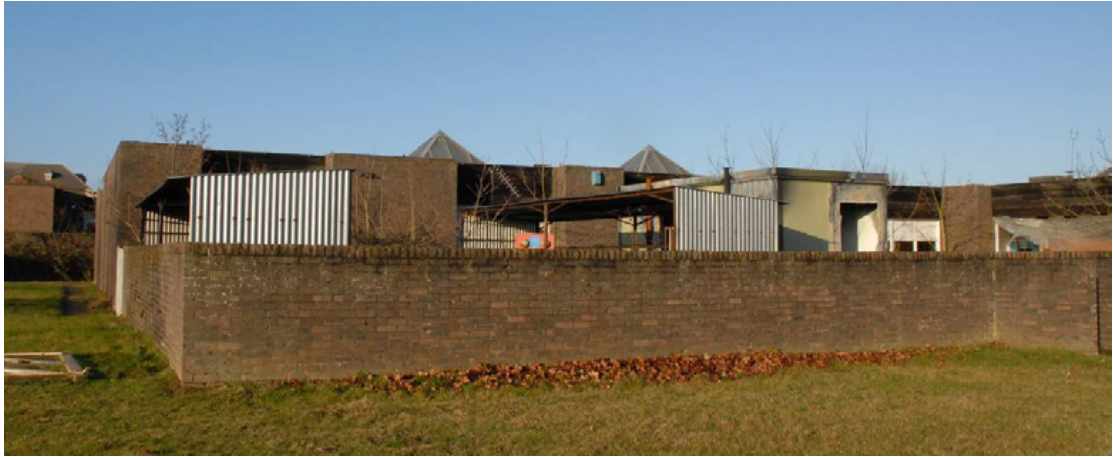
Block 4, smoking shelter, looking north-west Fig 25
