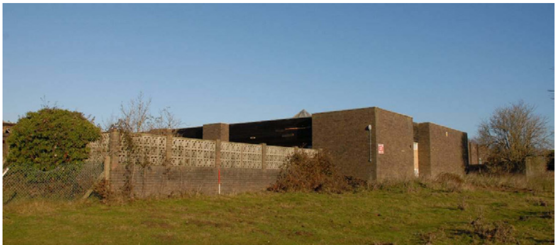
Block 1, looking north Fig 10
