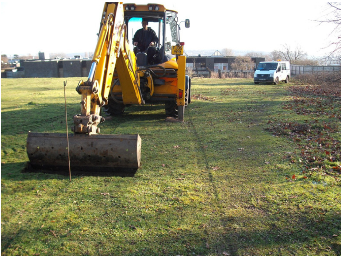
General view of the excavation of the trial trenches Fig 29
