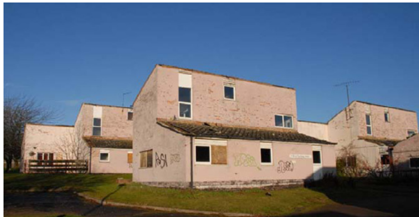
The staff accommodation Fig 26
