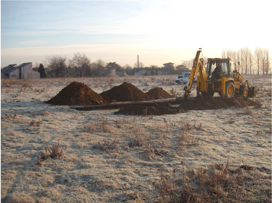
Trench 4 during excavation, looking east Fig 33
