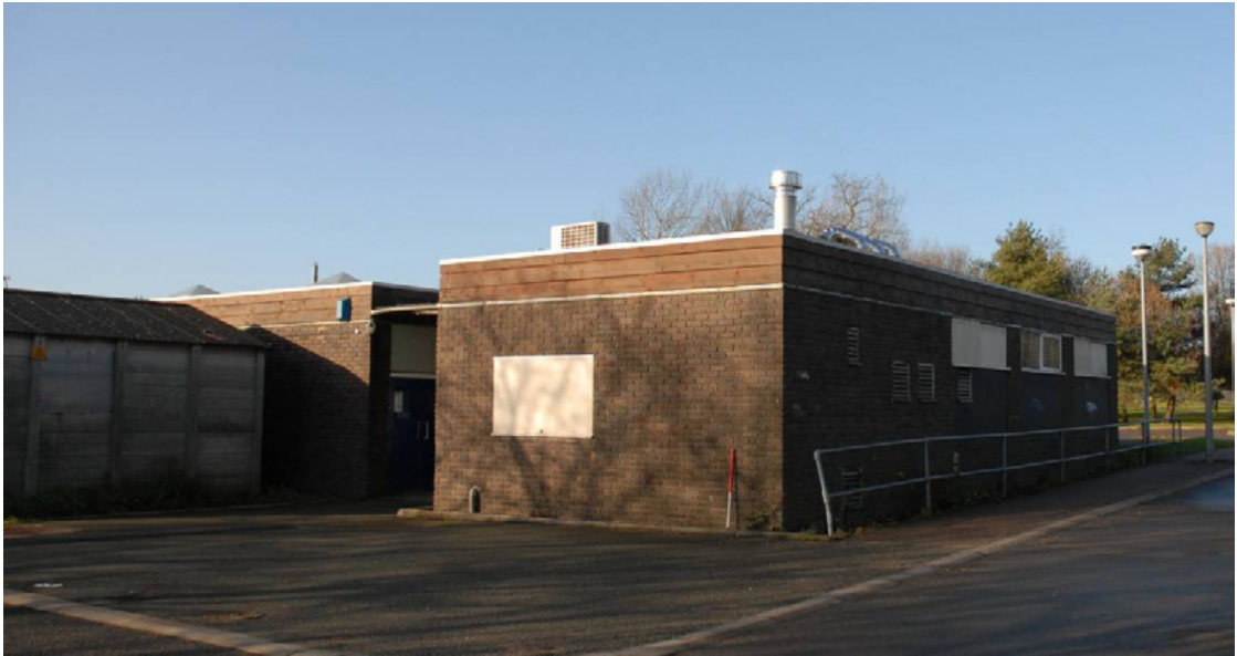
The estates office, looking north-west Fig 15
