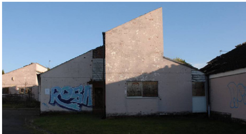
The staff accommodation showing the triangular lines of construction Fig 27
