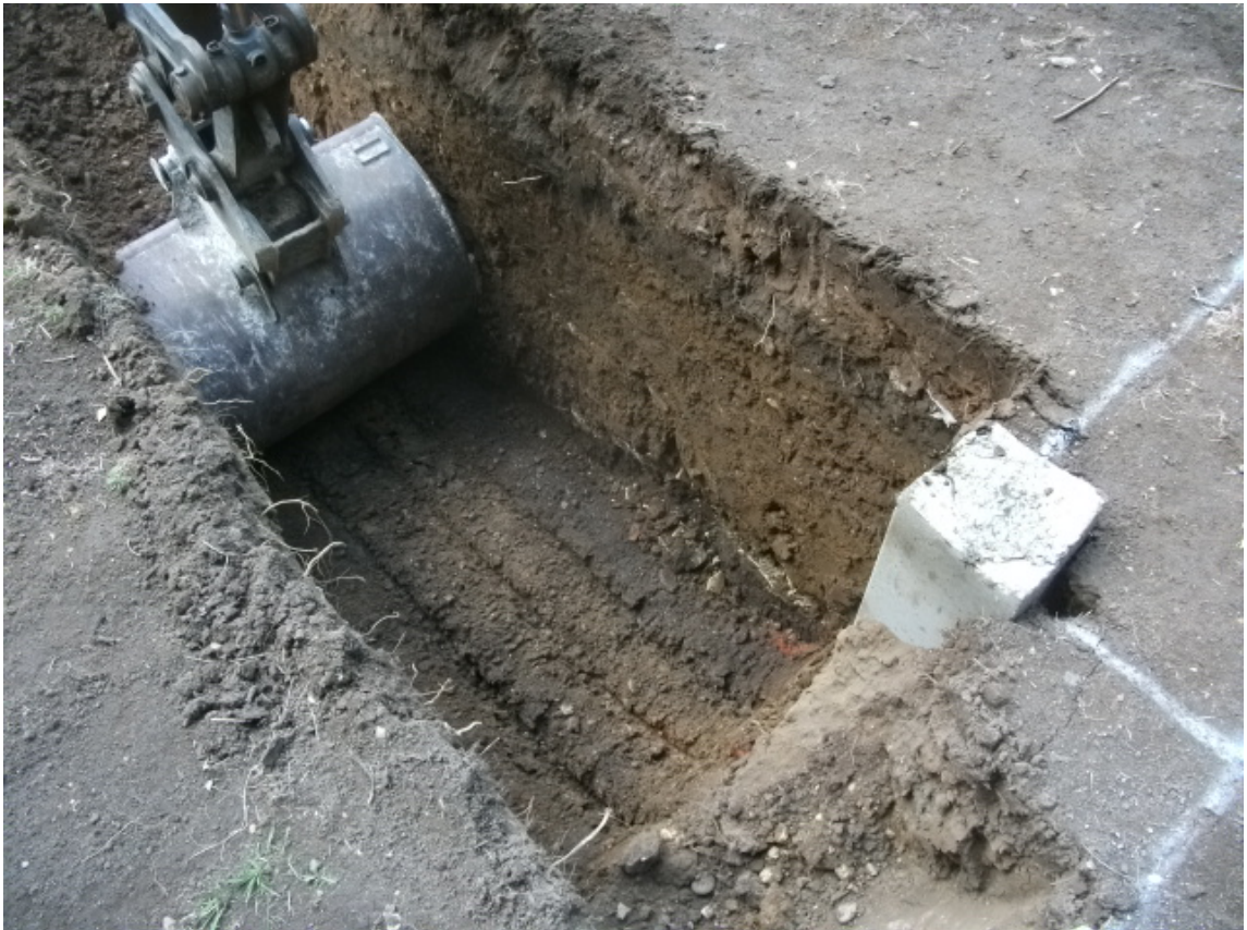
The concrete piles in-situ during the excavation of the foundations Fig 4
