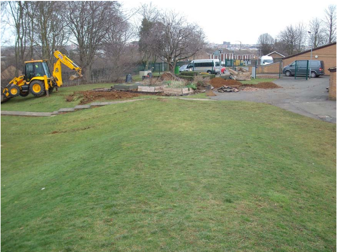
General view of the site during the evaluation, looking north-east Fig 3
