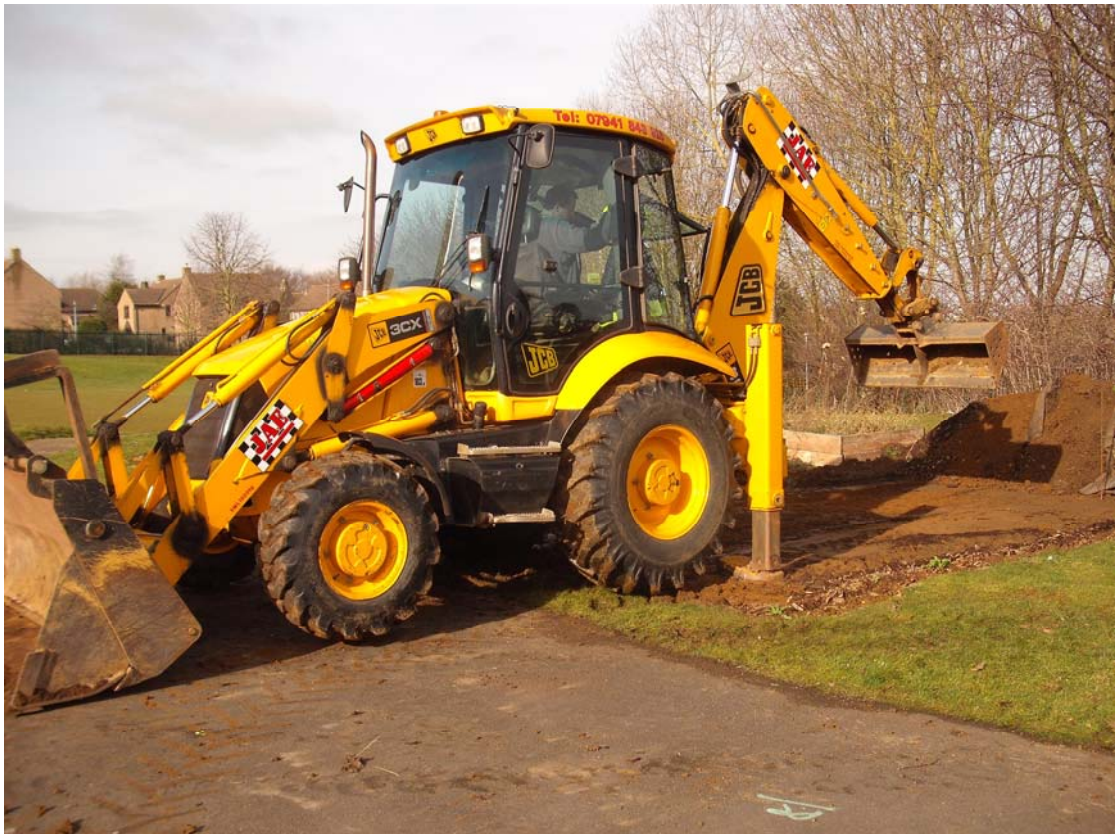
General view of the excavation of the trial trenches Fig 4
