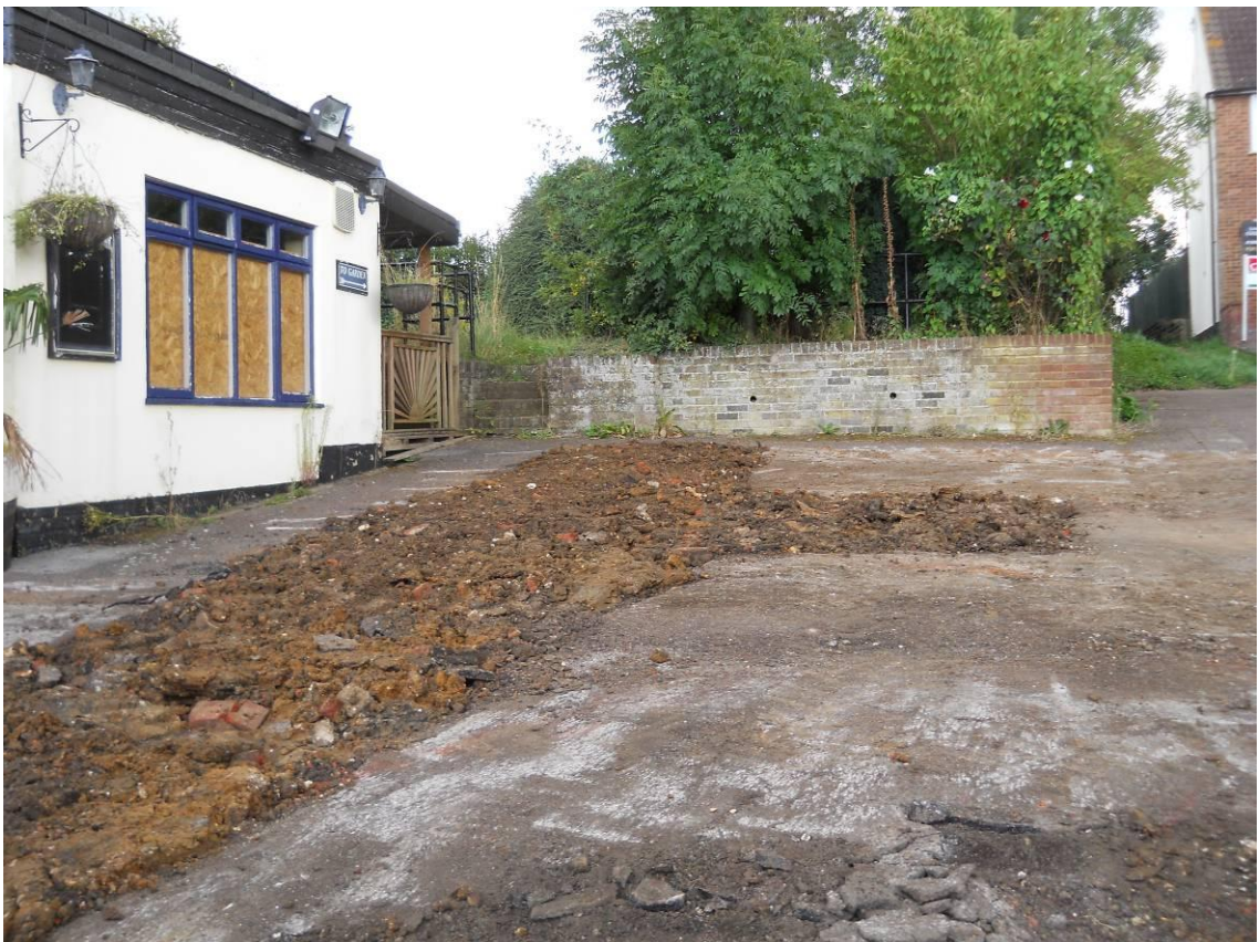
Backfilled trenches, looking east Fig 7
