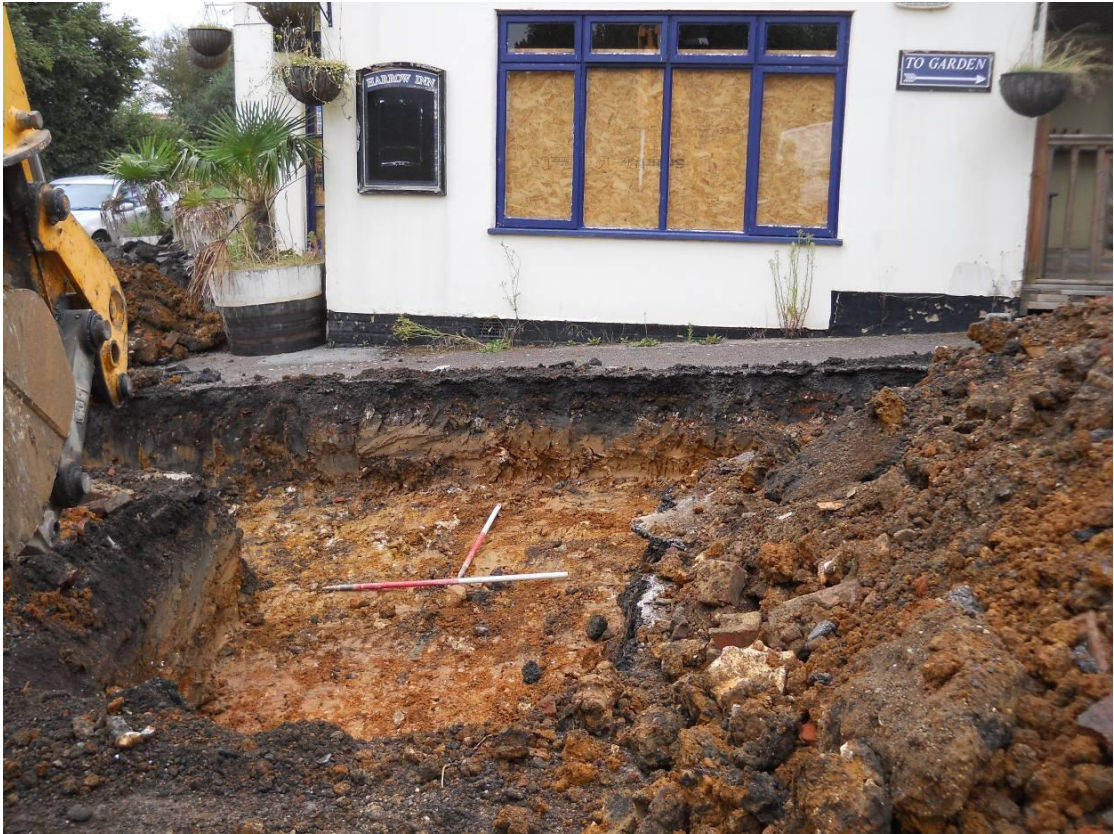
Trench 2 and slope down to Woodside Road, looking north-east Fig 6
