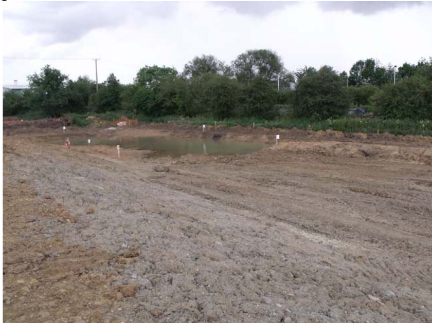
Balancing pond and raised ground in Area A, looking south-west Fig 6
