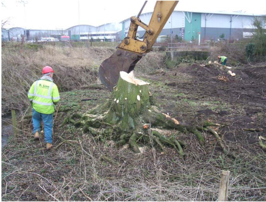
Removal of tree stumps in Area A, looking south-west Fig 5
