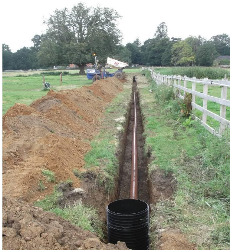
Waste water drainage trench under excavation, looking north Fig 4
