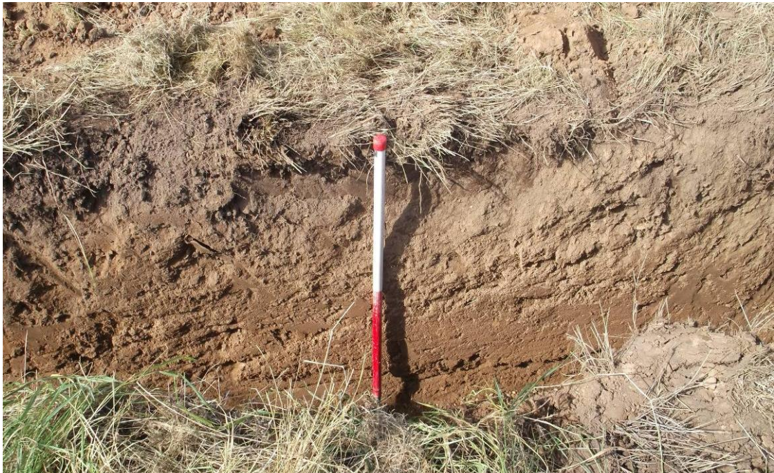
Typical trench section at the south end, looking west (scale 1.0m) Fig 5
