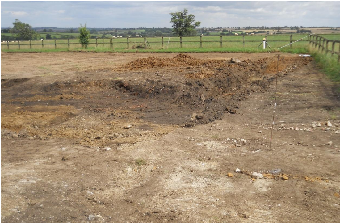
South side of ménage area during stripping, looking east Fig 5
