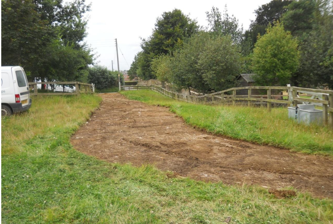
Topsoil removed from new access road, looking east Fig 3
