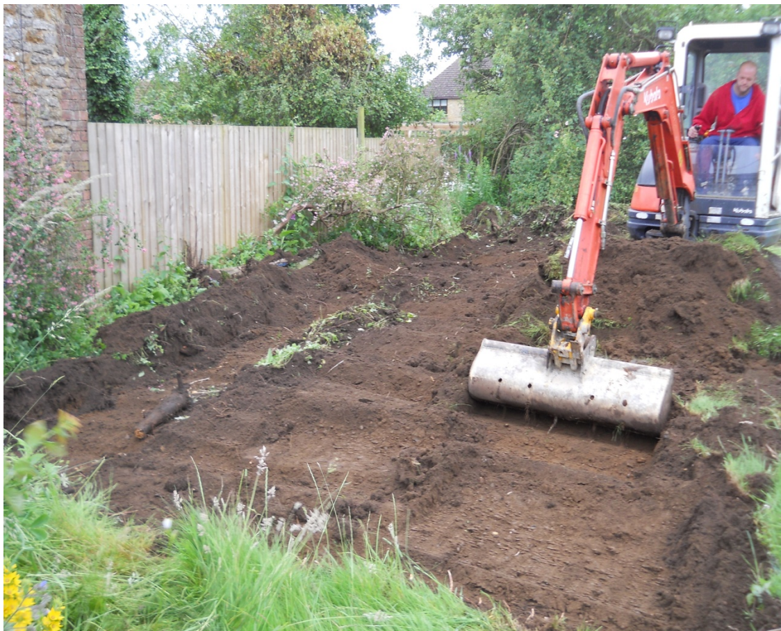
Stripping of topsoil, looking east
