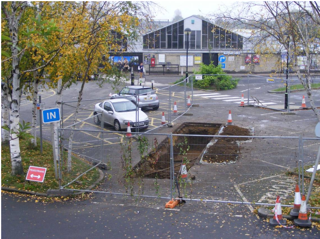
The location of the trench within the station concourse Fig 6
