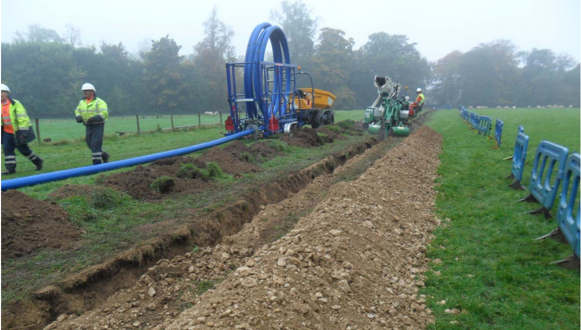
Pipe trench excavation, looking south-west Fig 4
