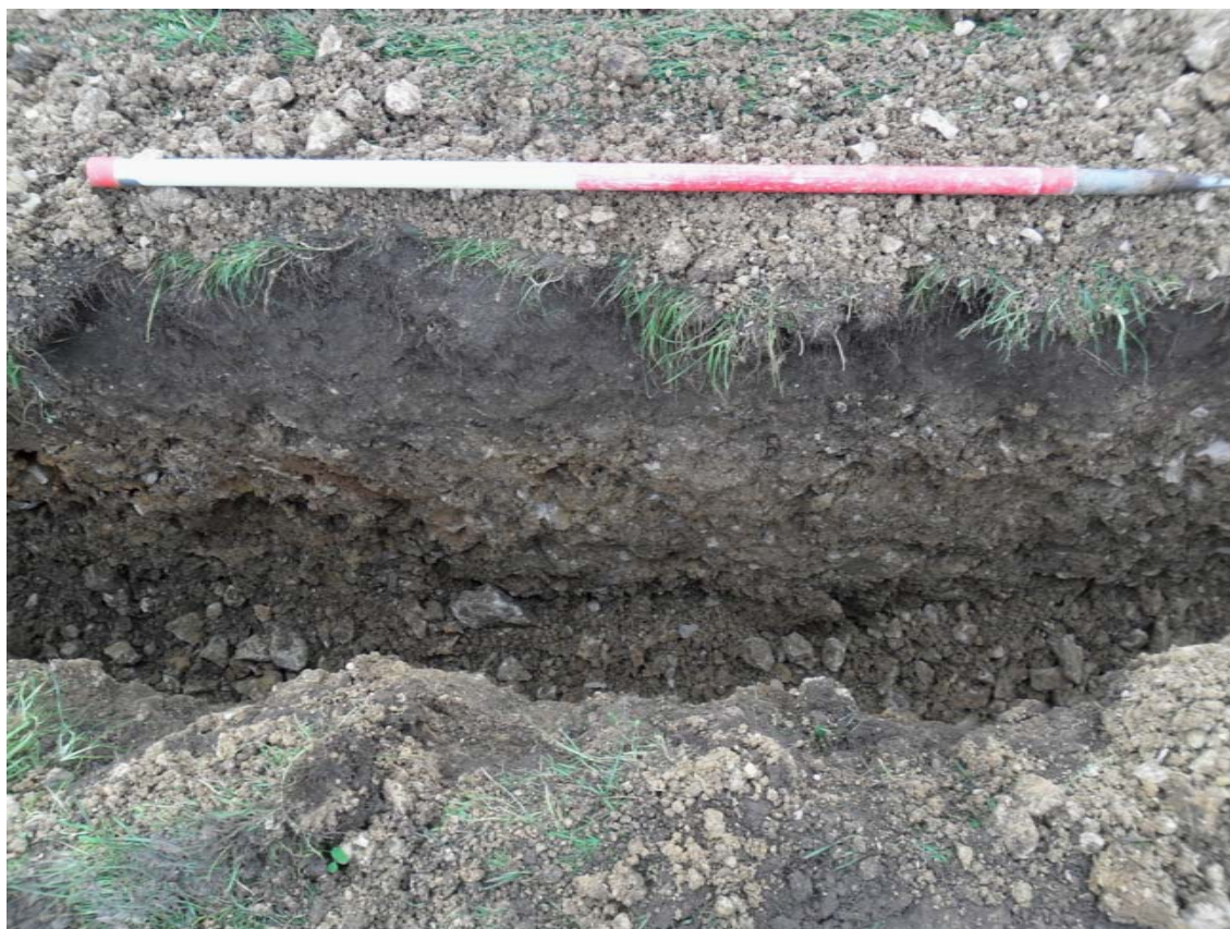
Section of the fully excavated pipe trench, looking north Fig 3
