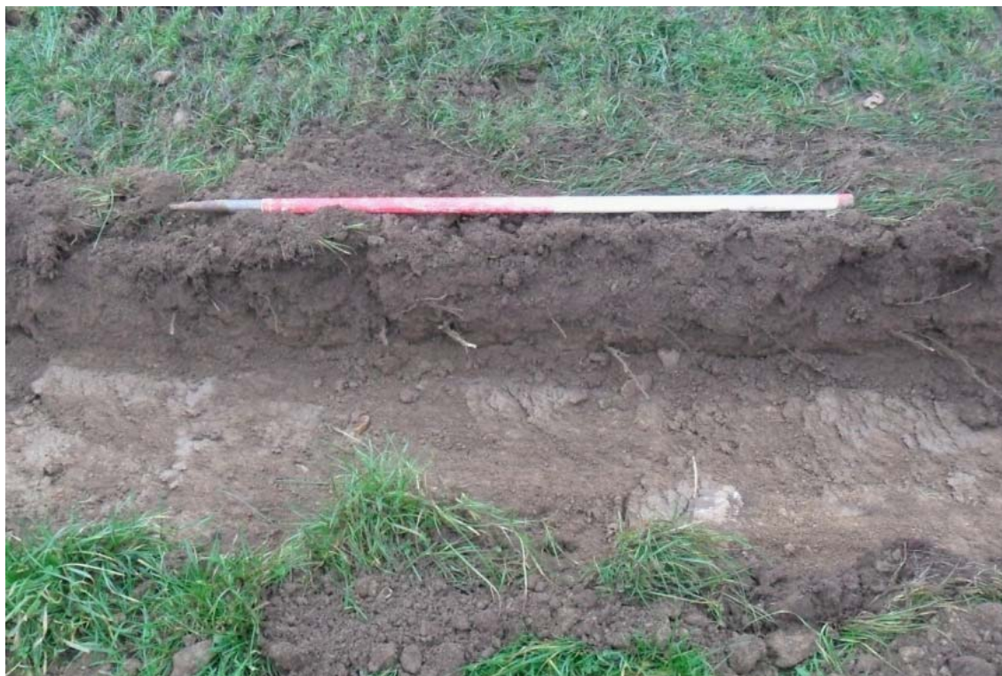
Topsoil strip along the pipe trench, looking north Fig 2
