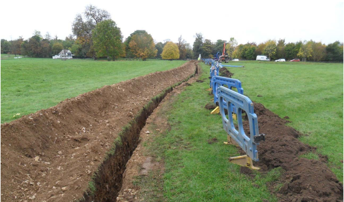
Route of the pipe trench, looking south-west Fig 5
