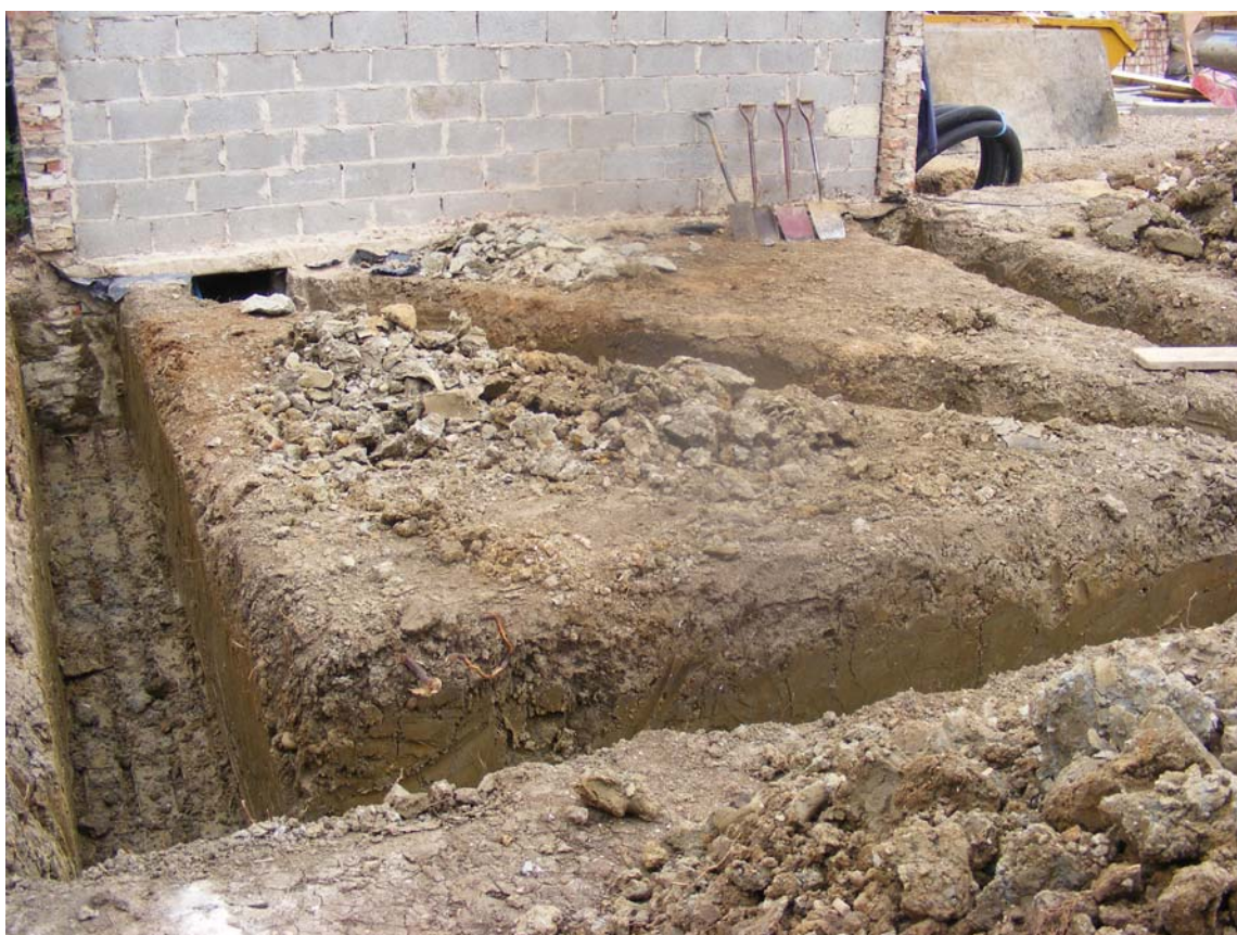
The new garage extension, looking north-east Fig 5
