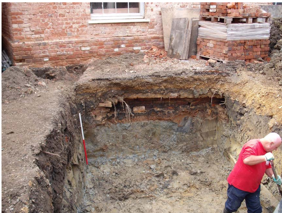
The gas tank pit Fig 9
