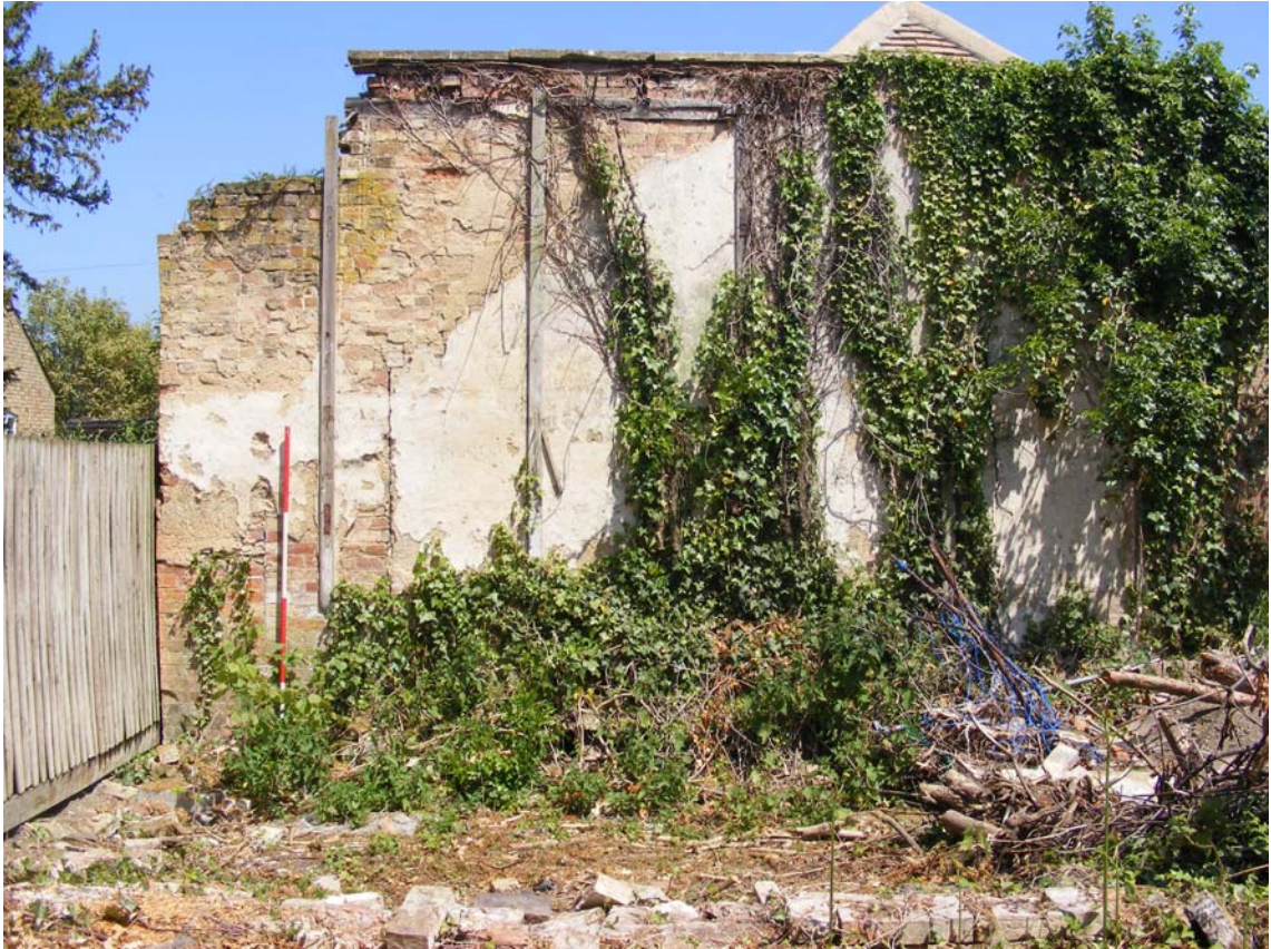
The Grade II Listed wall subject to the photographic survey Fig 11
