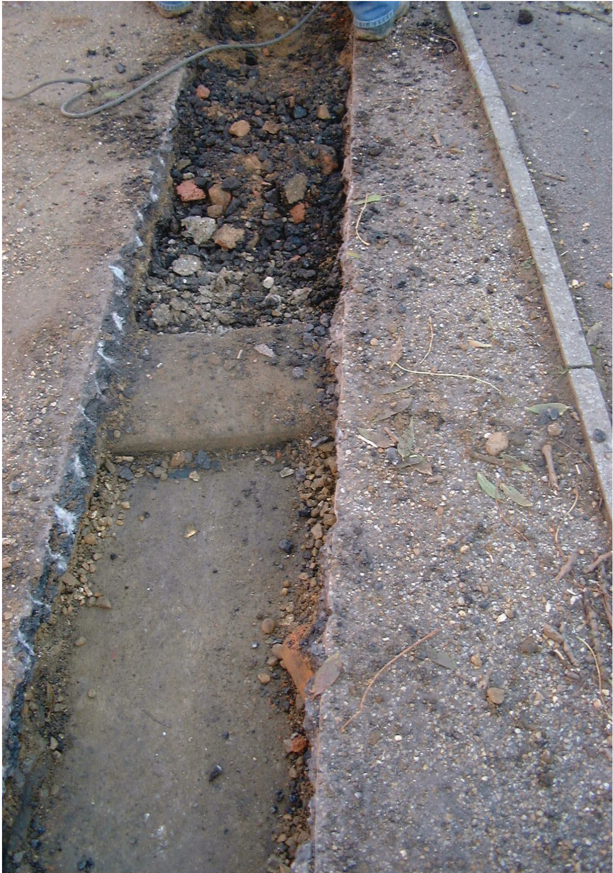
Plate 3: The north-south foundation trench, viewed towards the north
