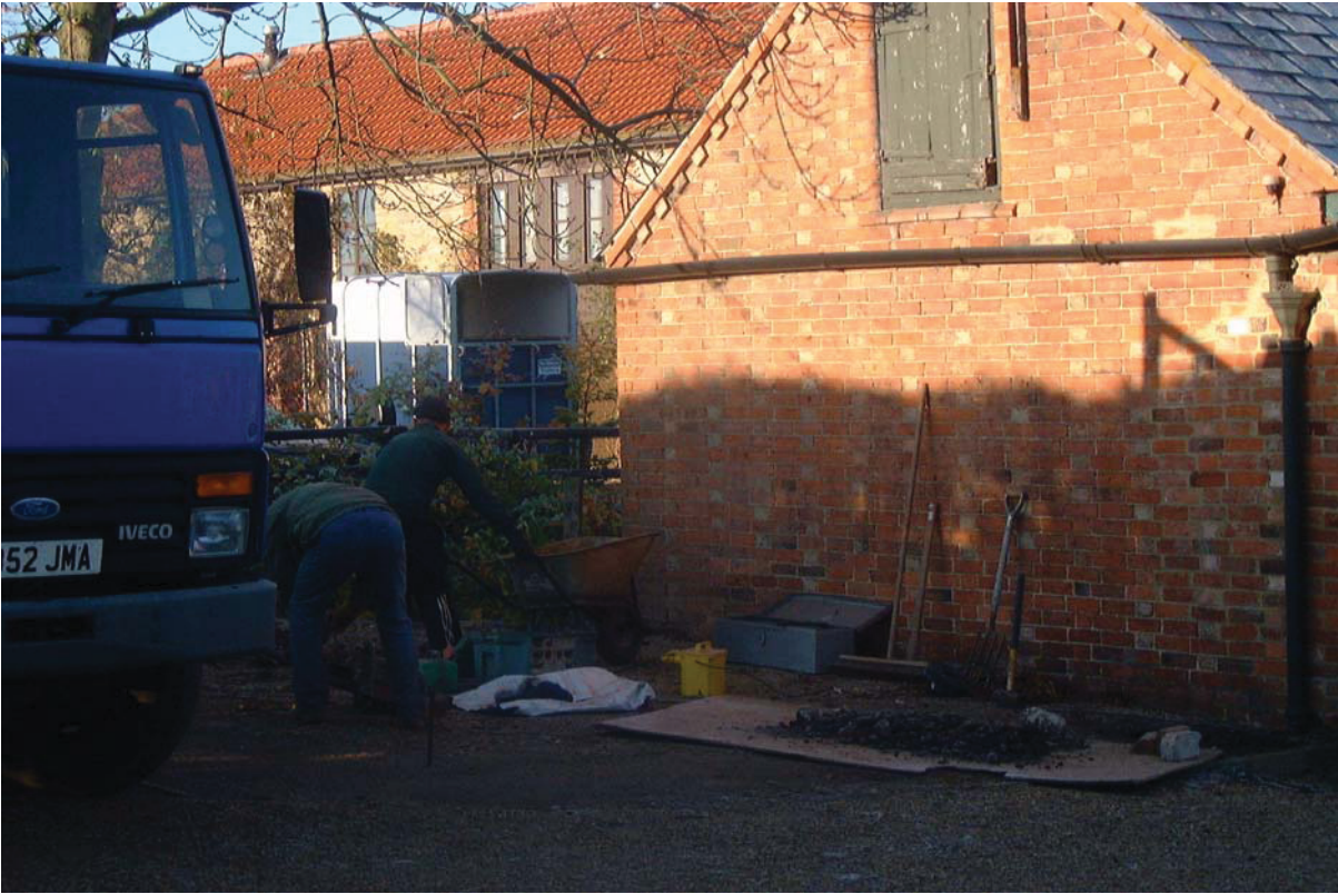
Plate 2: General view of the groundworks area
